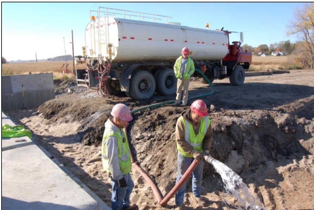
Figure 16. Water is applied to consolidate the fully-contained flooded backfill.
