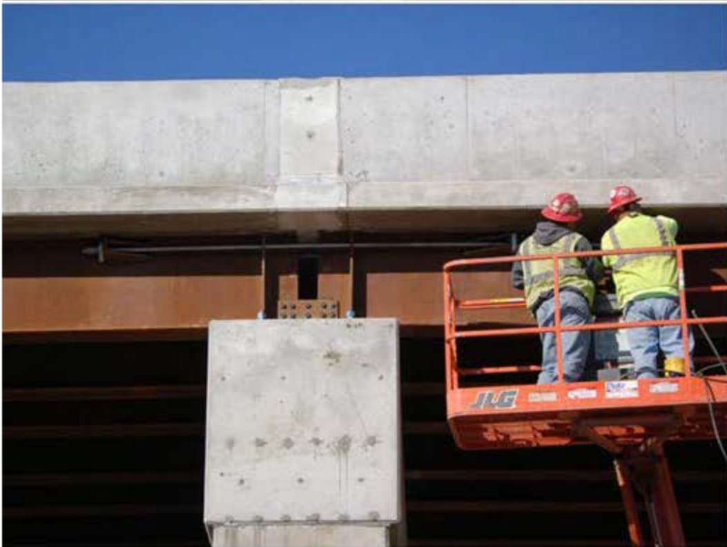
Figure 21. Post-tension retrofit installation.
