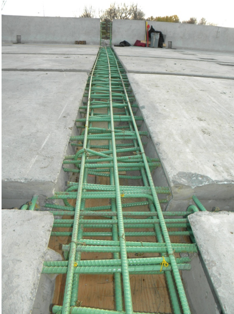
Figure 18. Pier joint reinforcement.
