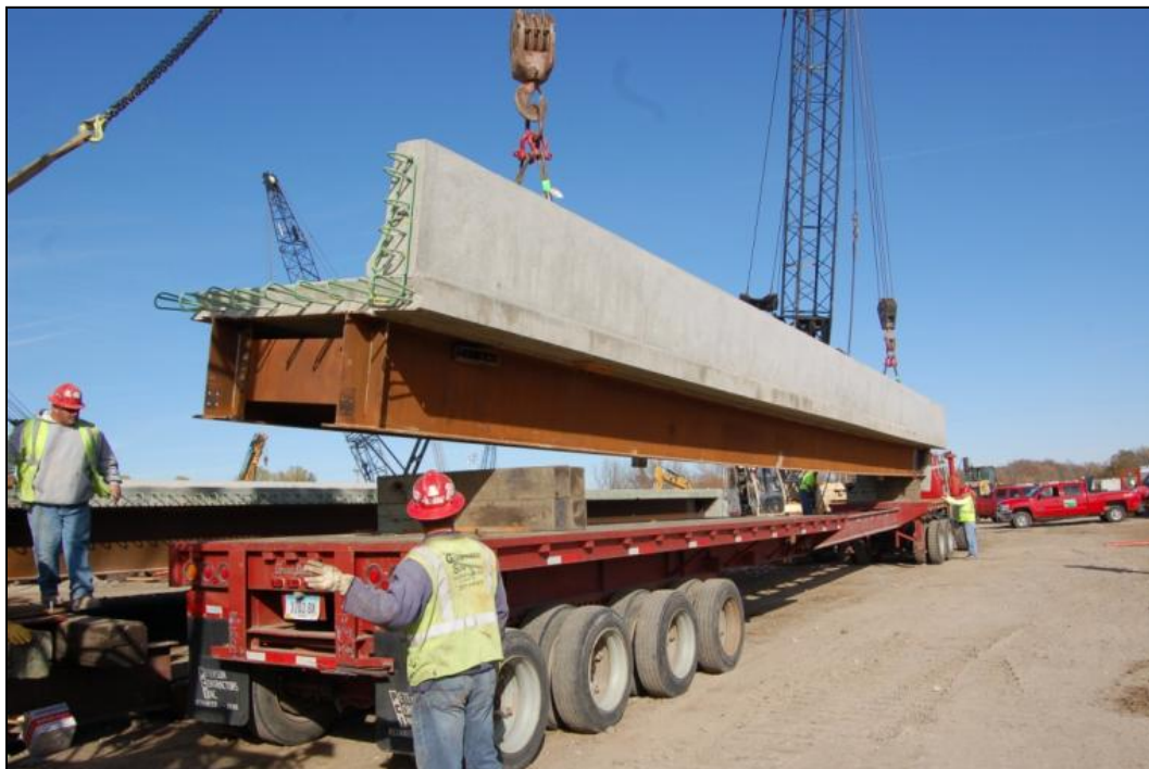
Figure 8. Lifting an exterior module into place.
