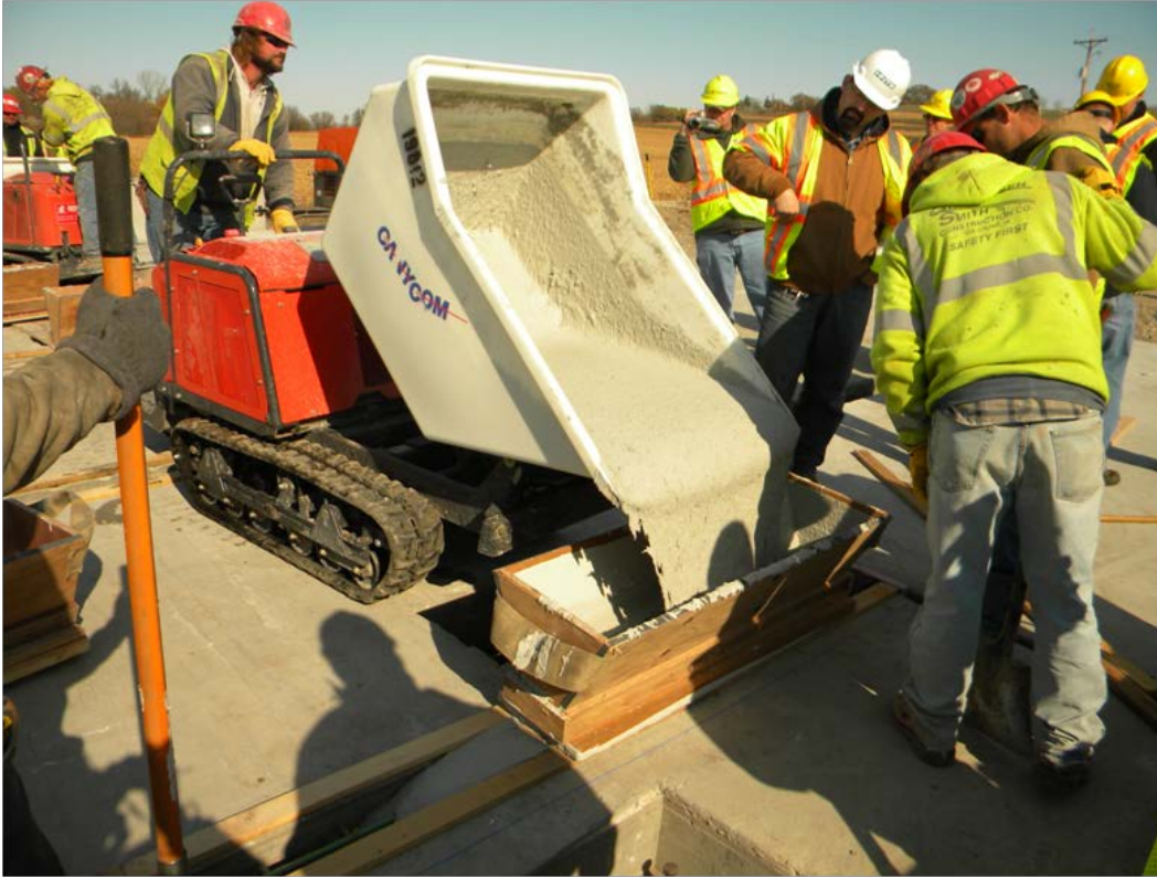
Figure 19. Workers place UHPC in a longitudinal joint.
