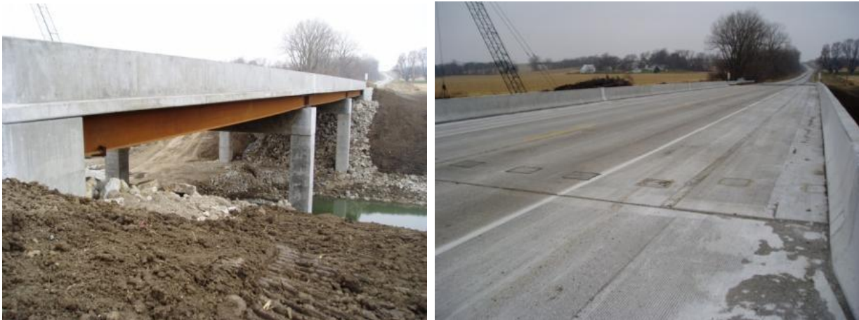
Figure 3. Newly reconstructed bridge.
