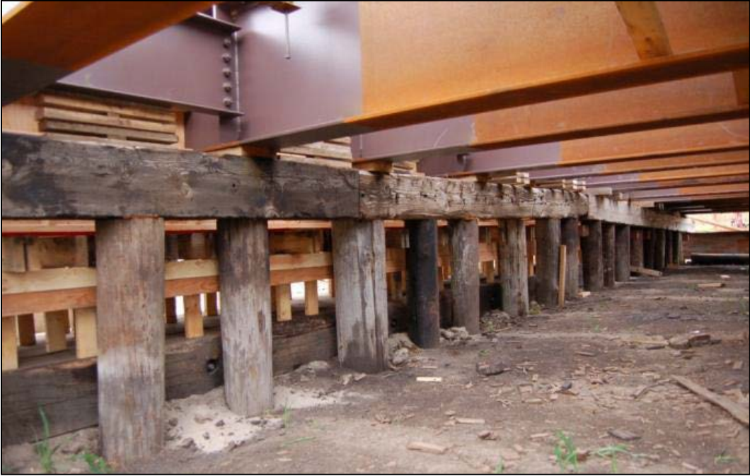
Figure 4. Temporary supports used for the bridge modules during fabrication.
