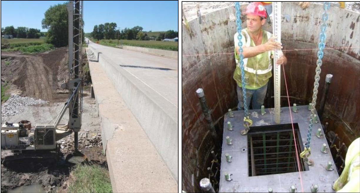
Figure 10. Drilled shafts next to existing bridge (left) and workers positioning rebar.
