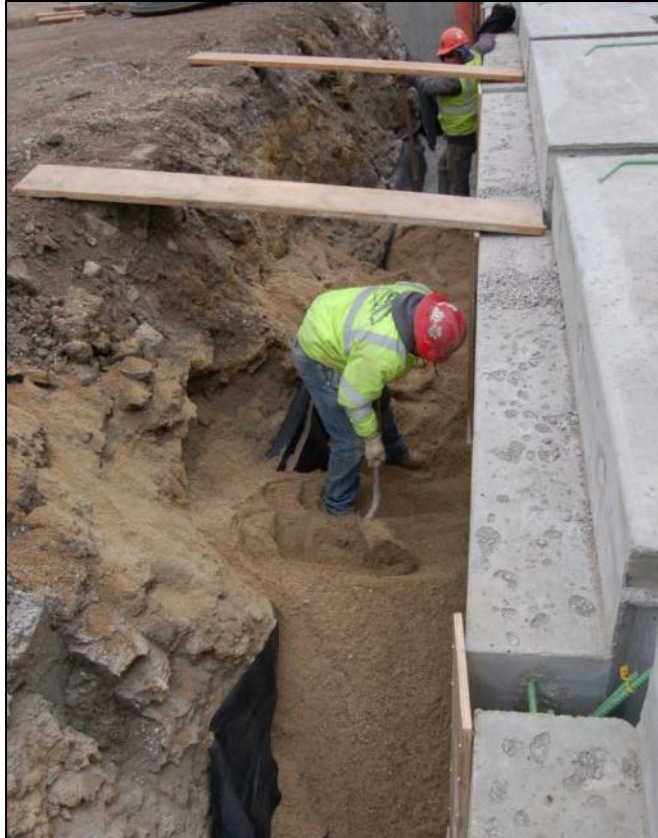
Figure 15. Workers spread granular backfill behind an abutment.
