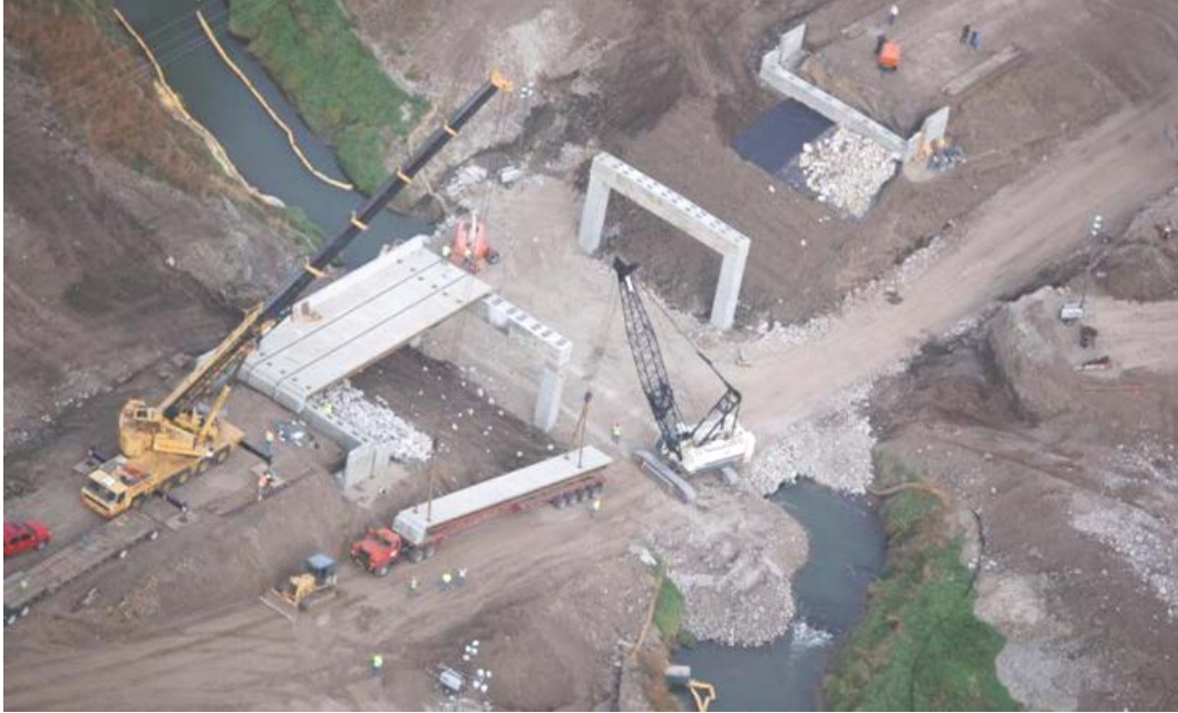
Figure 9. Aerial view showing placement of bridge modules.
