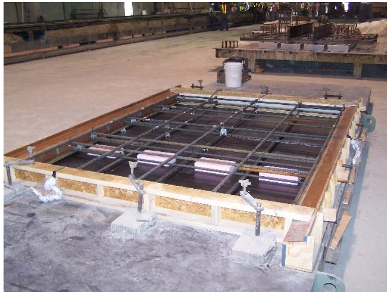
Figure 2 Final Form Setup
