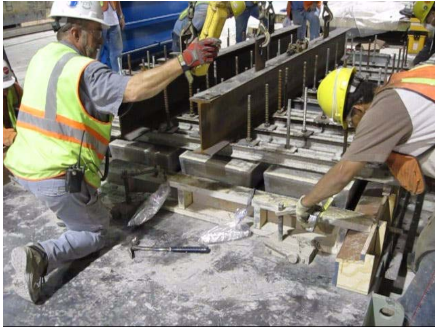
Figure 4 Placing the Voids
