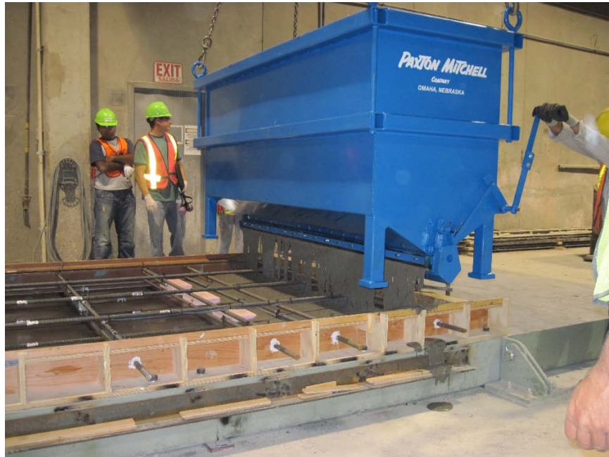
Figure 3 Casting
