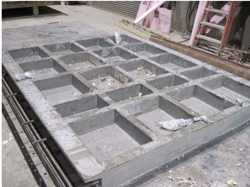
Figure 5 Formwork Removed
