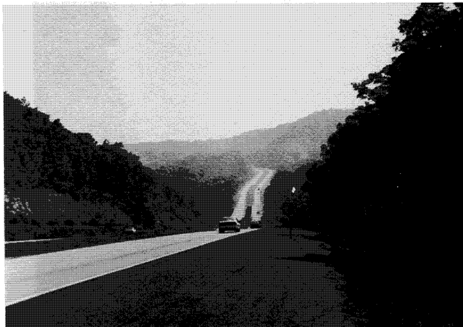
(13-B) Coal Road, U.S. 19 and State 16, near Fayetteville, WV
