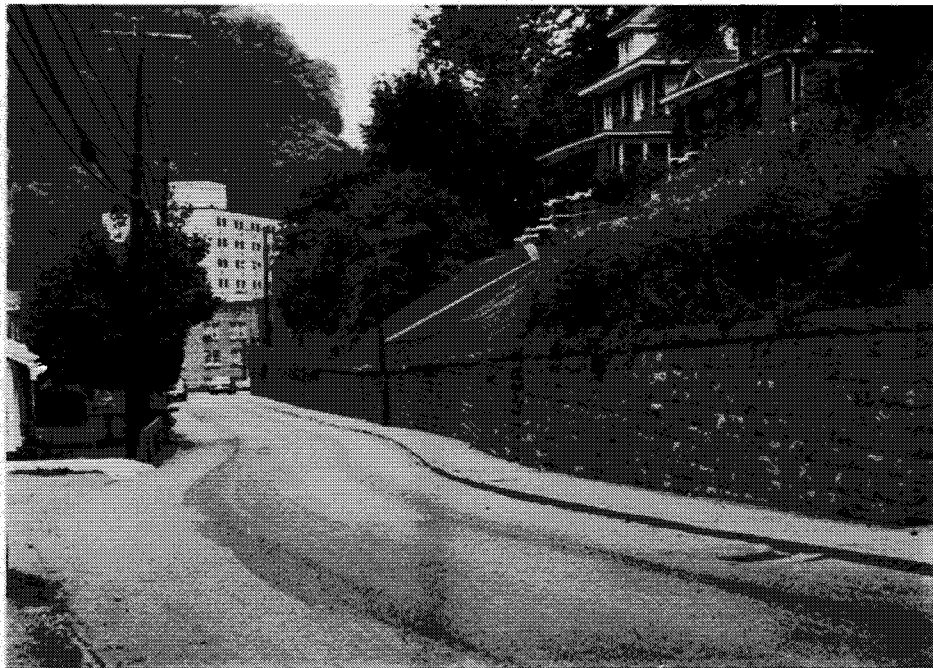
(34) Coal Road, Retaining Walls, U.S. 52 and State 16, Welch, WV
