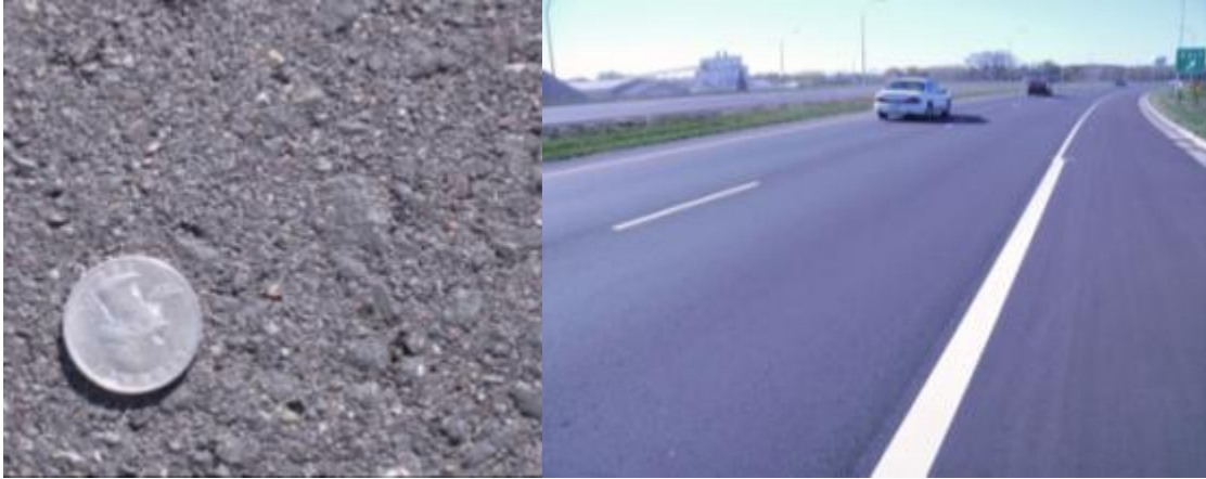
Figure 13. Newly constructed TH 36 HMA pavement.
