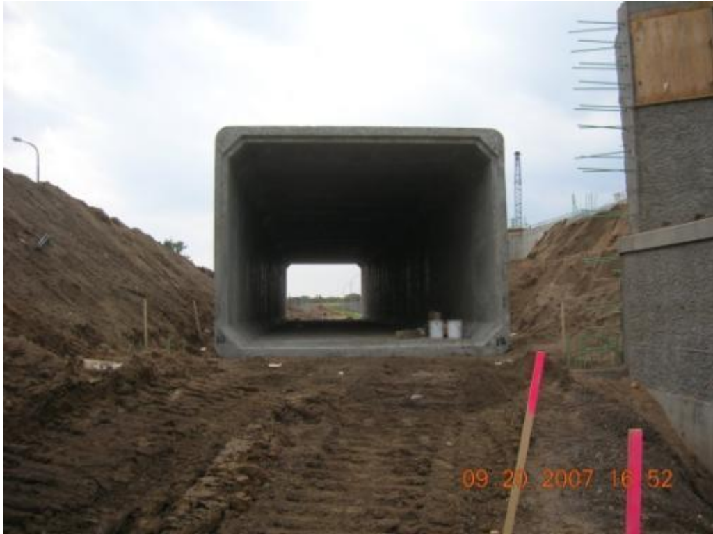
Figure 7. Gateway Trail box culvert tunnel at Margaret Street.
