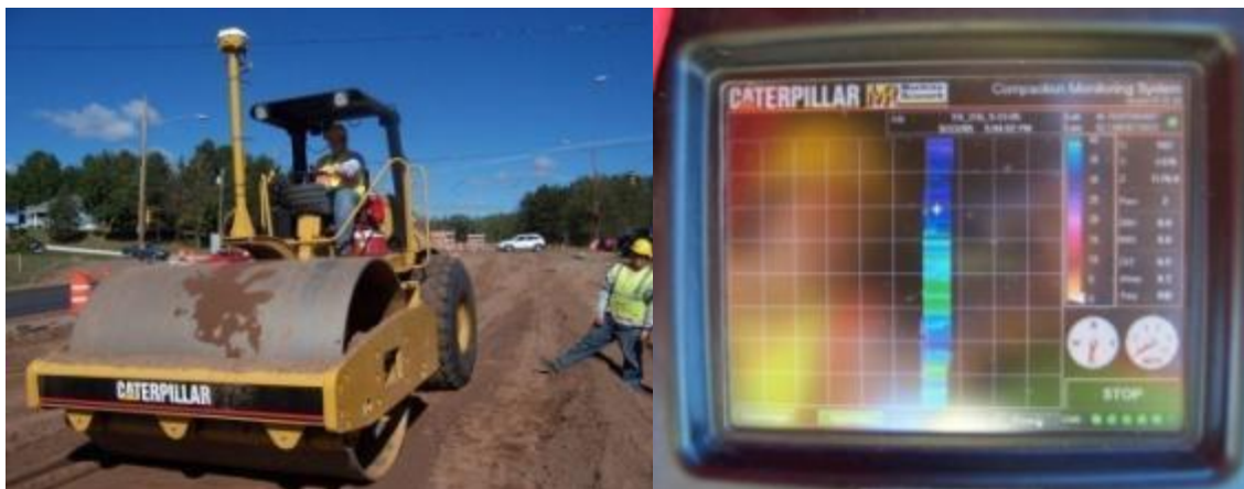
Figure 10. Intelligent compaction roller (left) equipped with compaction display (right). (Source: Mn/DOT)
