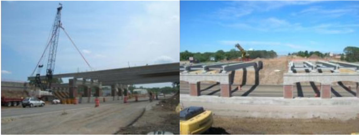
Figure 6. McKnight Road bridges under construction.
