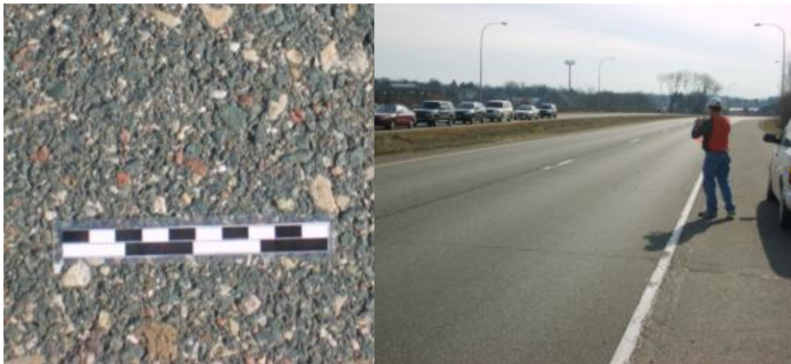
Figure 12. Existing TH 36 HMA pavement.
