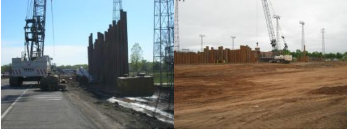
Figure 5. Shoring being placed along TH 36.
