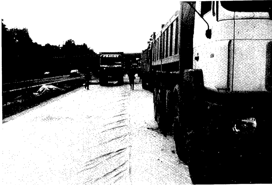
Figure 7: Concrete paving, Brandenburg. Separator fabric is placed between frost protection base layer and surface concrete. Fabric is nailed to the base.
