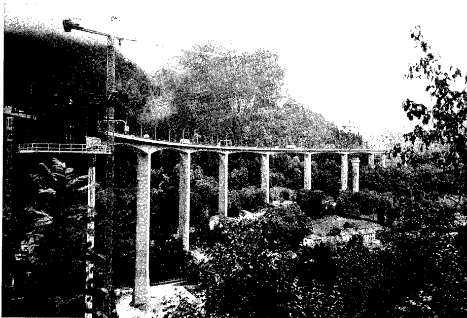
Figures 13 (a) and (b): High, twin structures (second structure under construction) near Nantua, France.
