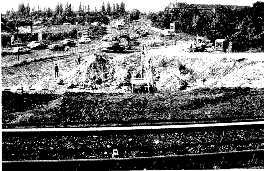
Figure 12: Interchange construction. Inner-ring autobahn, Berlin.
