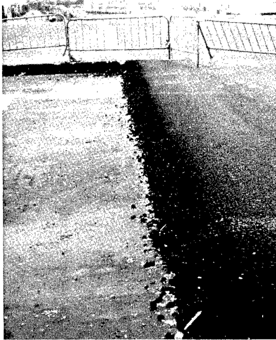
Figure 21: Asphalt paving underway, Madrid.
