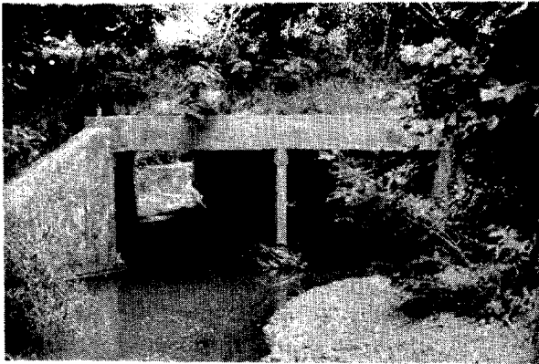
Figure VI-21--Double barrel box culvert.
