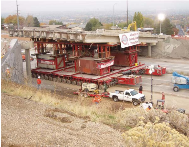
Figure 18. Lifting and removing the first span.
