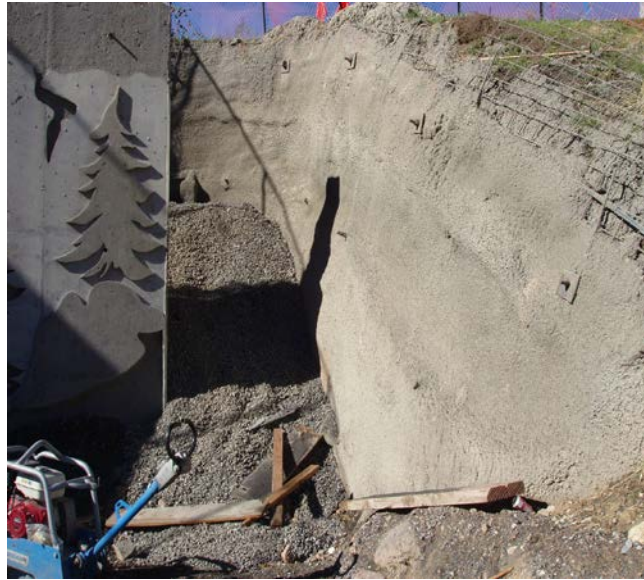
Figure 10. Soil nailing of the approach embankment.
