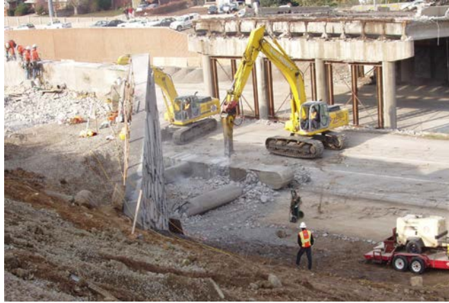
Figure 20. Demolition of the columns and bent caps.
