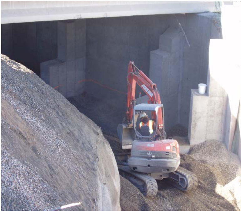
Figure 12. Placement of backfill material.
