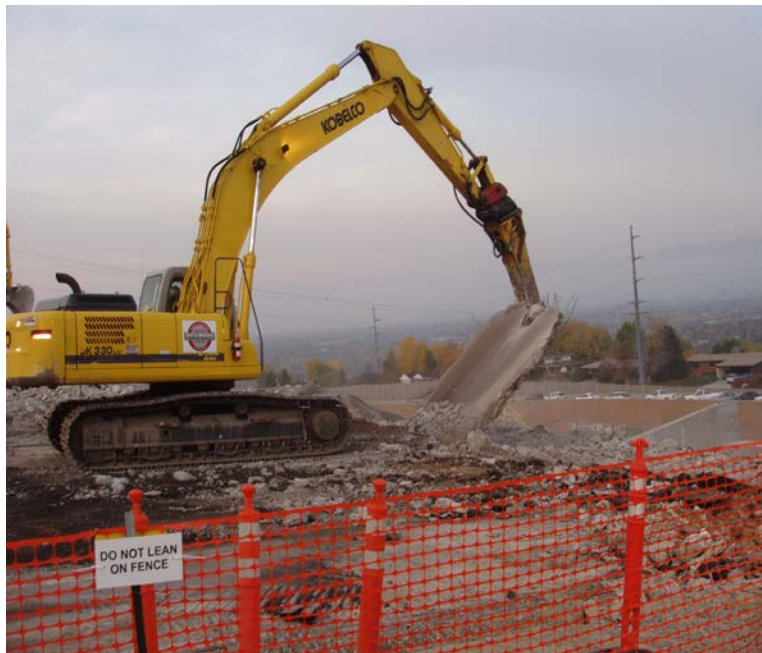
Figure 17. Approach panel removal.
