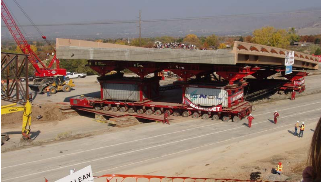
Figure 22. Moving the new superstructure.
