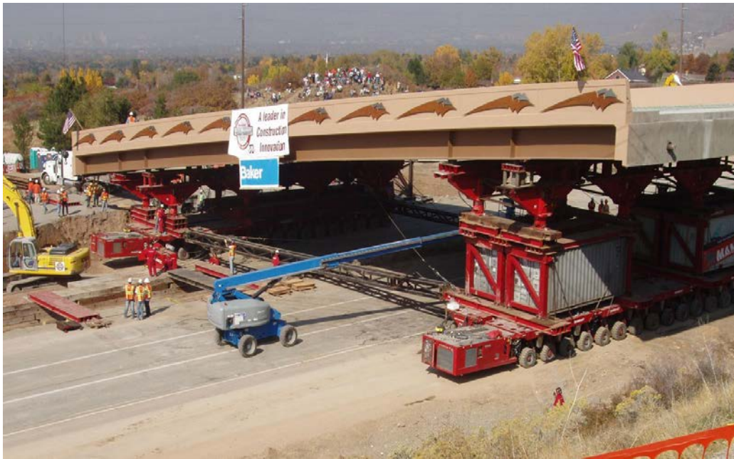
Figure 23. Another view of moving the superstructure.
