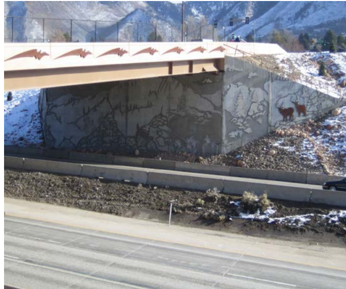
Figure 26. View of the new 4500 South Bridge.
