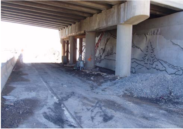
Figure 8. View of the CIP abutment.
