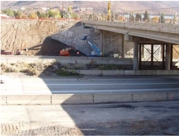
Figure 9. View of CIP wingwall.
