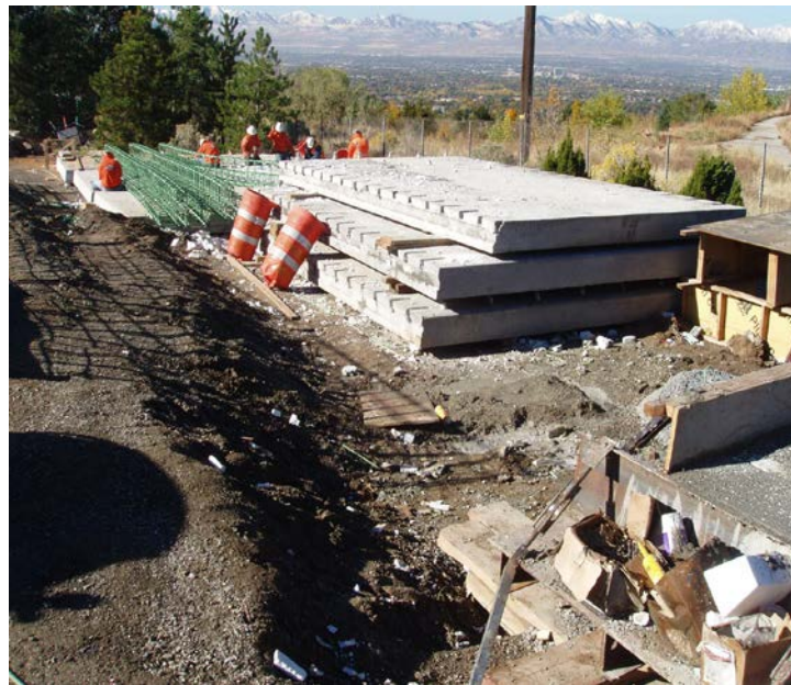
Figure 14. Precast approach slabs.
