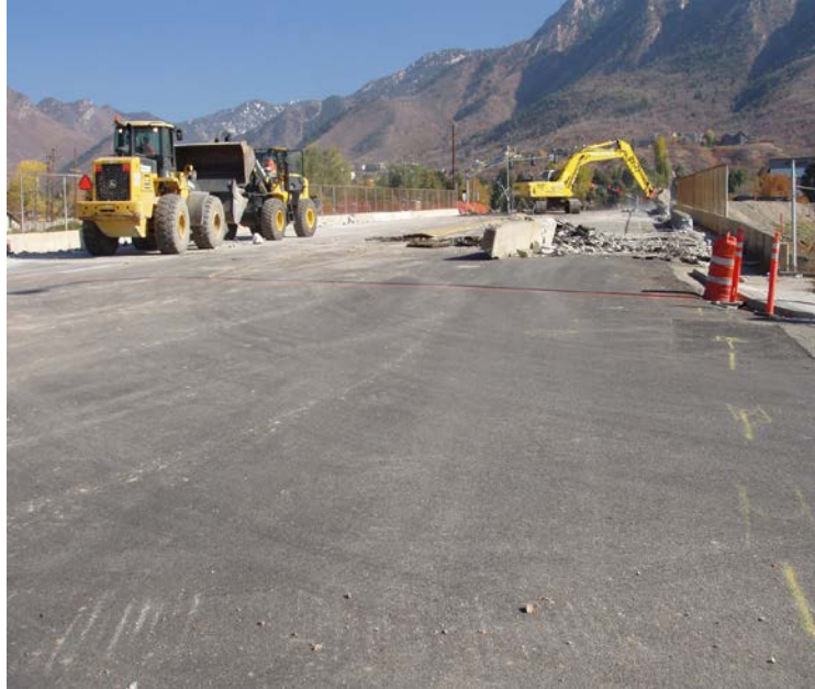
Figure 16. Demolition of railing and median.
