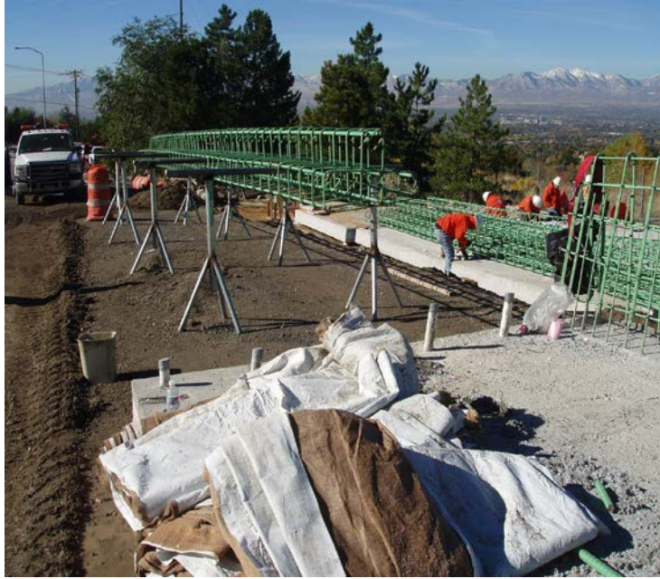
Figure 15. Sleeper slab reinforcement assembly.
