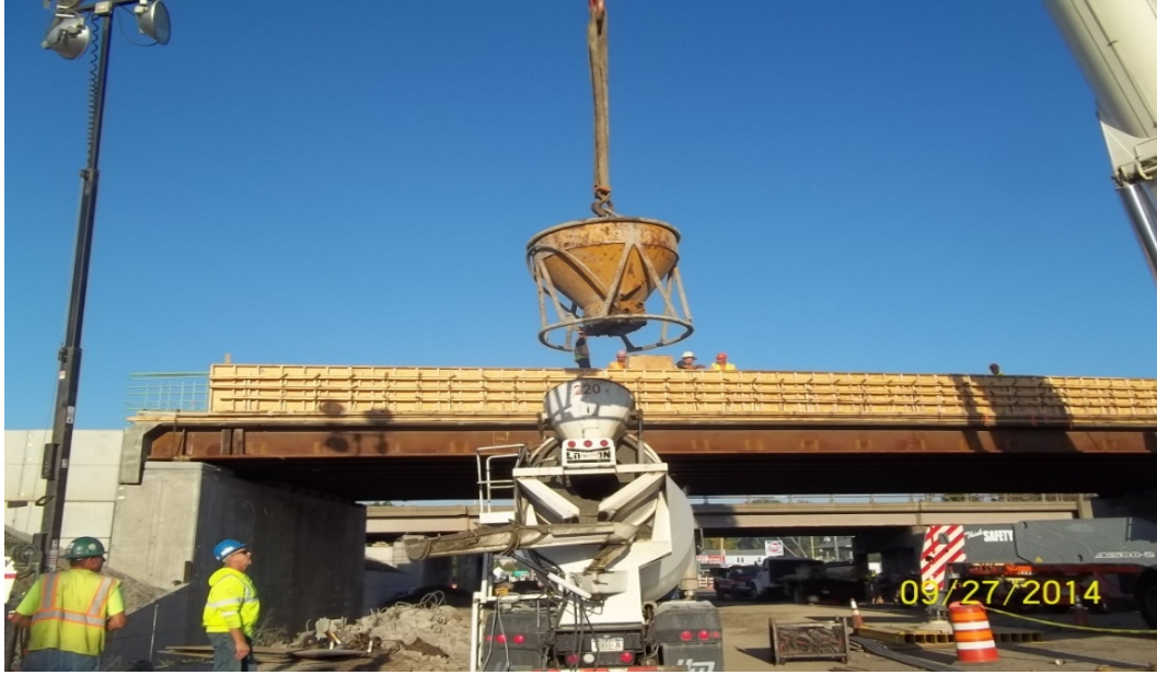
Figure 31. Photo. Concrete being poured in parapet.
