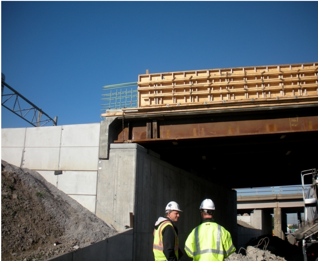
Figure 30. Photo. View of modular deck units, abutment stem, and modular wall.
