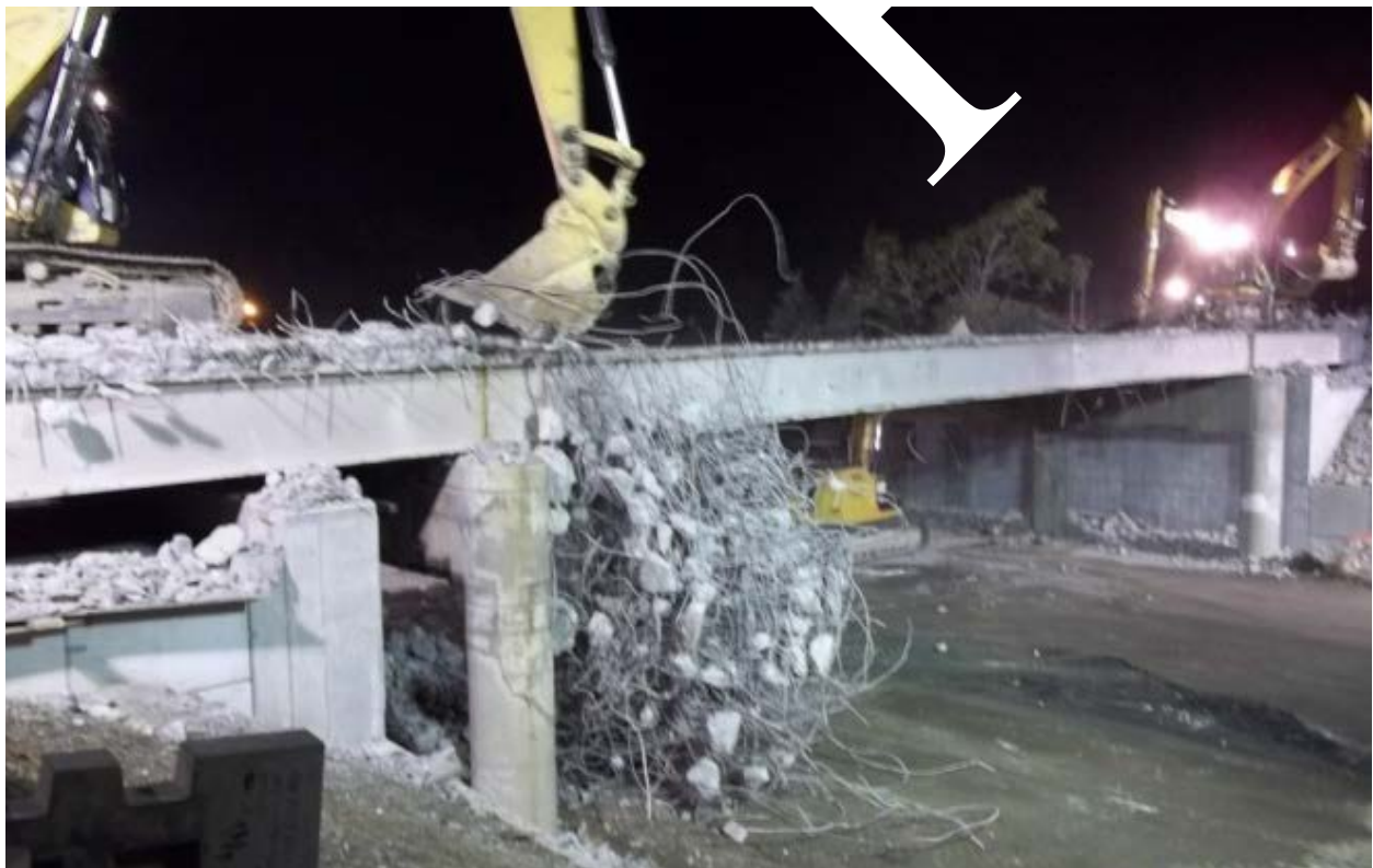
Figure 24. Photo. Demolition of existing structure.
