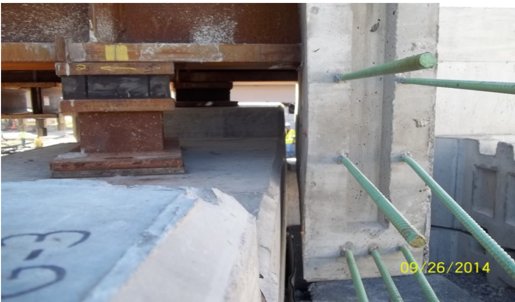
Figure 28. Photo. Close-up of deck beams resting on bearings.
