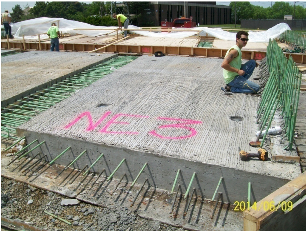
Figure 23. Photo. Precast slab preparation in progress at yard.
