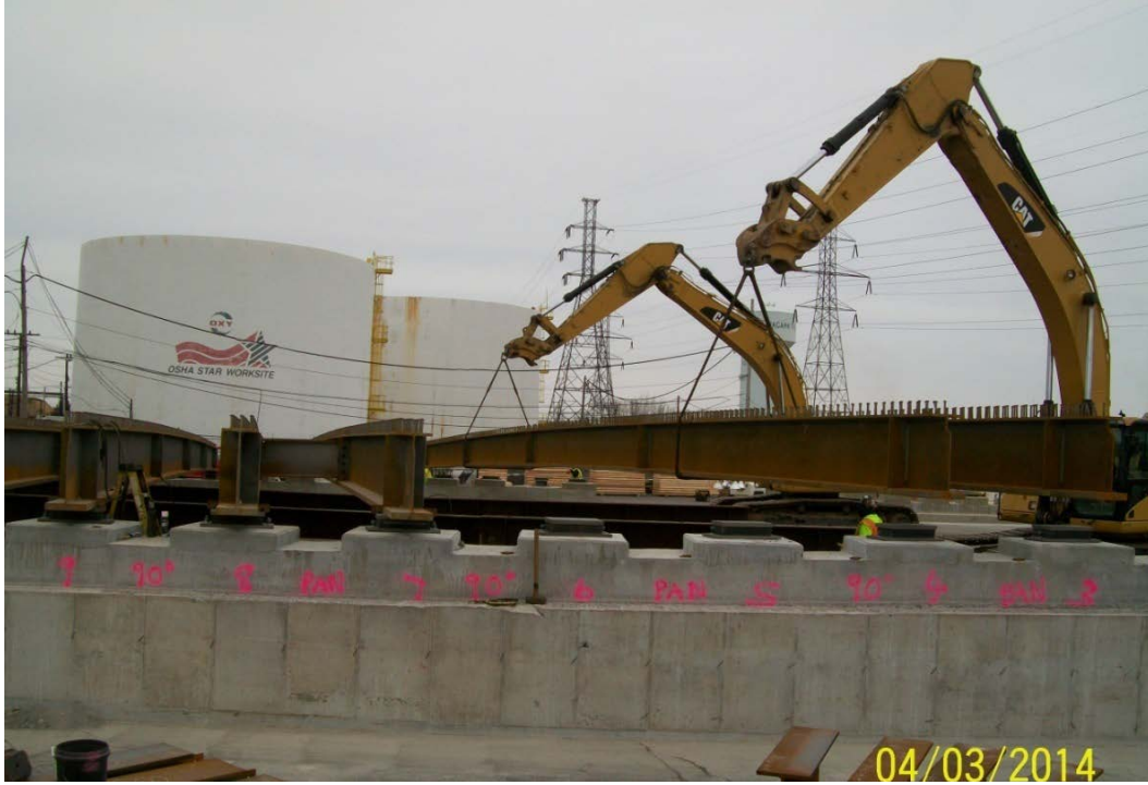
Figure 20. Photo. Steel beams being placed on simulated abutments in yard.
