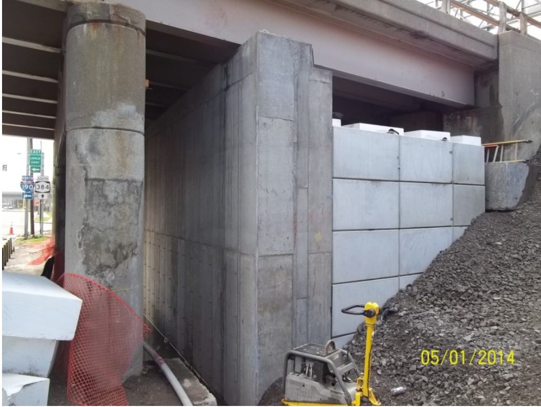
Figure 18. Photo. New abutment, modular walls, and space filled with EPS blocks.
