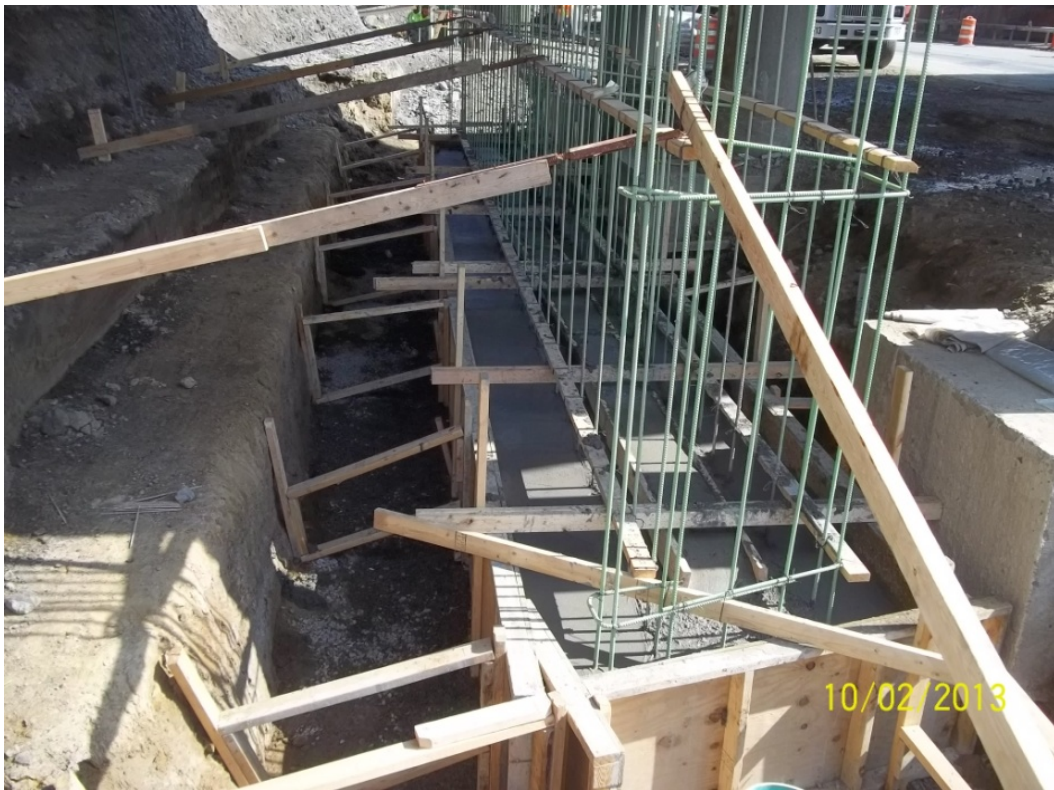
Figure 15. Photo. Construction of footings and reinforcement for abutment stems.
