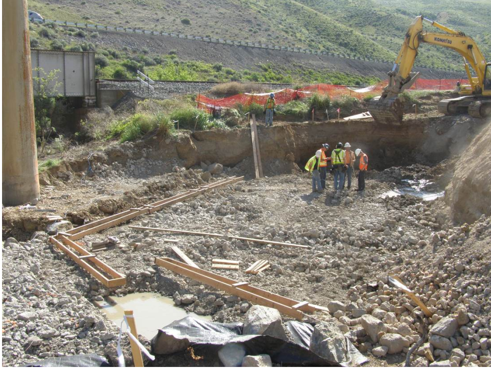
Figure 21. Setting the forms for building the substructure and MSE retaining wall.
