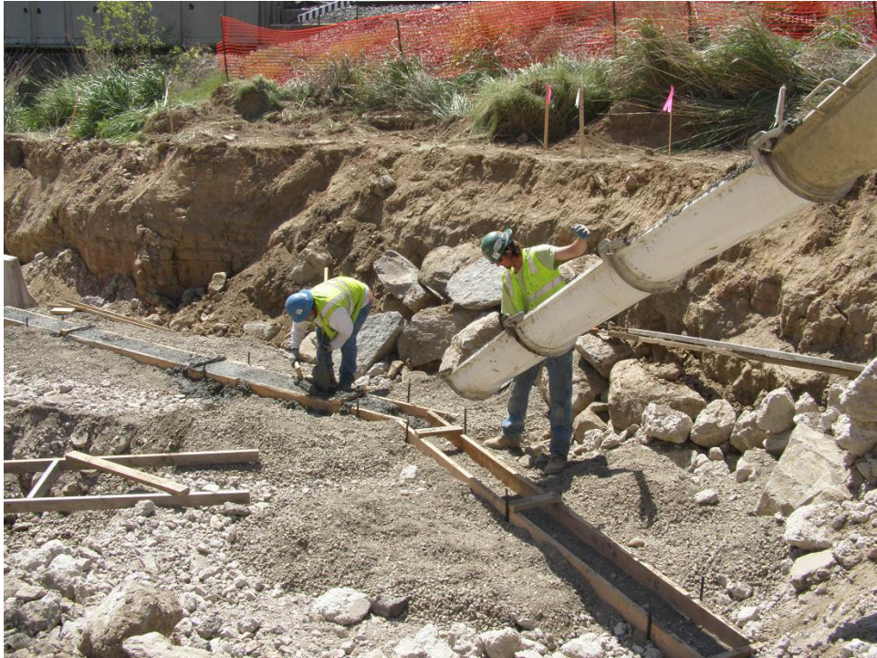
Figure 22. Pouring concrete for building the substructure and MSE retaining wall.
