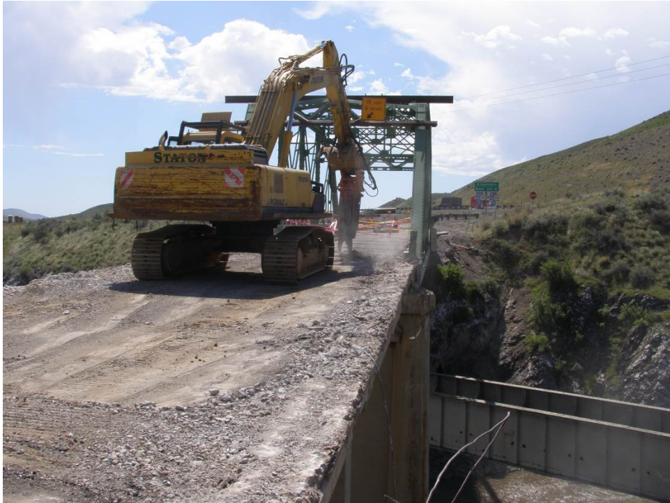
Figure 17. Demolition of approach to bridge 0700.
