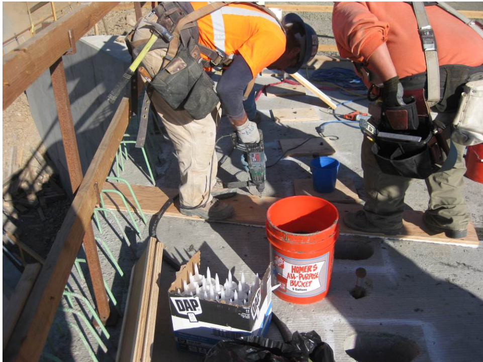
Figure 54. Plywood used to top-form filled areas of UHPC to prevent overflowing.
