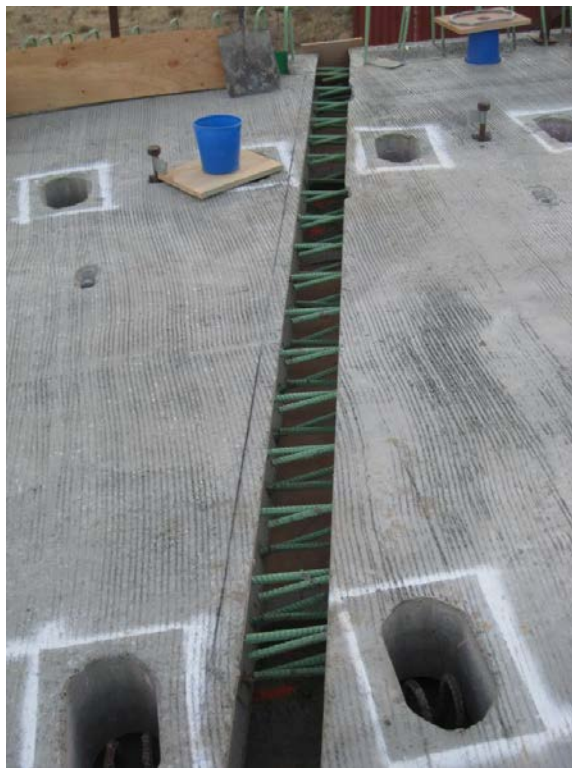
Figure 44. Transverse view of the joint between the deck panels. Composite action between panels is obtained when the reinforced transverse joints are filled with the UHPC. The use of UHPC also eliminates the need for longitudinal posttensioning.
