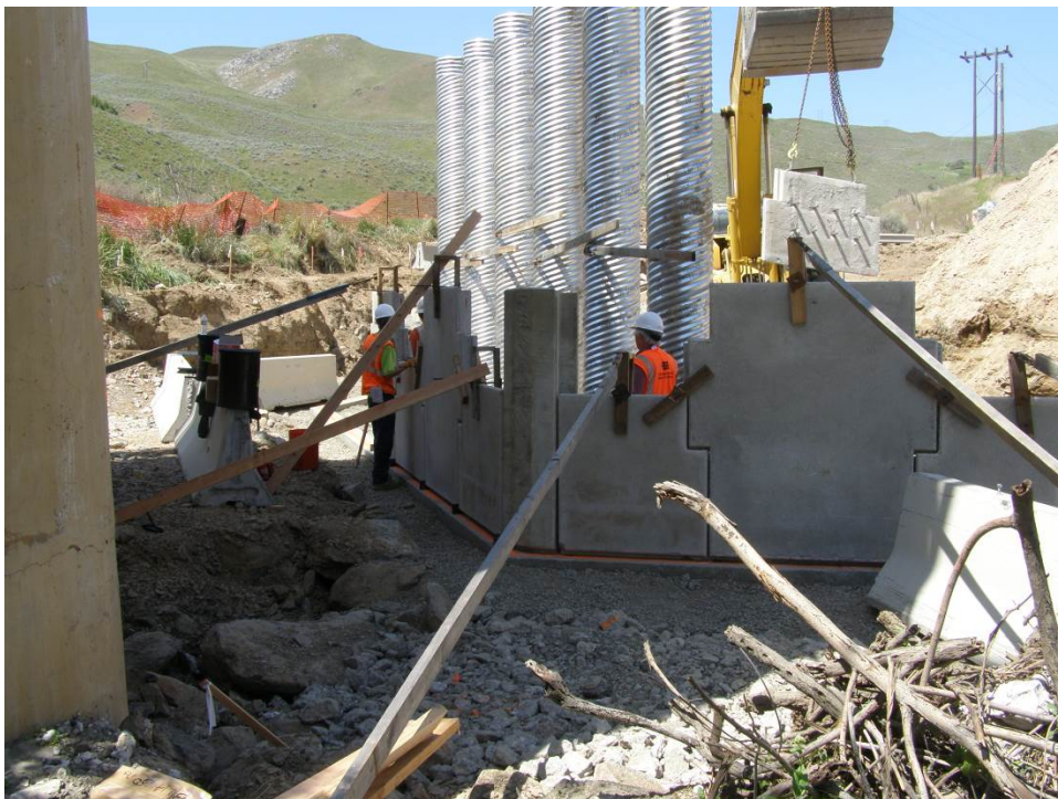
Figure 24. Installing MSE retaining wall (side view).
