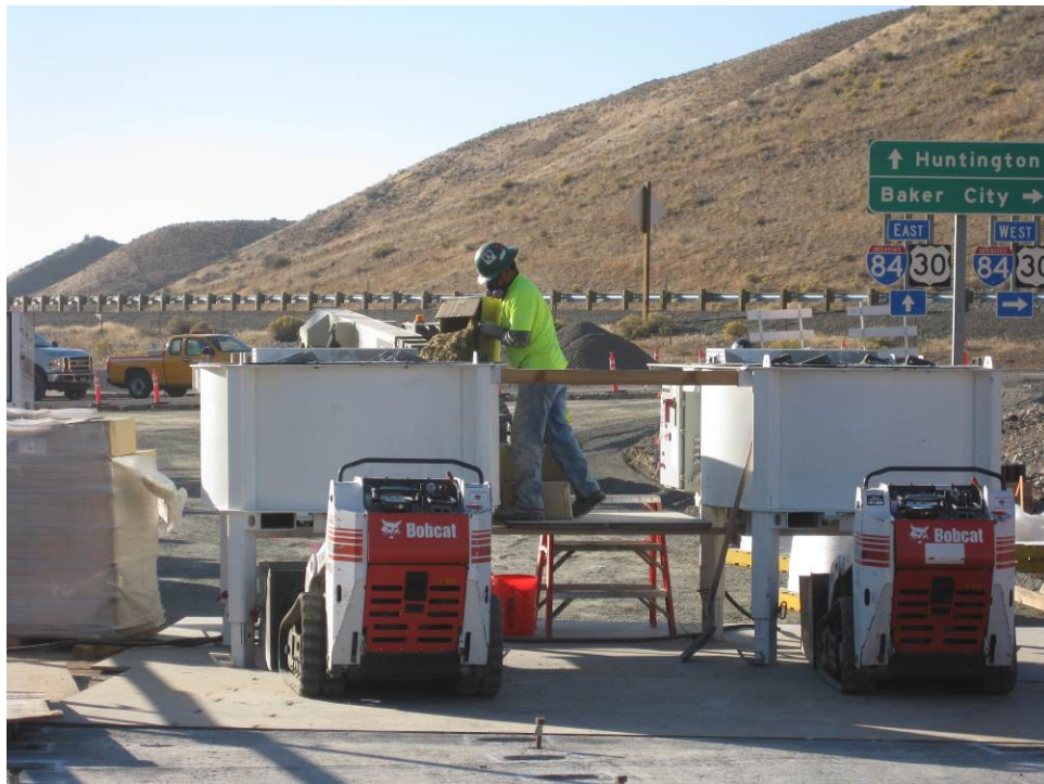
Figure 48. UHPC fiber being put in the mixer.
