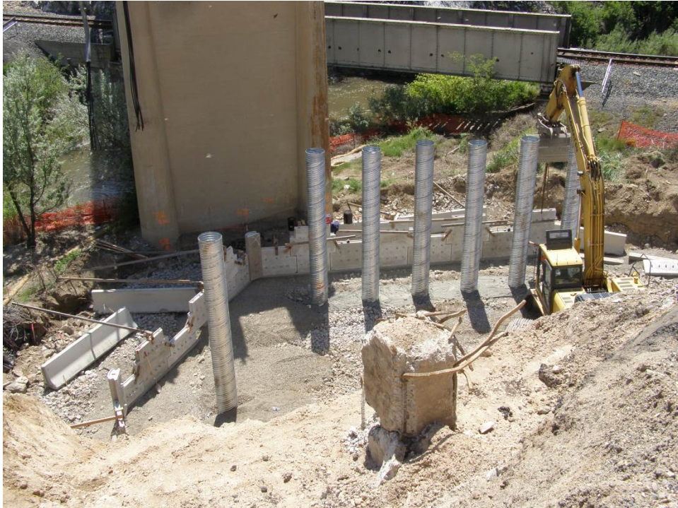
Figure 26. Installing MSE retaining wall (top view).
