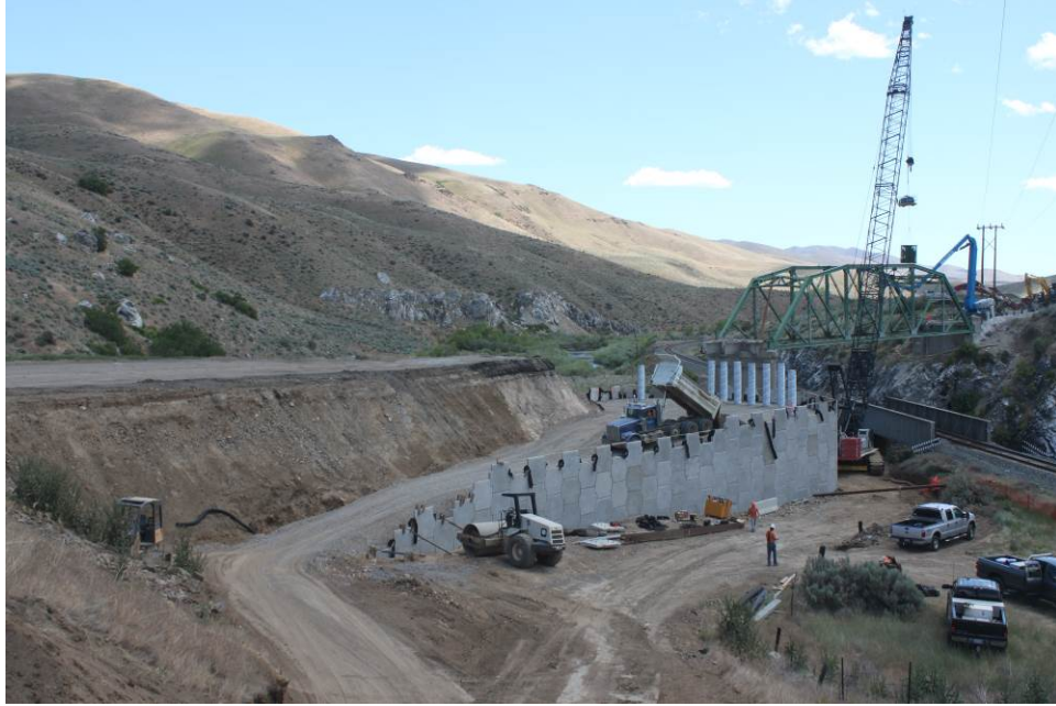
Figure 27. Backfilling MSE retaining wall (long view).
