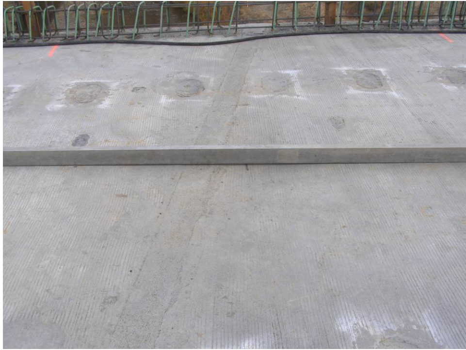
Figure 56. Close-up view of bridge 21252 deck surface after completion.
