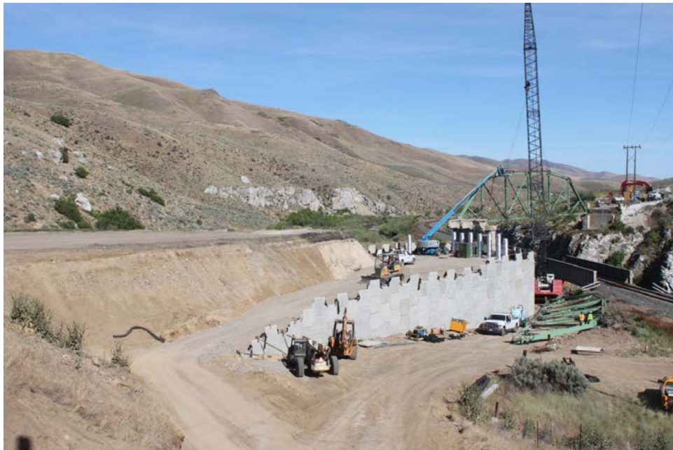
Figure 28. Removal of truss frame of existing bridge 0700 (long view).
