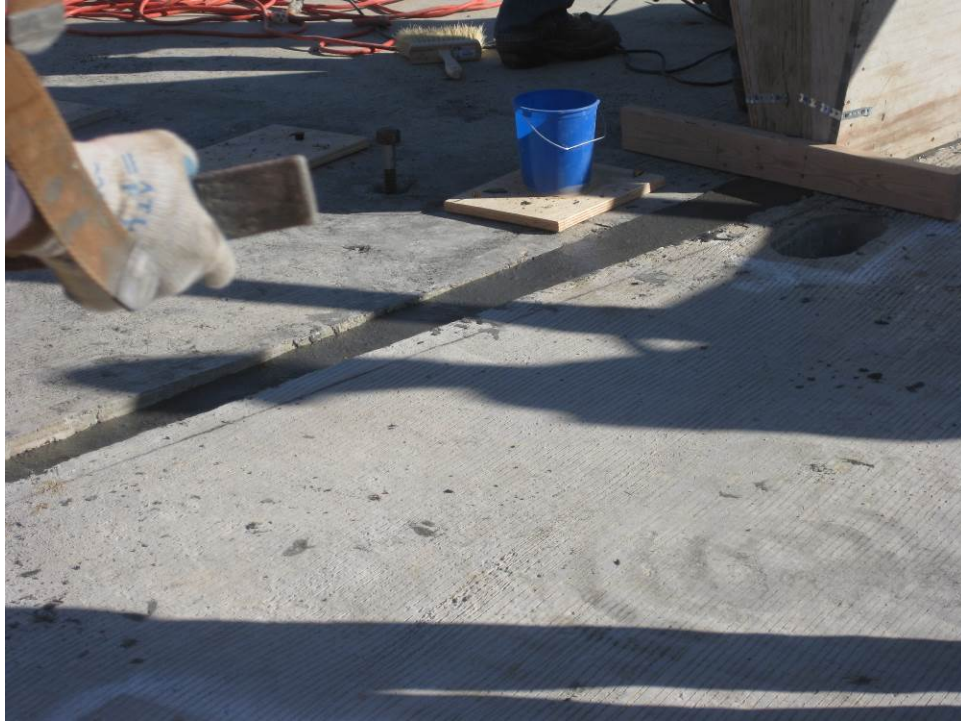
Figure 53. UHPC flowing into the transverse joint.
