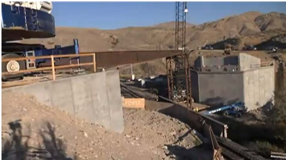
Figure 30. Completed installation of falsework to temporarily support the girders during construction of the superstructure.
