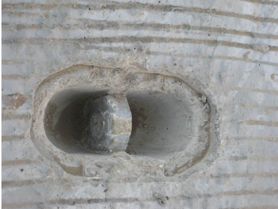
Figure 41. Lifting hardware cast into each individual bridge deck panel.
