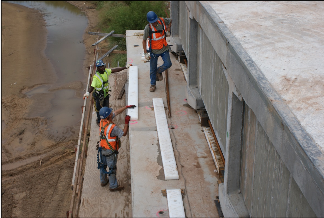
Figure 13. Photo. Hard plastic rails attached to pier caps.
