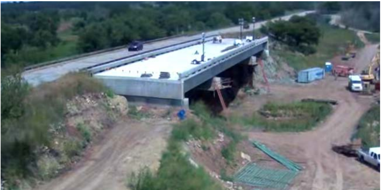
Figure 10. Photo. Completed deck alongside existing structure (courtesy: ODOT).
