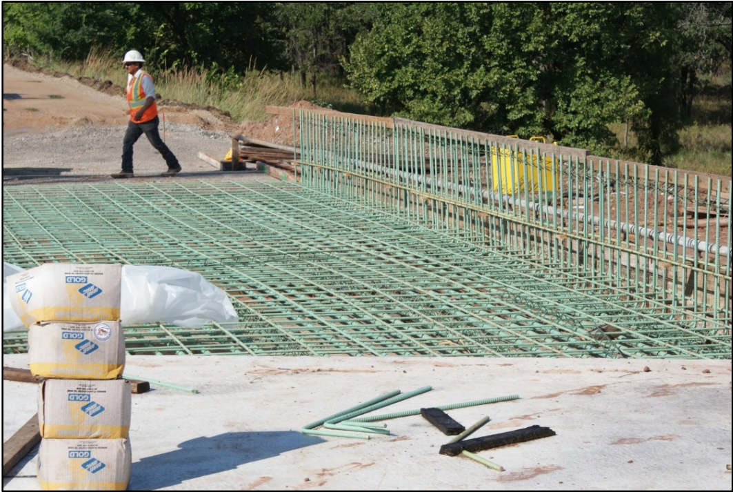
Figure 19. Photo. Steel in place for approach slab pour.
