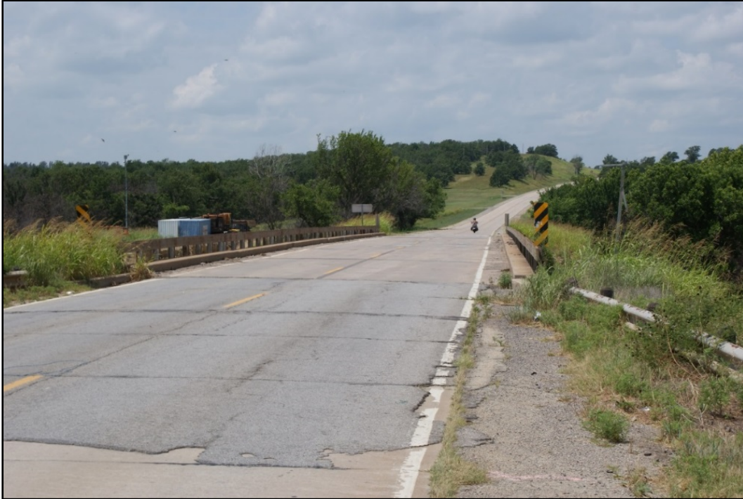
Figure 2. Photo. Existing structure 15375 on SH 51.
