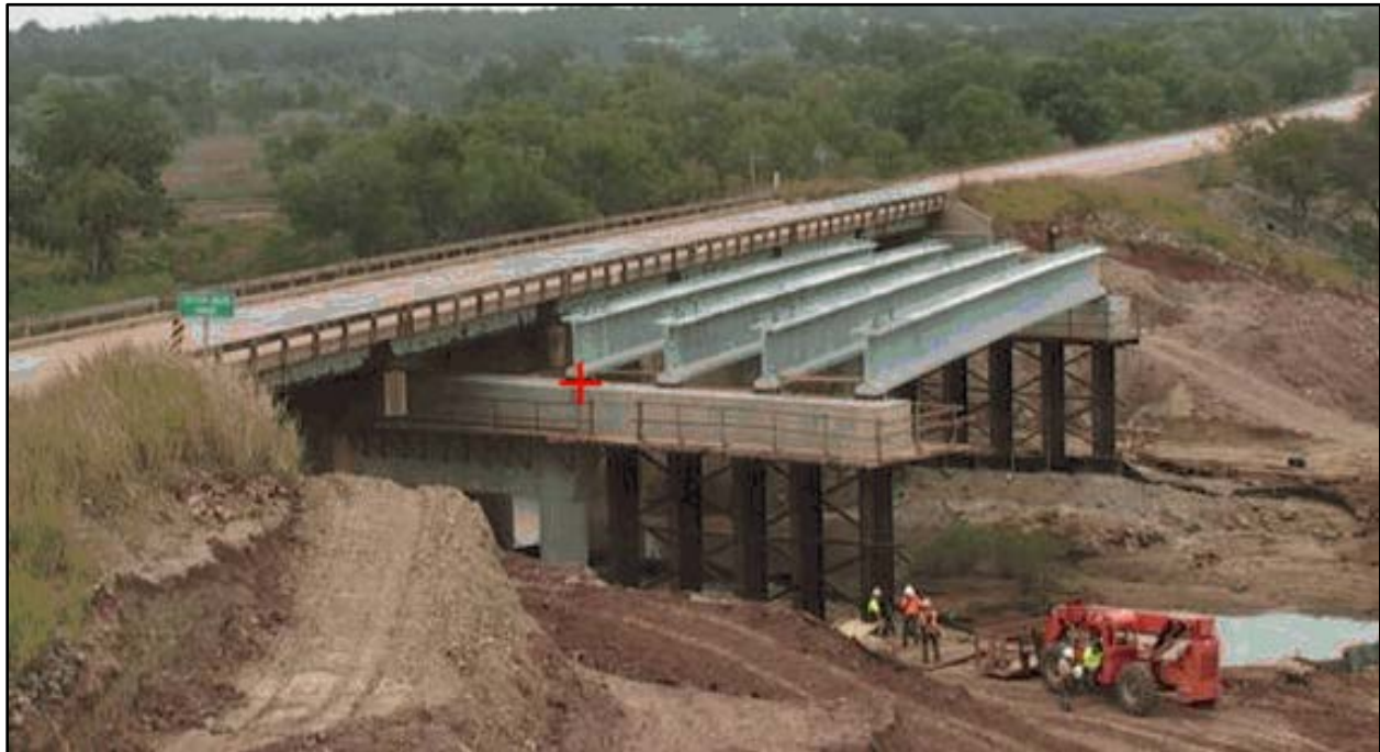
Figure 8. Photo. Center section of concrete girders in place (courtesy: ODOT).
