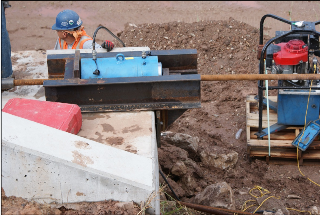
Figure 15. Photo. Screw jack attached to end of abutment to facilitate pull.
