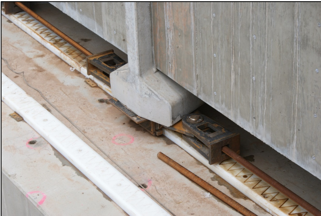
Figure 16. Photo. Threaded rod run through sled under girders.
