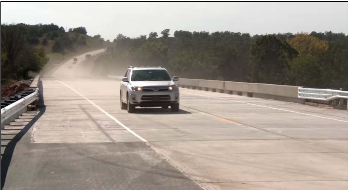
Figure 20. Photo. Traffic on completed structure (courtesy: Google Earth).
