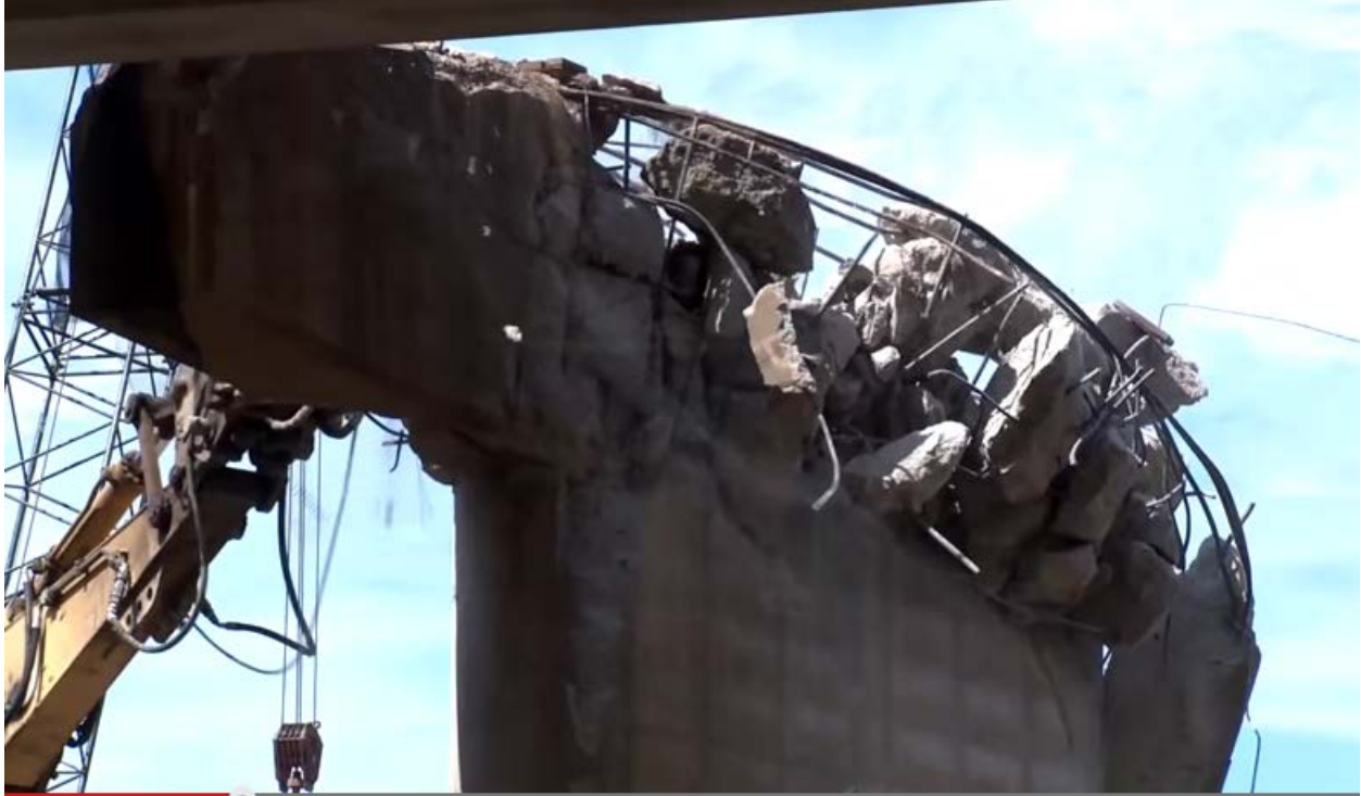
Figure 11. Photo. Removal of existing piers (courtesy: ODOT).
