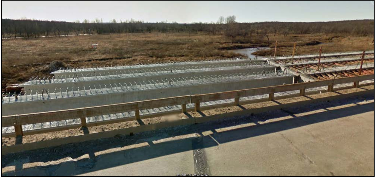
Figure 9. Photo. Concrete girders in place on falsework (courtesy: Google Earth).
