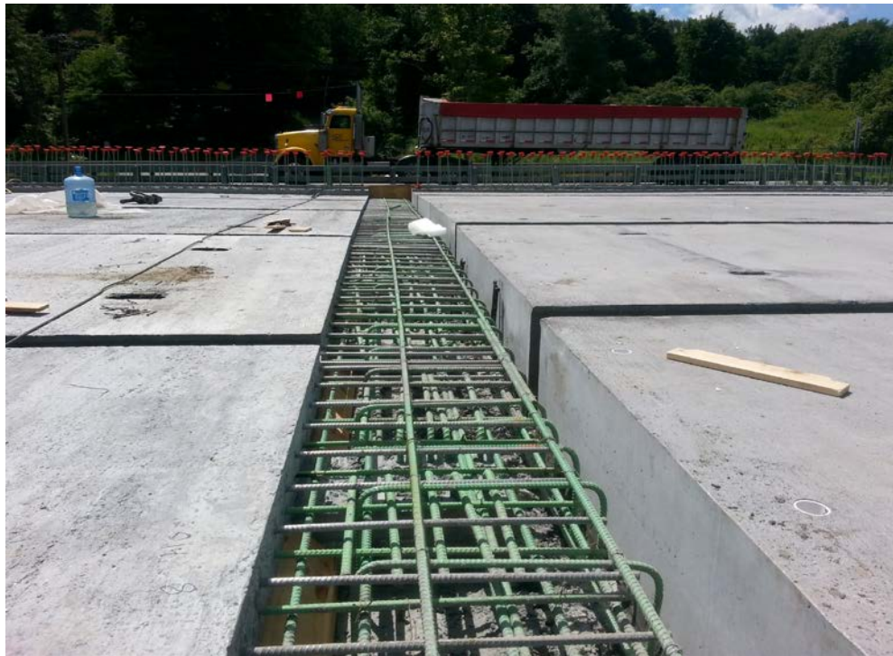
Figure 25. Photo. Close-up of reinforcement connecting beams and approach slab.
