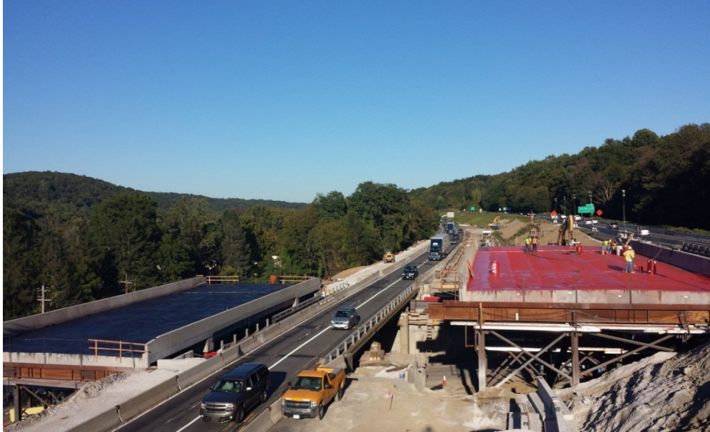
Figure 31. Photo. Westbound structure ready for move.
