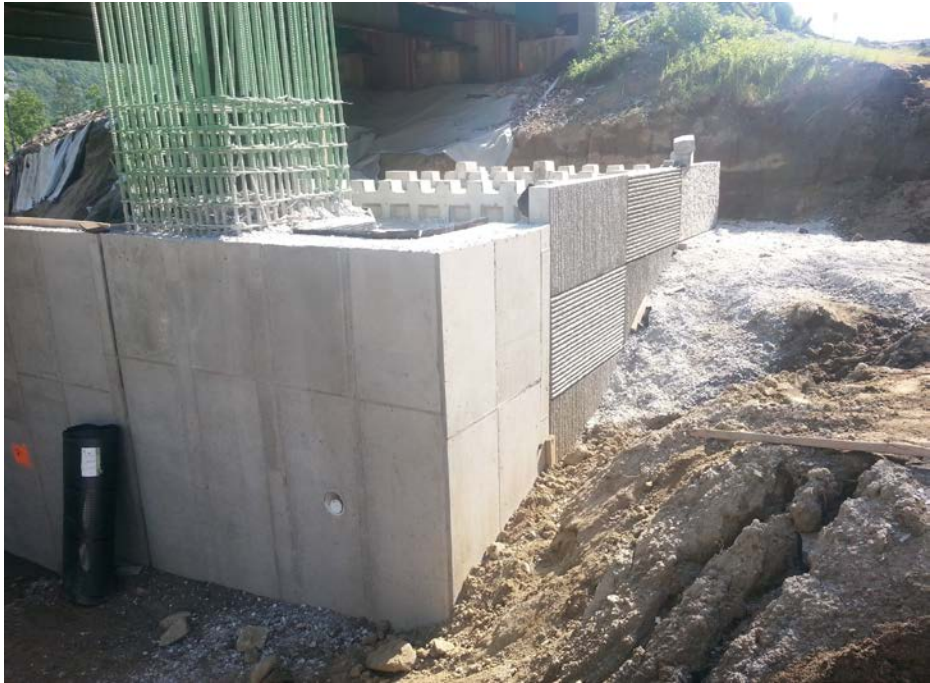
Figure 18. Photo. Installation of the T-wall used for abutment wings.
