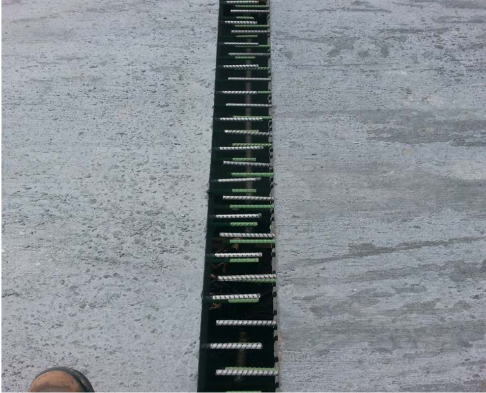
Figure 24. Photo. Close-up of reinforcement of adjacent NEXT beam elements.
