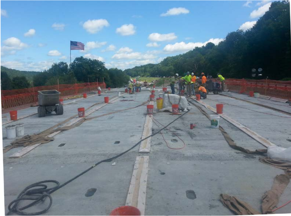
Figure 26. Photo. UHPC closure pours in progress.
