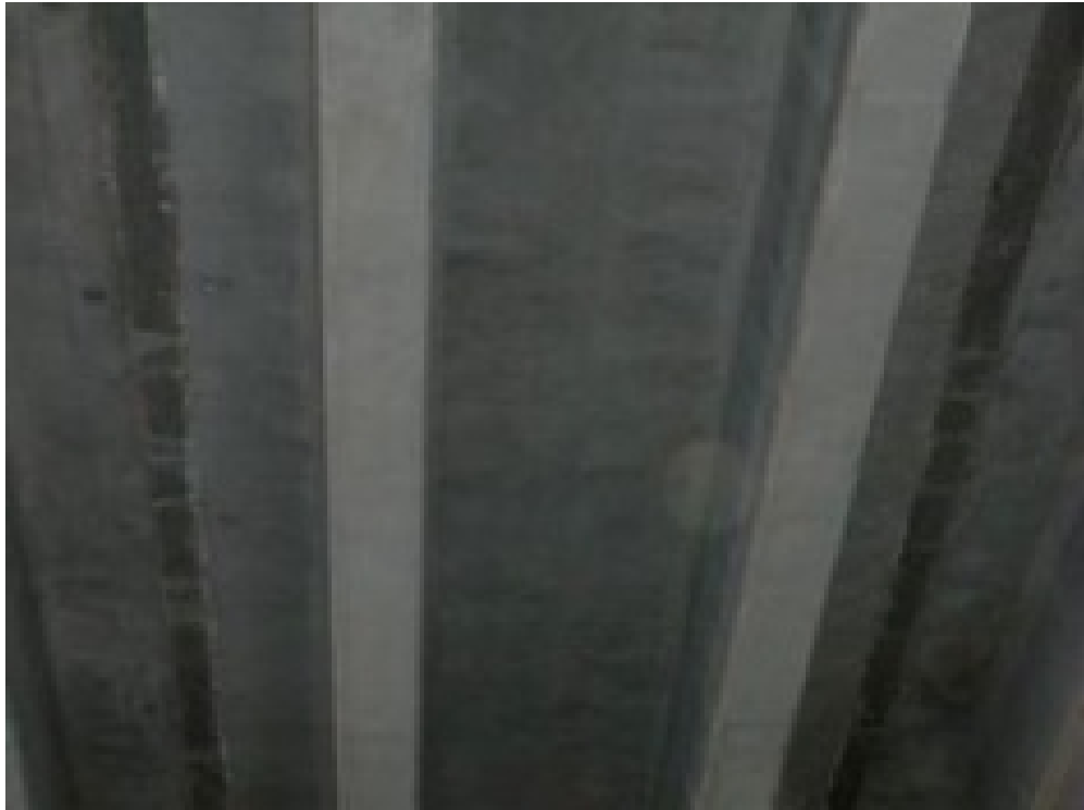
Figure 27. Photo. Close-up of NEXT beam from underneath after UHPC pour.
