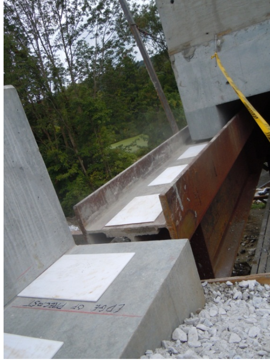
Figure 39. Photo. Close-up at approach slab end.
