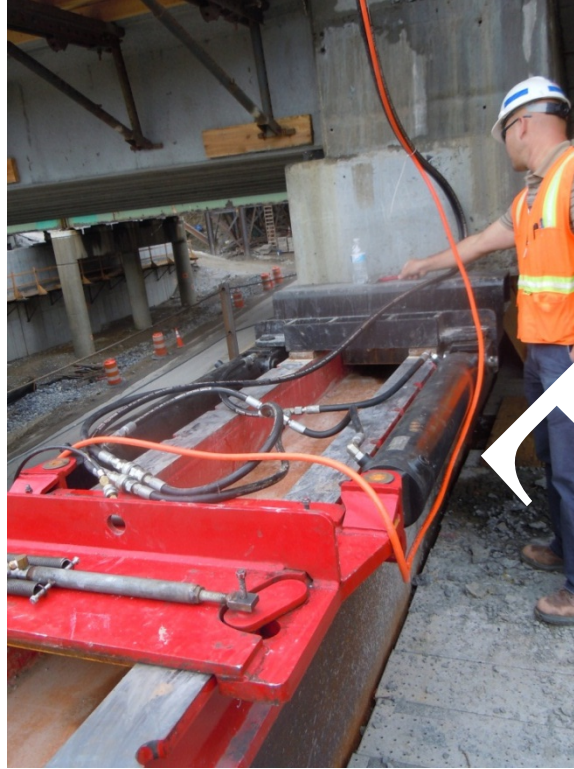
Figure 34. Photo. Push Gripper assembly pushing the end diaphragm.
