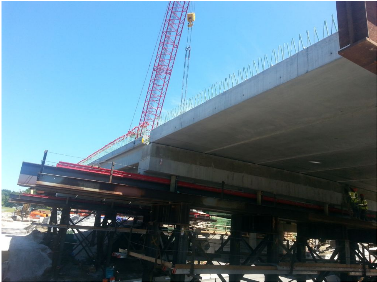
Figure 11. Photo. Primary bent in the foreground and secondary bent in the background.
