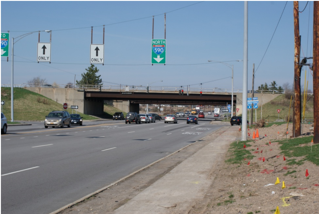
Figure 4. View of Winton Road before construction from the south.
