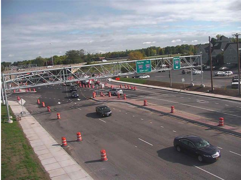
Figure 9. Screen capture from camera on NYSDOT Web site.
