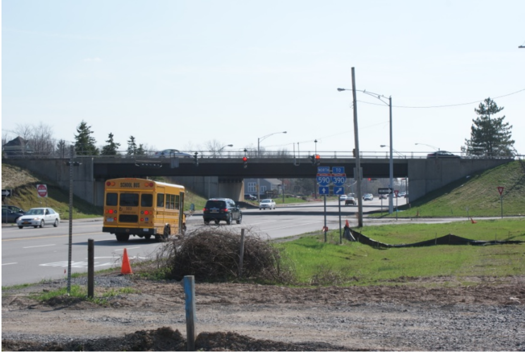
Figure 3. View of Winton Road before construction from the north.
