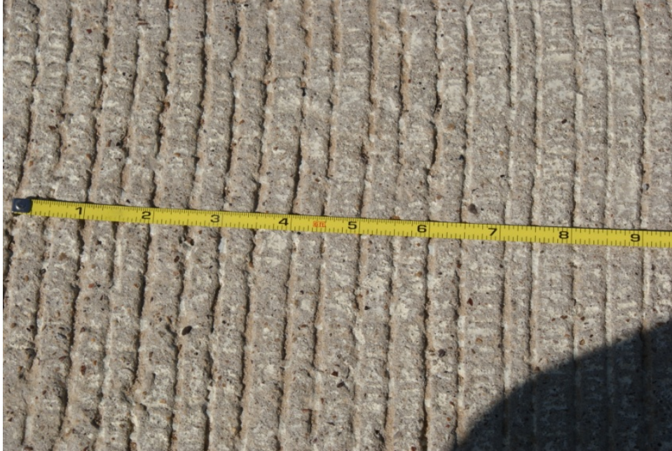
Figure 15. Typical texture of 1/2 inch transversely tined surface.
