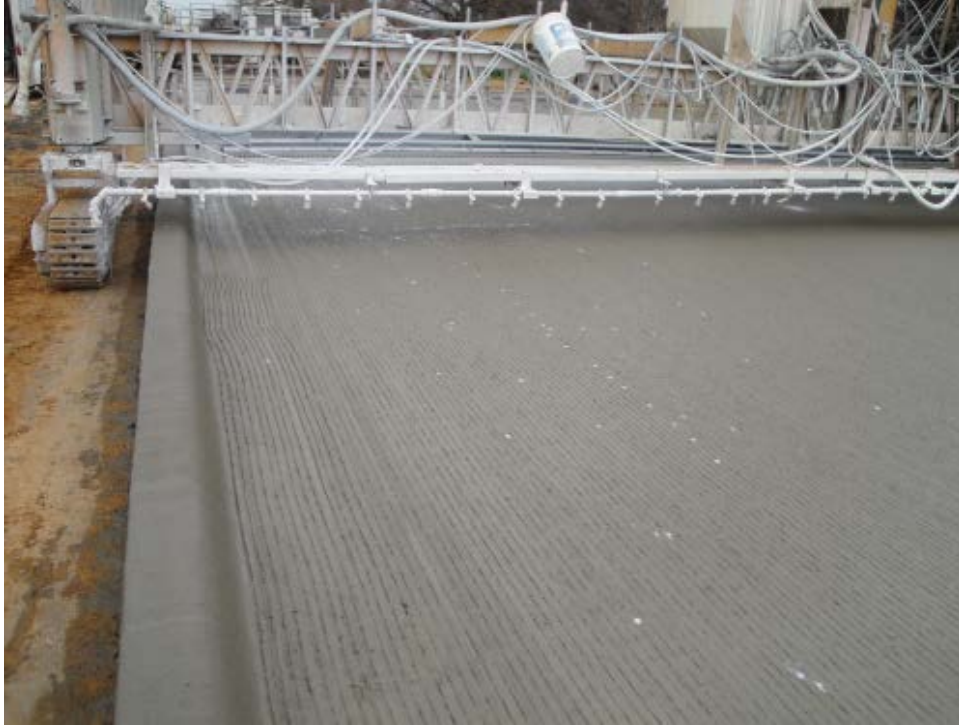
Figure 13. Typical texture of longitudinally tined surface.
