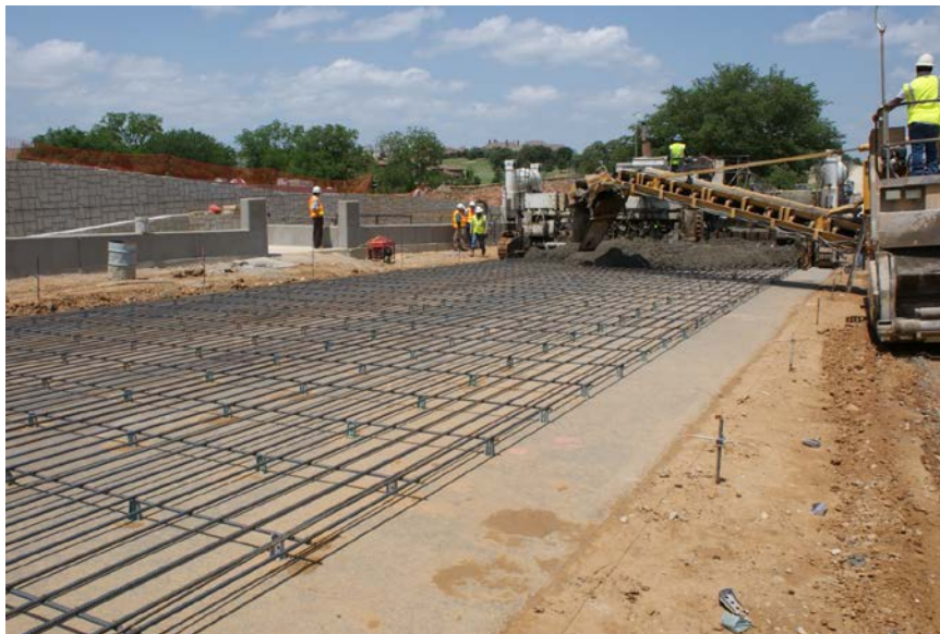
Figure 20. Placement of rebar assembly.
