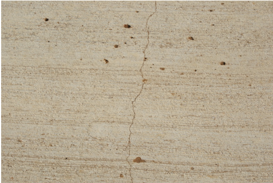
Figure 14. Typical texture of carpet drag surface.
