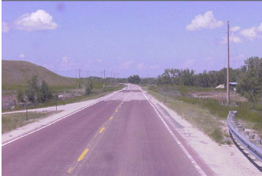
Figure 7. Photo. Beginning of pavement section (courtesy: Wyoming DOT)
