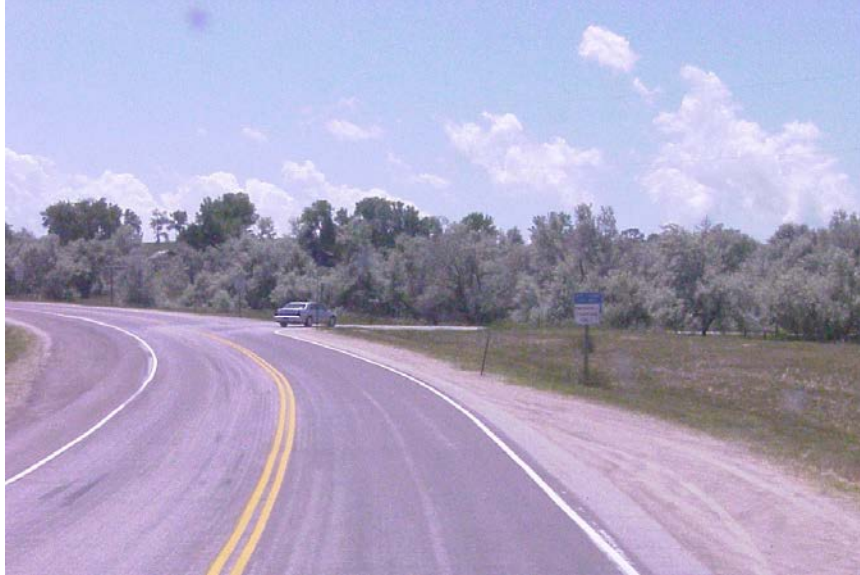
Figure 9. Photo. End of pavement section (courtesy: Wyoming DOT)
