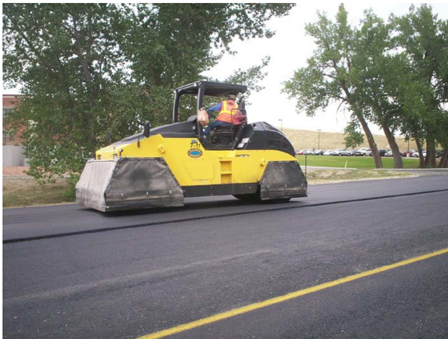
Figure 23. Photo. Pneumatic roller. (courtesy: Wyoming DOT)
