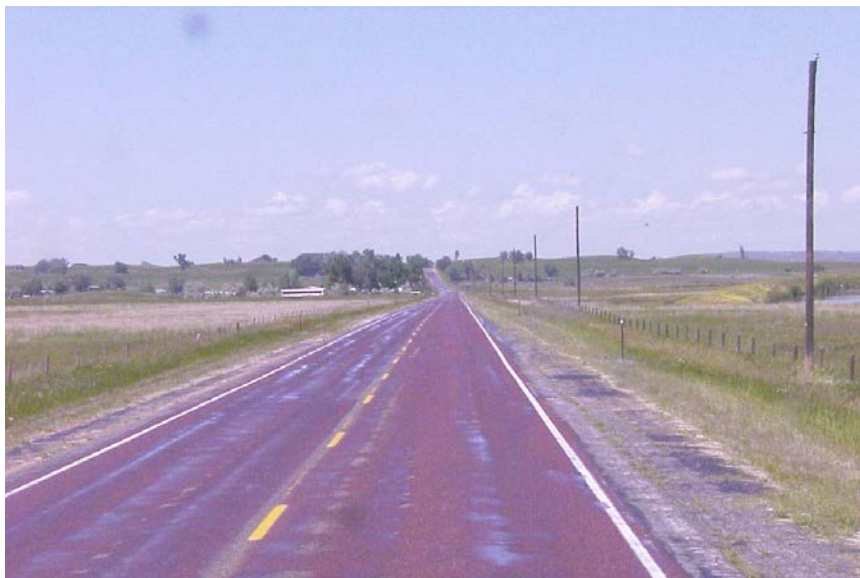
Figure 8. Photo. Middle of pavement section (courtesy: Wyoming DOT)
