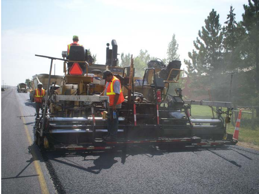
Figure 24. Photo. HMA paving. (courtesy: Wyoming DOT)
