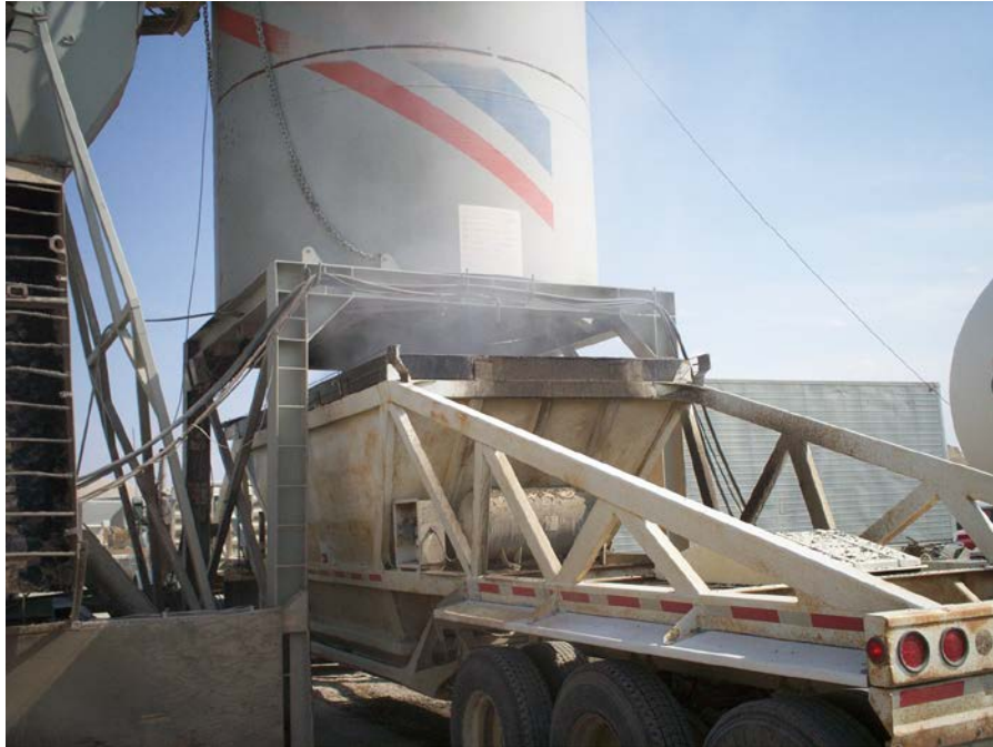
Figure 26. Photo. Truck Loading (courtesy: Wyoming DOT)
