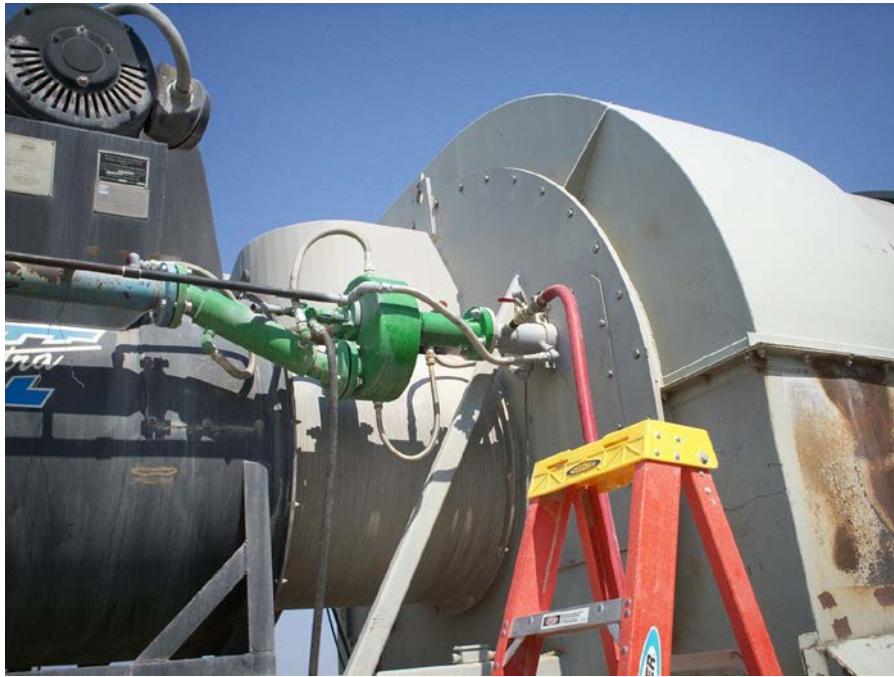
Figure 19. Photo. Foaming device. (courtesy: Wyoming DOT)
