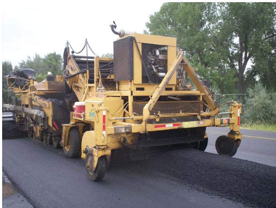
Figure 21. Photo. Elevator and paver. (courtesy: Wyoming DOT)
