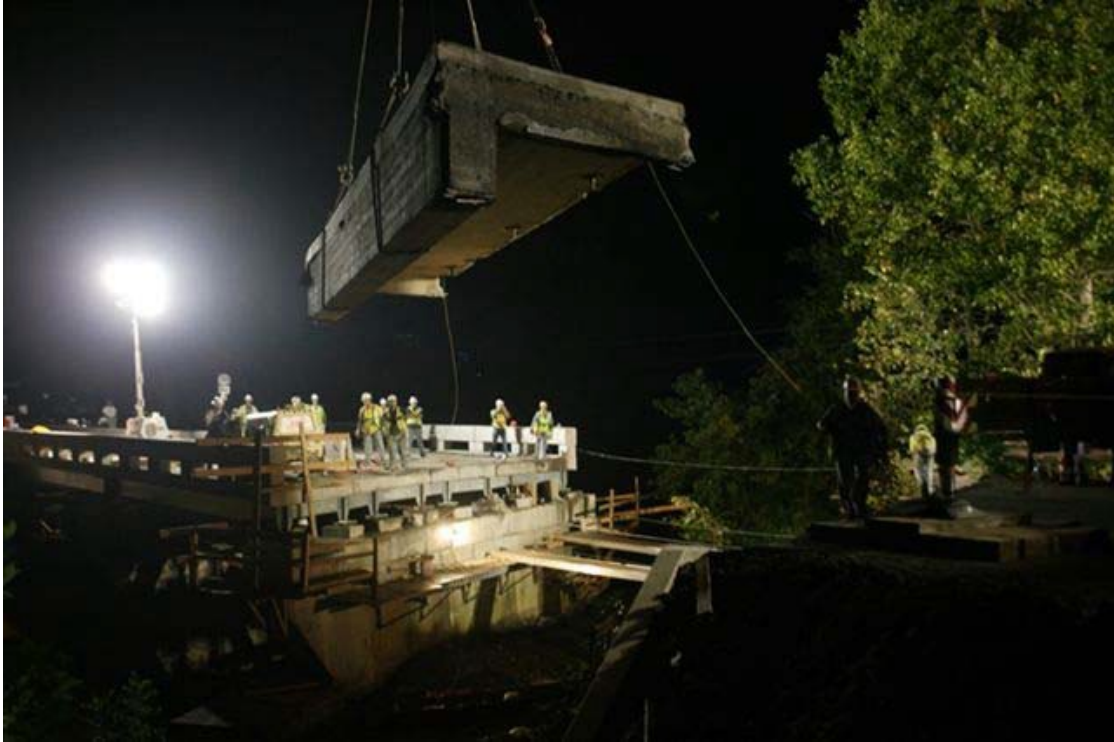
Figure 7. Removal of part of the existing superstructure of the U.S. 15/29 bridge.
