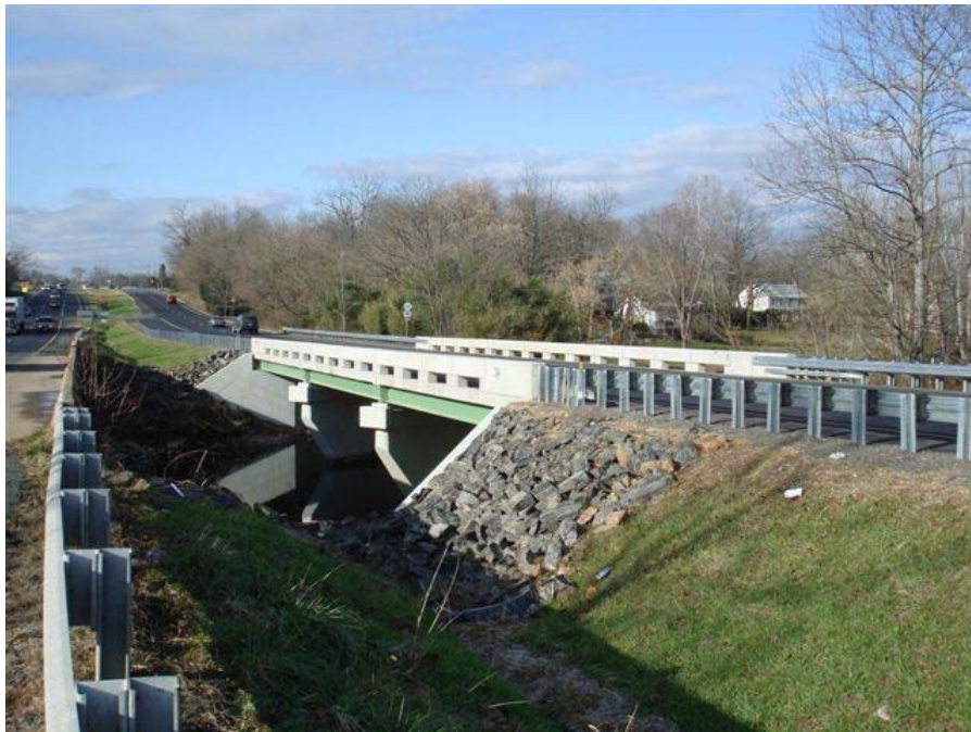
Figure 12. Completed U.S. 15/29 bridge over Broad Run, looking south.
