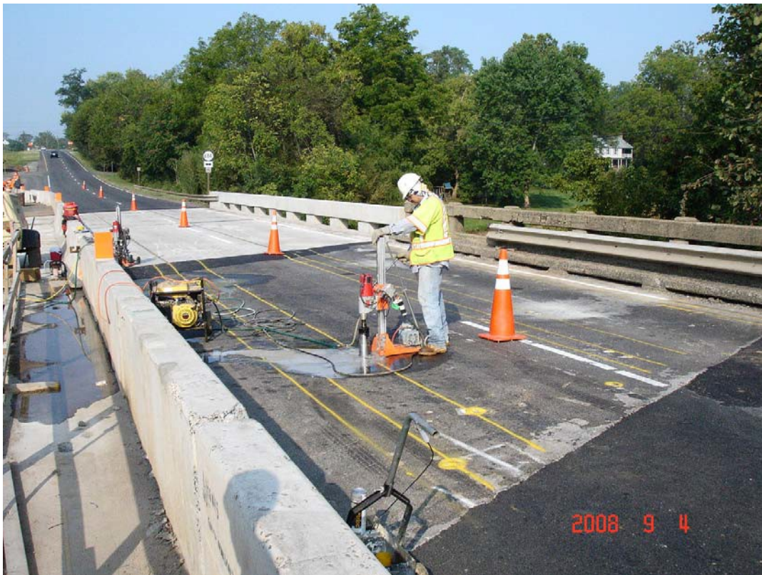
Figure 8. Portion of superstructure replaced on the U.S. 15/29 bridge.
