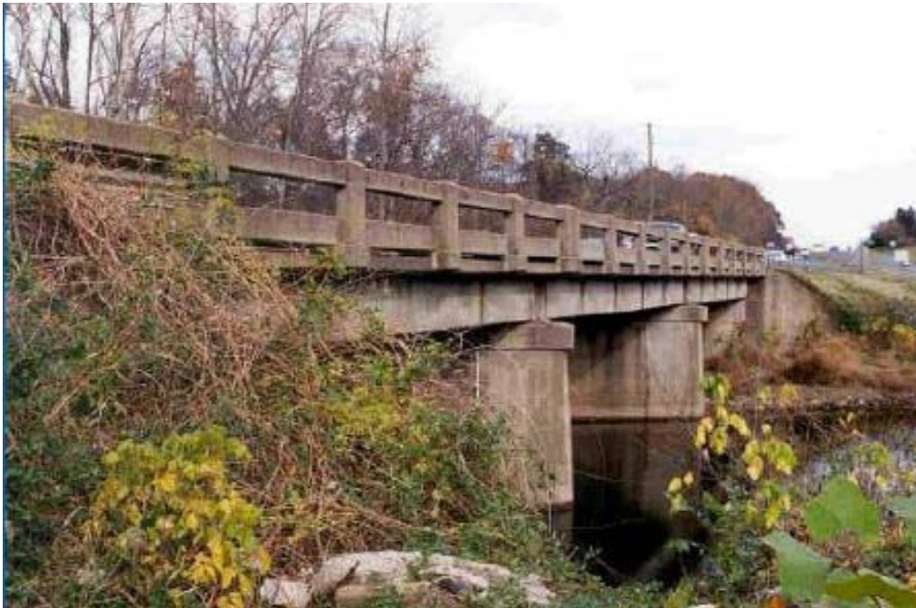
Figure 2. Existing southbound U.S. 15/29 bridge over Broad Run, looking north.
