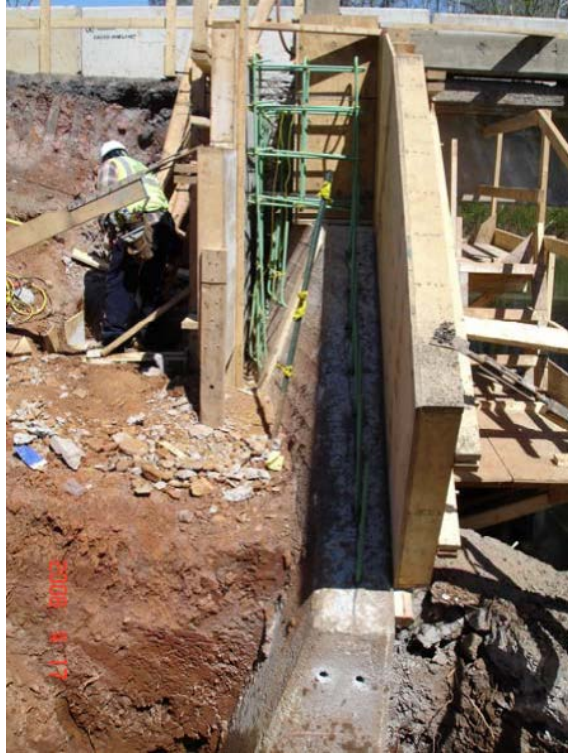
Figure 9. Wingwall modifications on the U.S. 15/29 bridge.
