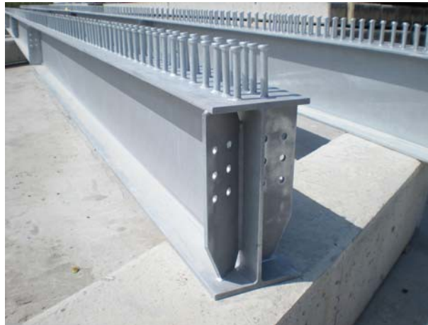
Figure 4. Steel beams for U.S. 15/29 bridge at Coastal Precast Systems precasting yard.
