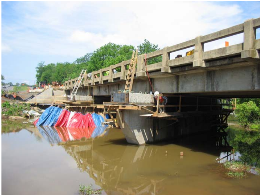
Figure 10. Pier widening on the U.S. 15/29 bridge.
