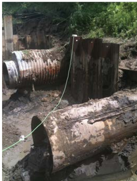
Figure 5 – Steel Casing and Existing Culvert with Liner
