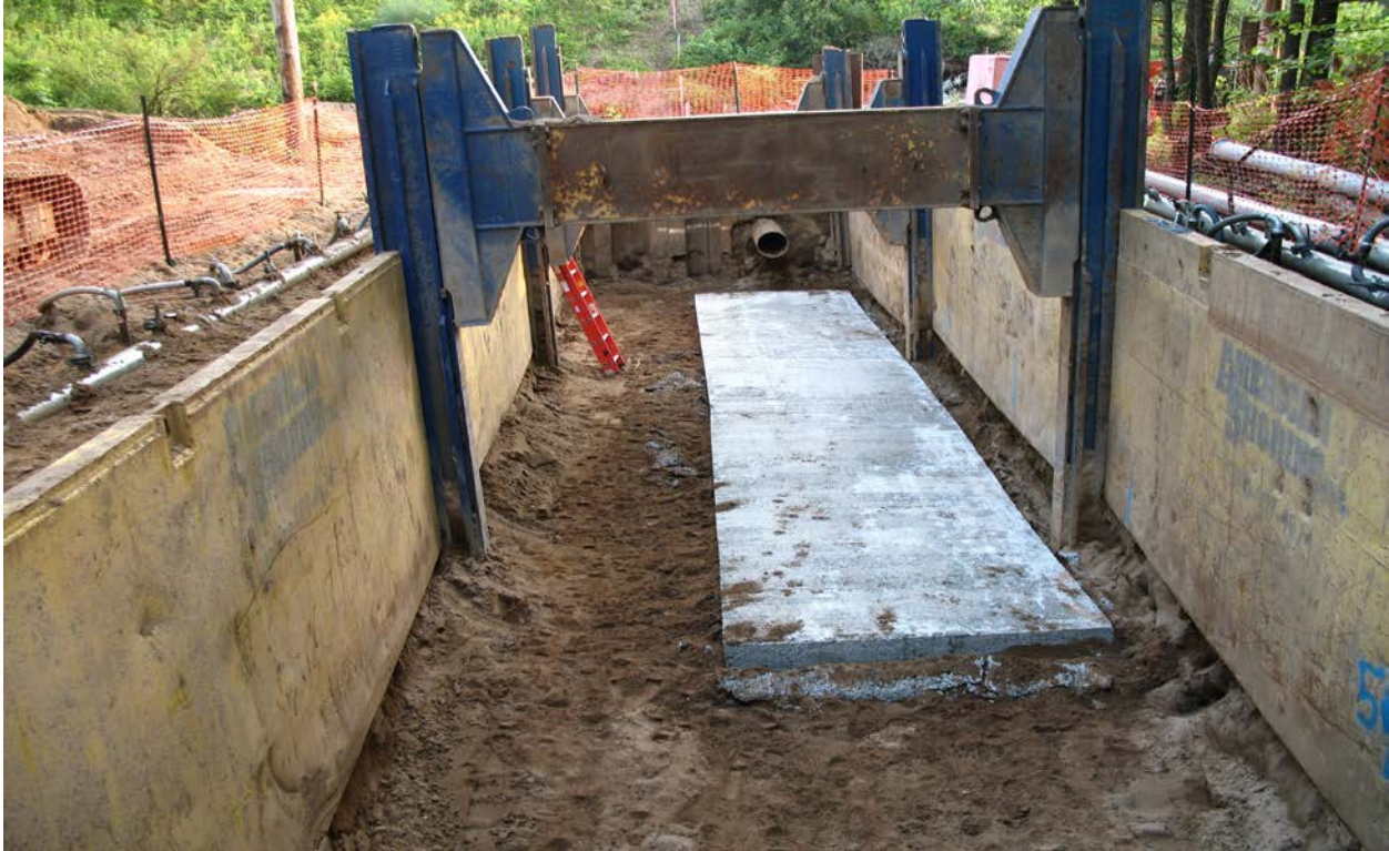
Figure 13. Concrete slab for pipe ramming equipment.
