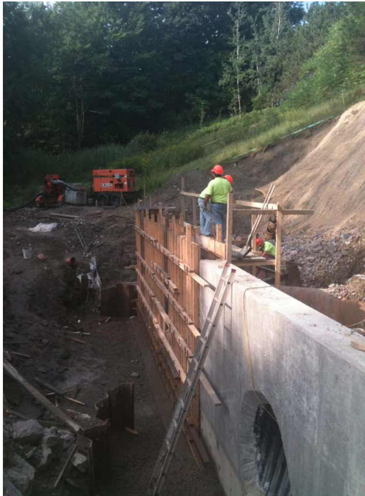
Figure 20. Headwall under construction for additional pipe.
