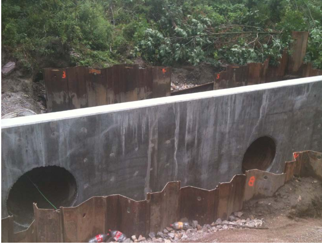
Figure 21. Completed headwall showing both pipes.
