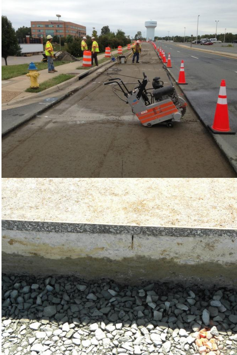
Figure 14. Photos. Joint sawing and AC surfacing over a sawcut in the RCC layer
