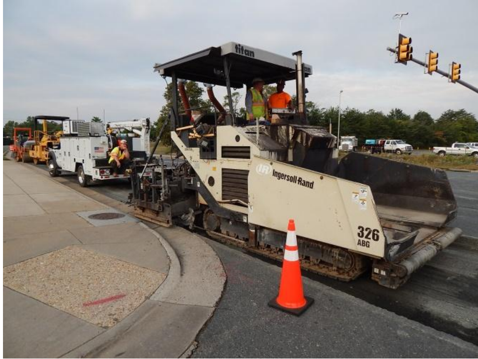
Figure 8. Photo. Asphalt paver used.
