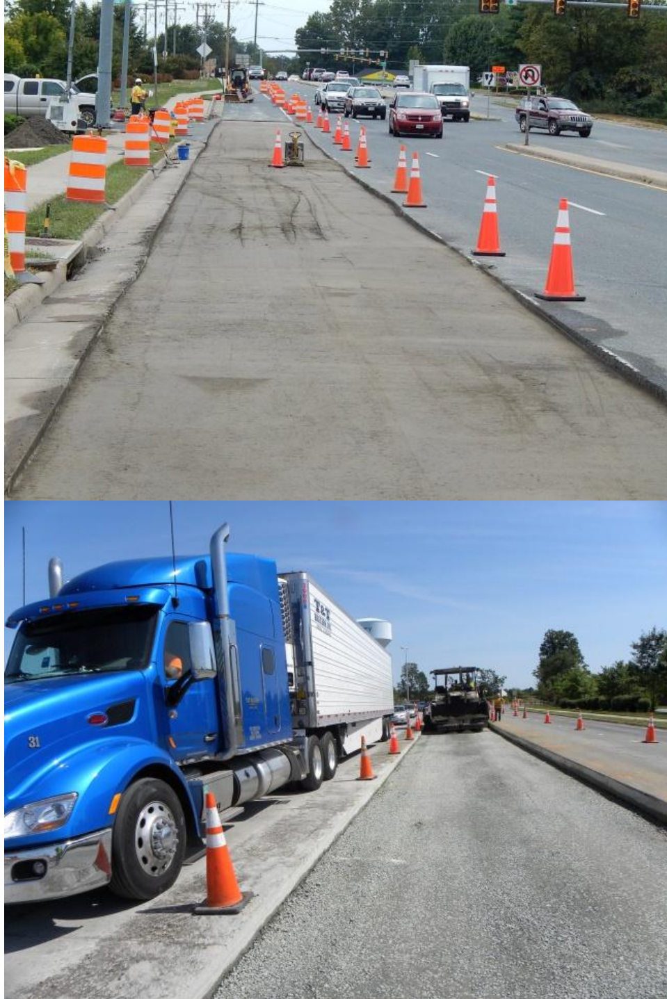
Figure 16. Photos. Traffic flow during RCC placement.
