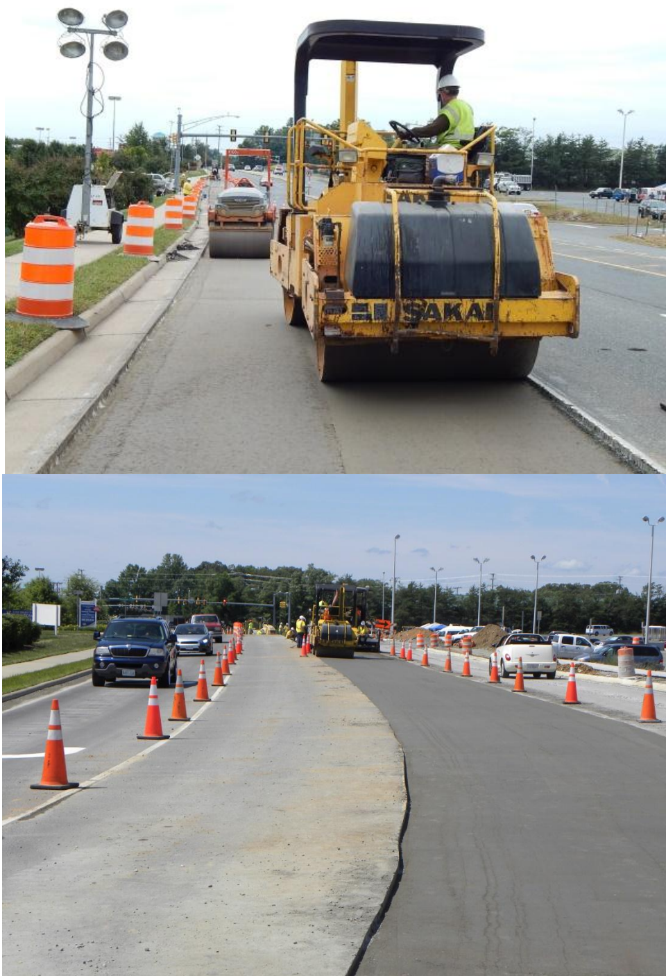
Figure 11. Photos. RCC compaction behind the paver (with rollers operated in a static mode).
