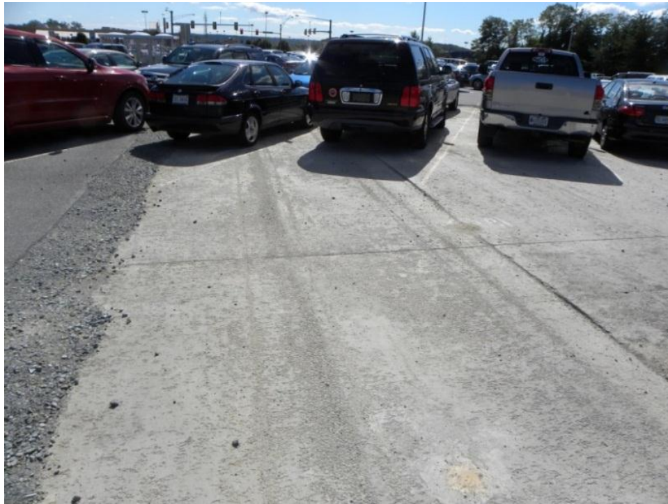
b) Completed RCC test sections
