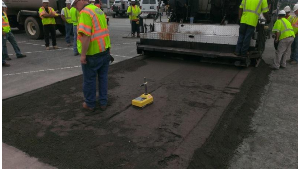
a) RCC placement at the test section
