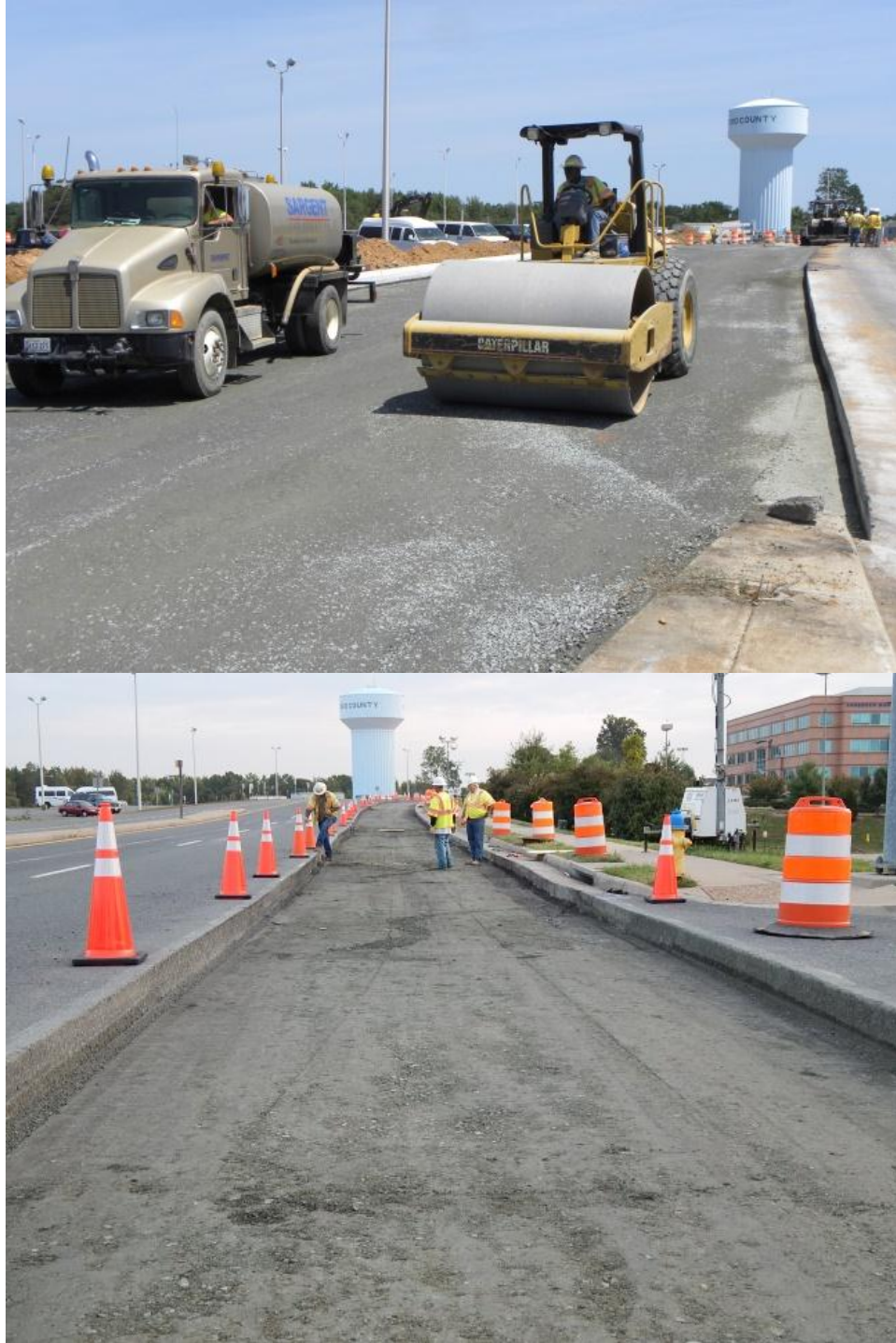
Figure 7. Photos. Base compaction and finished base just before RCC placement. Note that geogrid was used to stabilize the subgrade prior to placement of the base.
