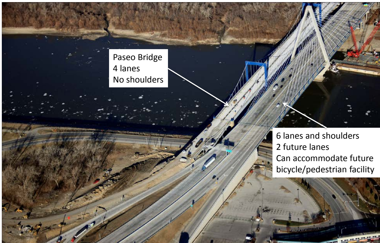
Figure 14. Six-lane Bond Bridge crossing the Missouri River—January 2011.
