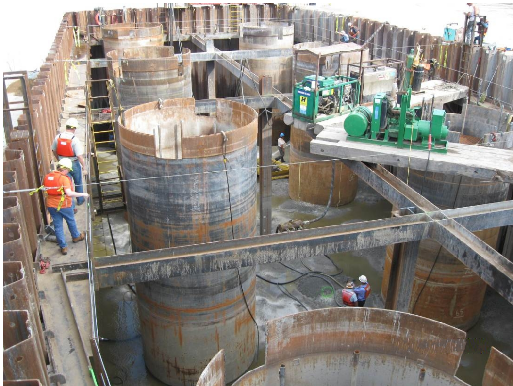
Figure 36. A dry cofferdam—October 2008.
