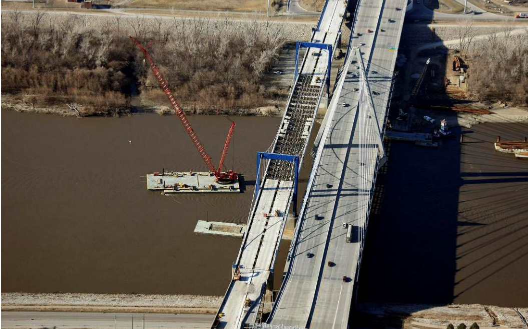
Figure 61. Removal and recycling of the old Paseo Bridge—March 2011.
