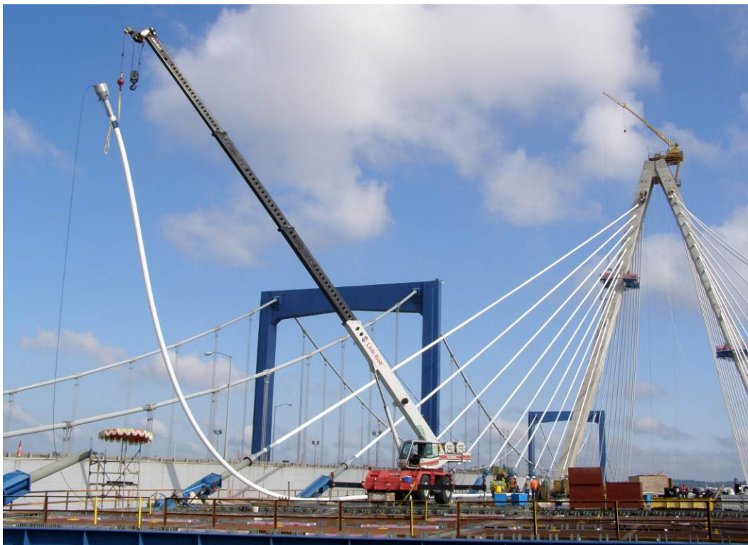
Figure 56. Final stay cable installed—August 2010.
