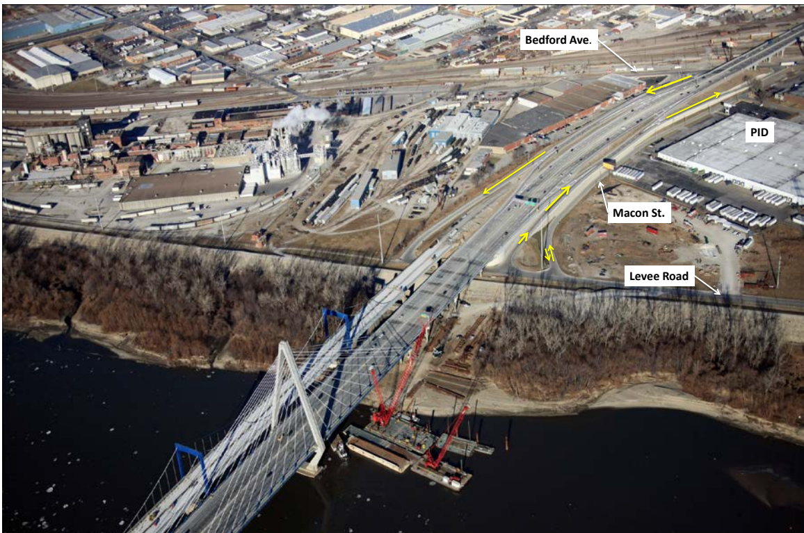
Figure 16. Levee Road crossing—January 2011.
