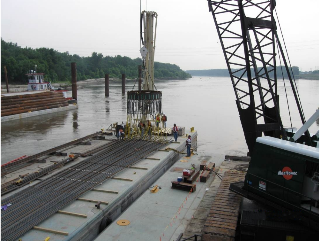
Figure 29. Aligning the wagon wheel for the rebar lift—August 2008.
