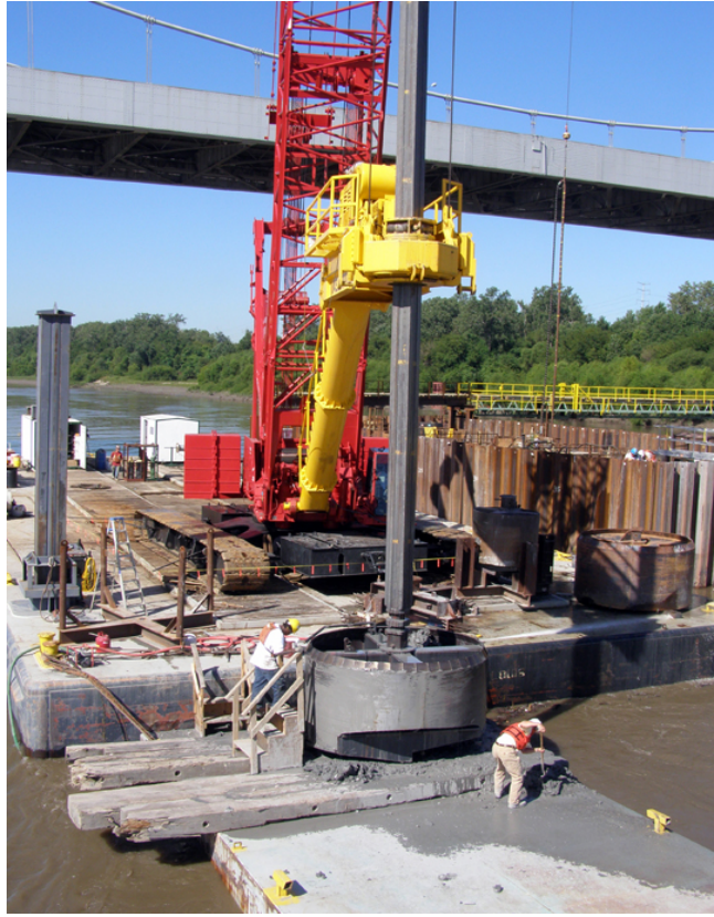
Figure 27. Augering the drilled shafts—August 2008.
