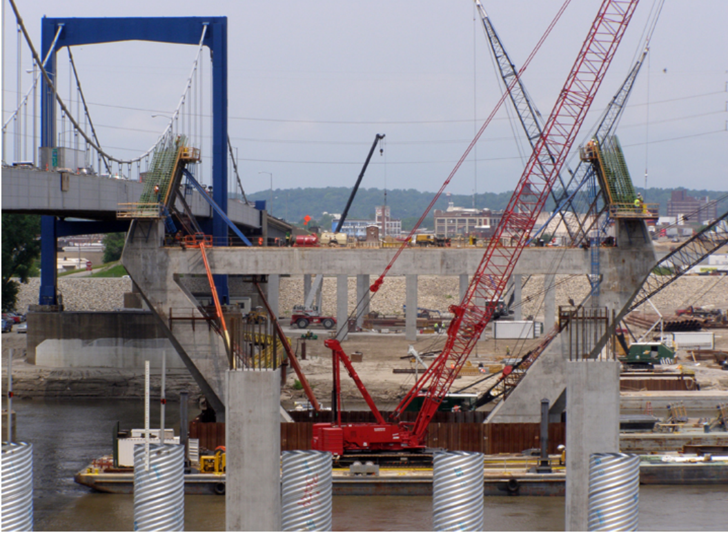
Figure 45. A third of the way to the top in constructing pylon above the roadway strut—May 2009.
