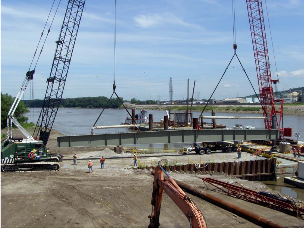
Figure 47. Two cranes moving floor beam from truck to barge—August 2009.
