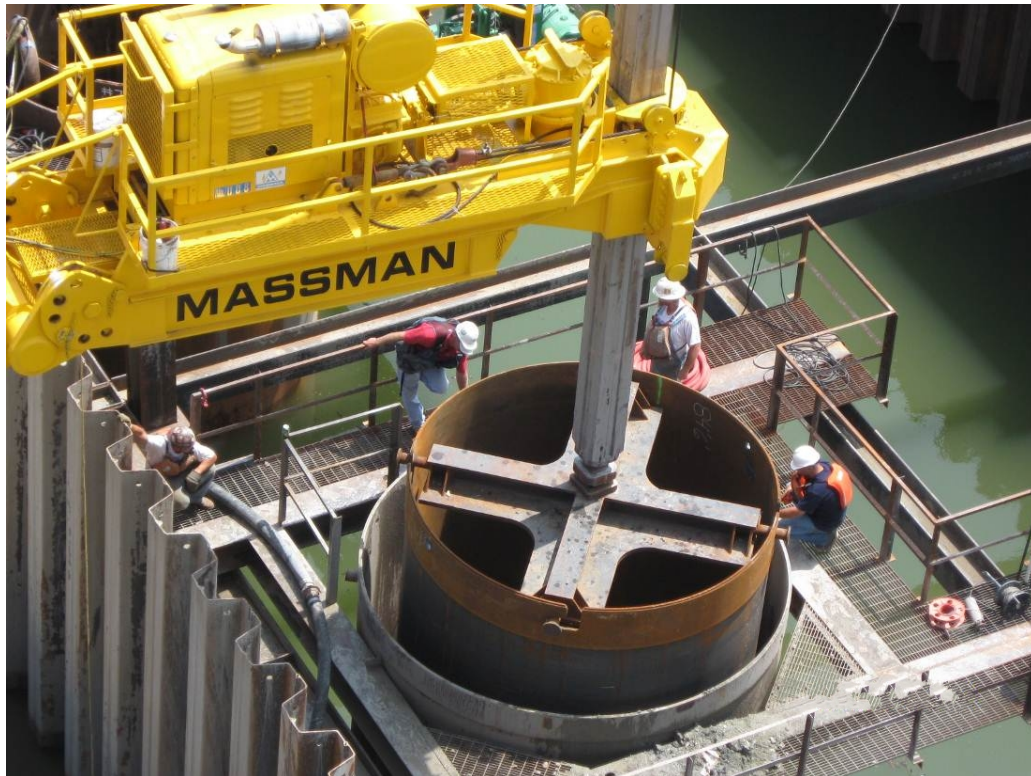
Figure 26. Final alignment of the permanent casing—August 2008.
