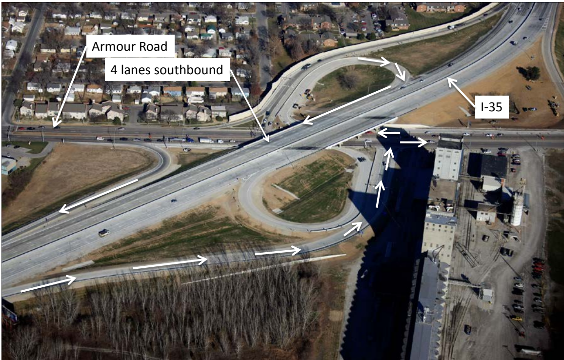
Figure 20. Armour Road interchange—January 2011.
