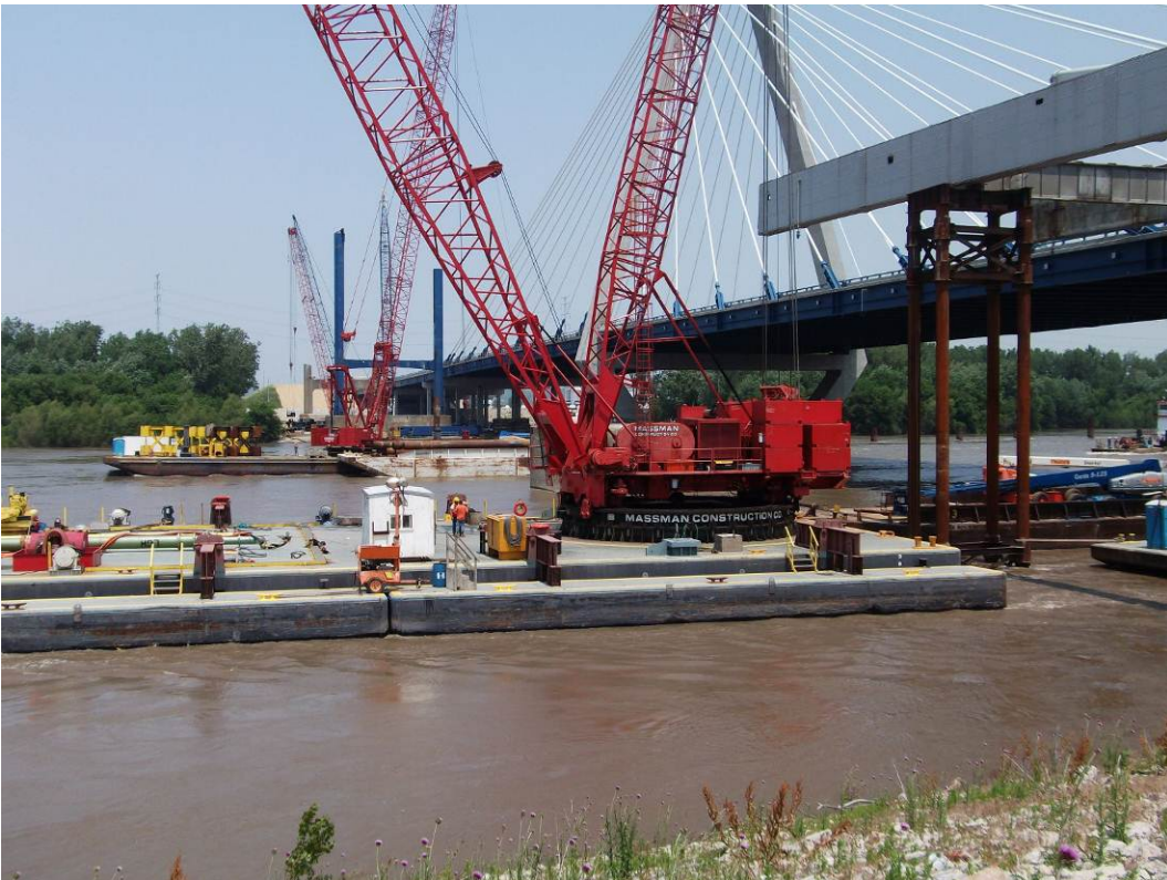
Figure 62. Removal of Paseo Bridge nearing completion—June 2011.
