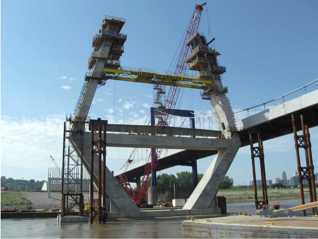
Figure 49. Placing the first floor beam onto the roadway strut—August 2009.
