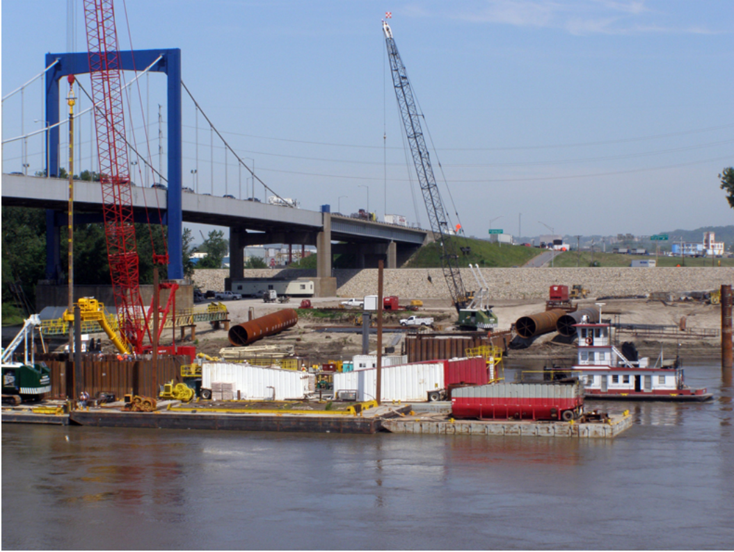
Figure 23. Beginning cofferdam work—August 2008.
