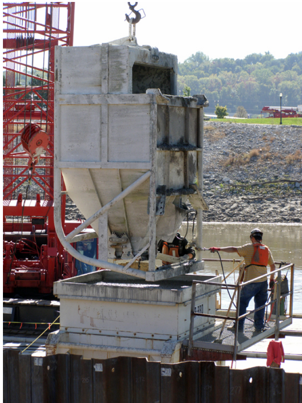
Figure 35. Pouring the concrete into the drilled shaft—October 2008.
