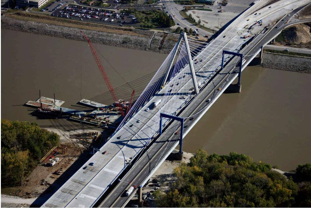
Figure 59. Christopher S. Bond Missouri River bridge—November 2010.
