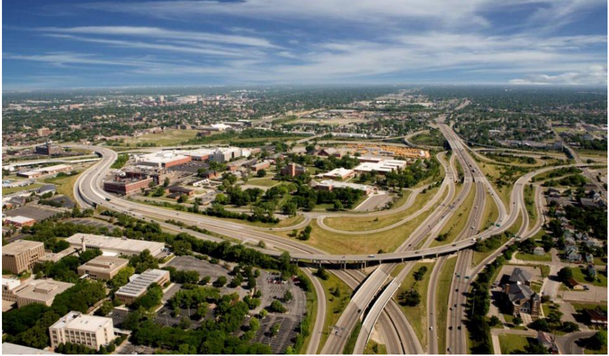
Figure 3. Photo. I-71/I-670 interchange before construction.
