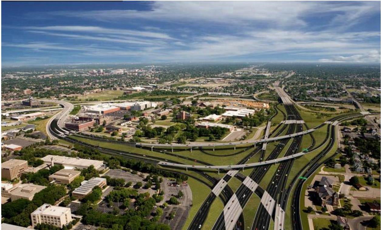
Figure 4. Photo. I-71/I-670 interchange after construction.
