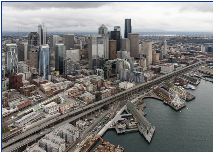
The photo above is an aerial view of the Alaskan Way Viaduct prior to demolition. (Source: Washington State Department of Transportation).
