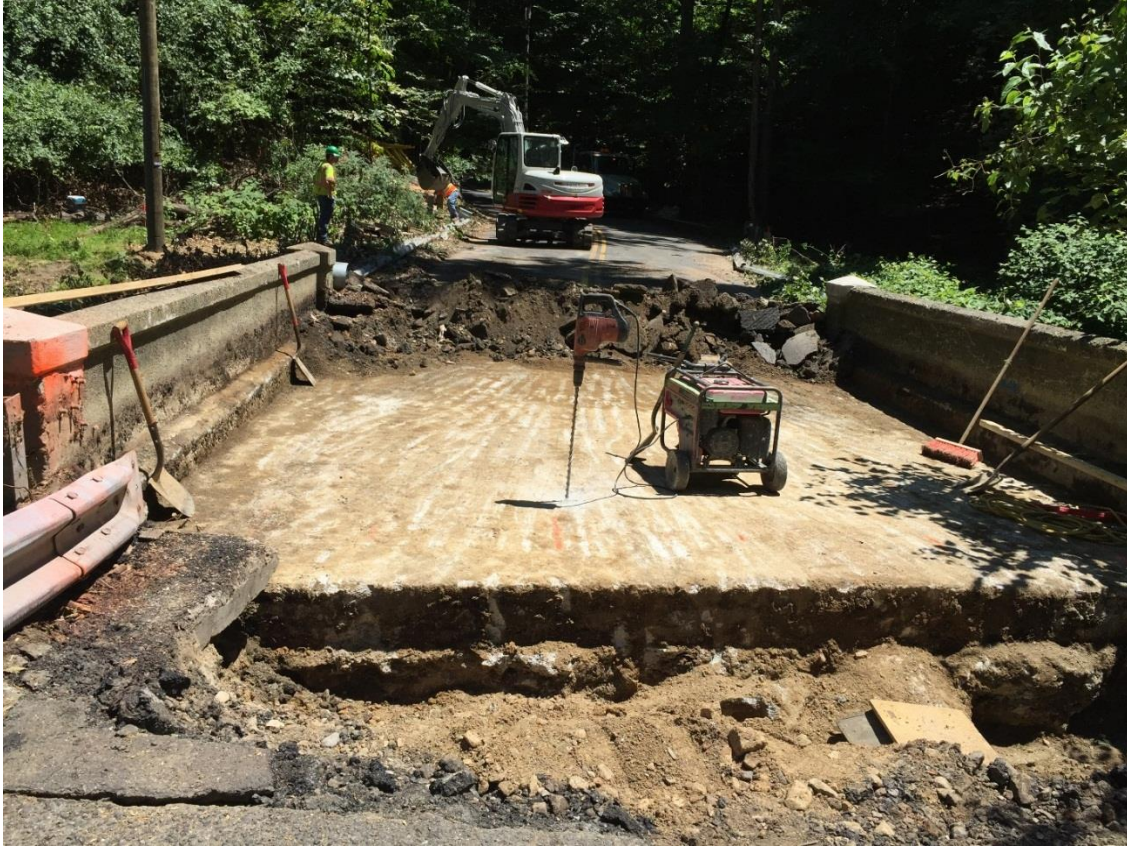
Figure 9. Photo. Demolition of existing bridge.
