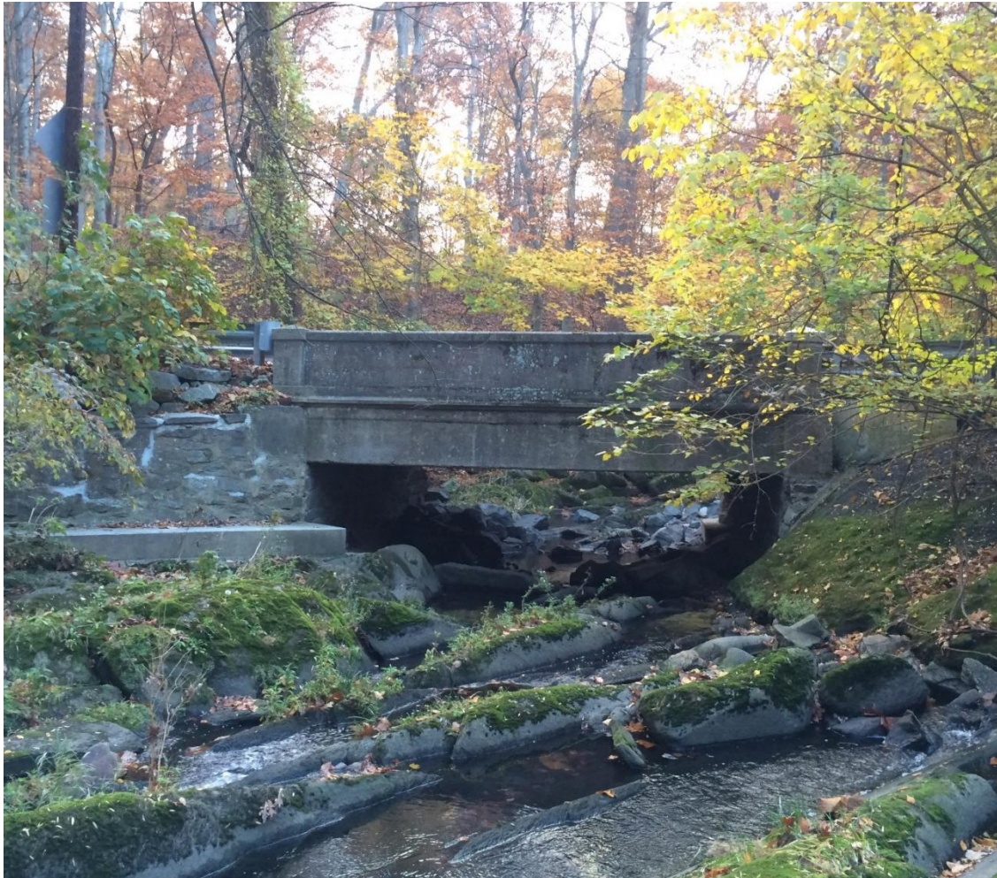
Figure 4. Photo. North face of existing bridge (courtesy: DDOT).
