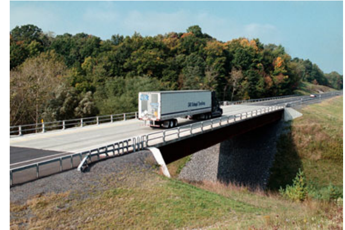
Photo Courtesy of FHWA
