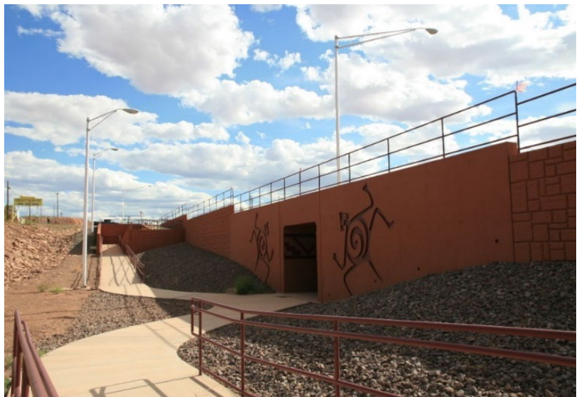
Figure 6: Undercrossing after construction. (Image courtesy of Arizona Department of Transportation)
