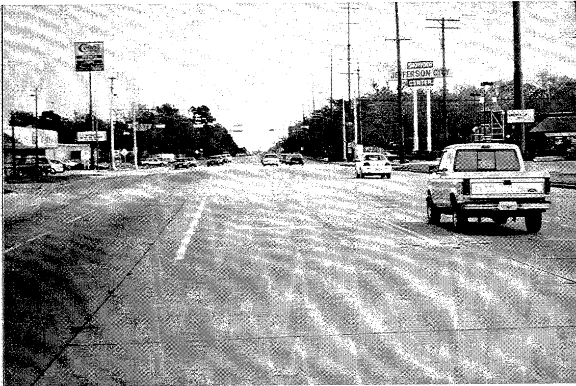
Figure 16. Southbound Twin Cities Highway at 33 rd Street
