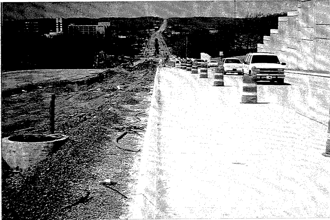
Figure 33. Westbound 71 st Street West of Harvard Avenue
