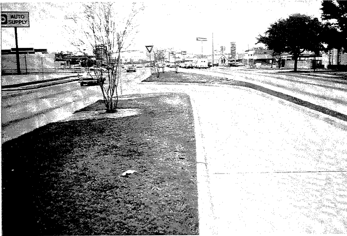
Figure 2. Southbound South Post Oak Road Illustrating Channelized Median
