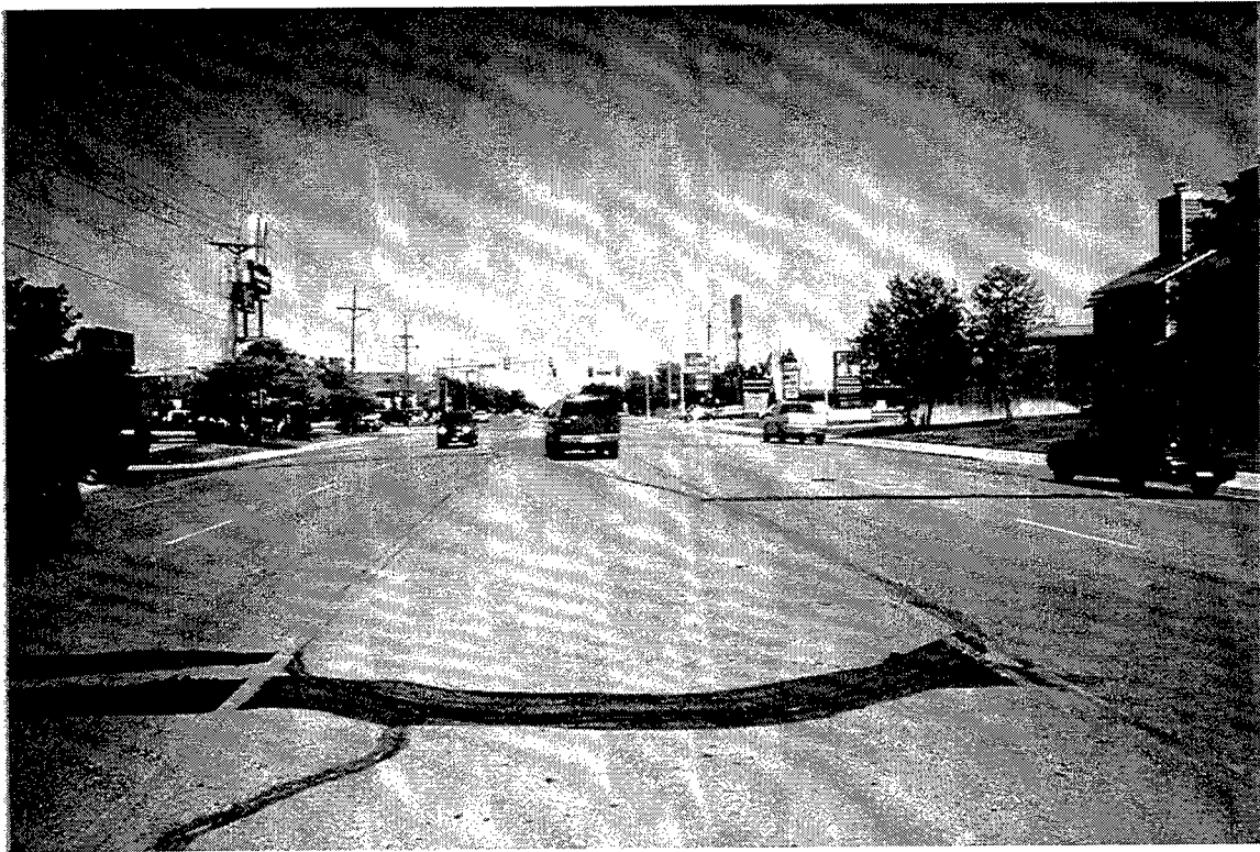
Figure 36. Westbound 34 th Street Just East of Coulter Street
