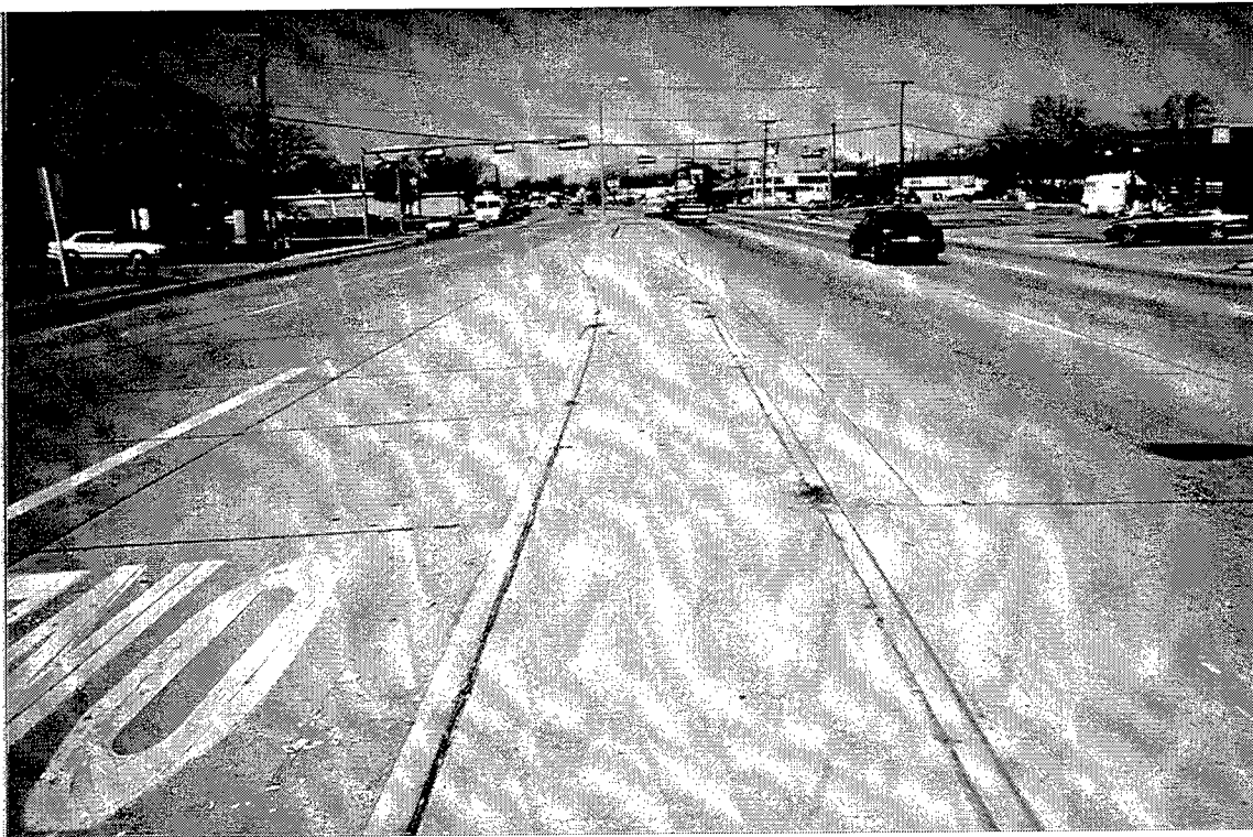
Figure 19. Westbound University Drive Near Church Street
