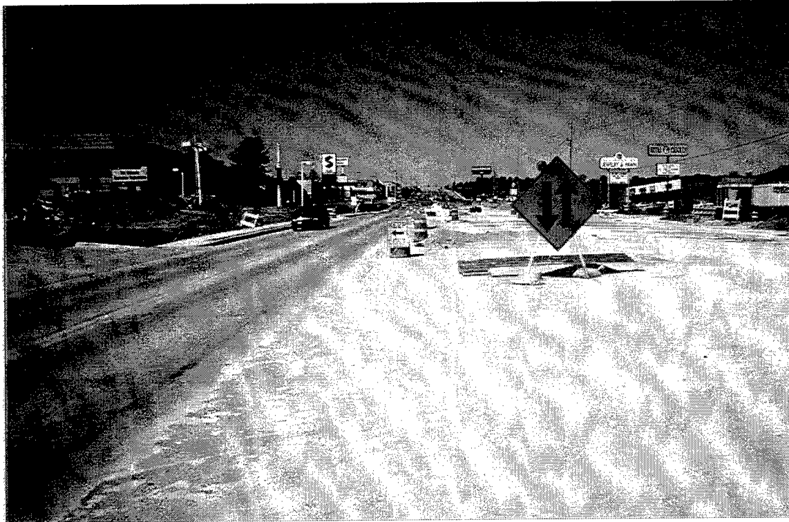
Figure 32. Westbound 71 st Street at 69 th Avenue
