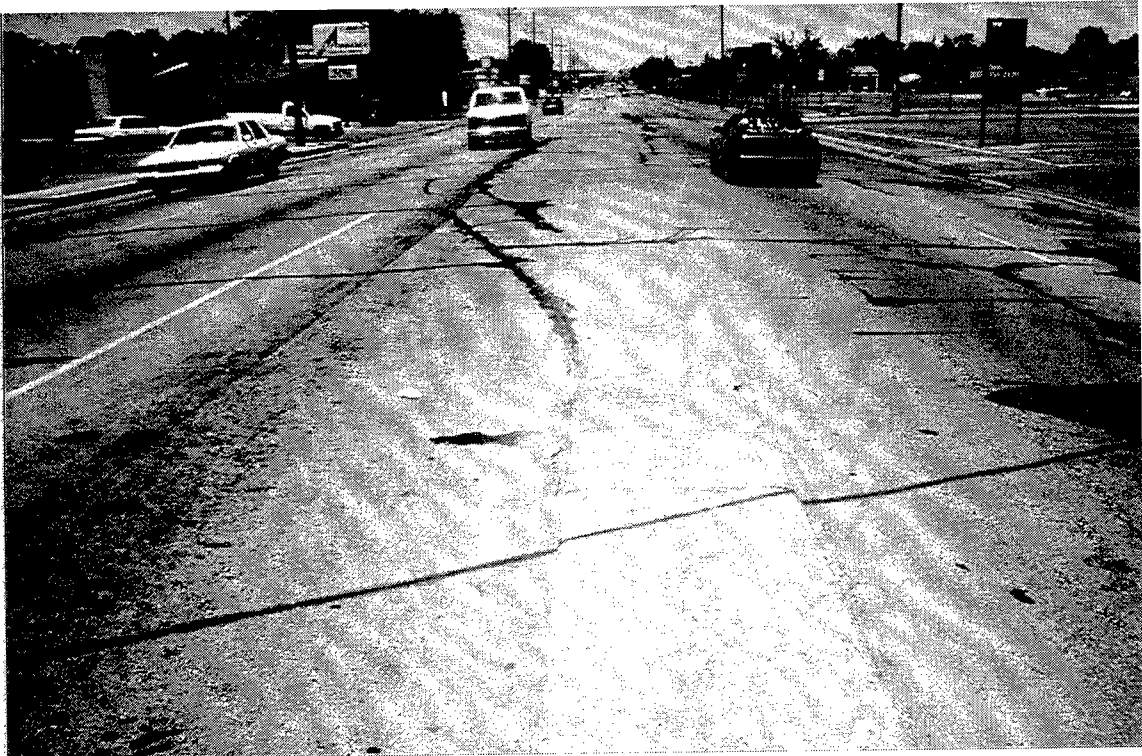
Figure 35. Northbound Georgia Street North of 34 th Street
