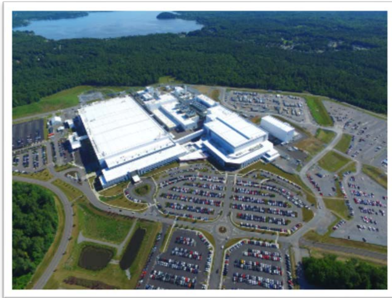
Figure 10: GlobalFoundries Fab 8 Plant, Malta, NY
