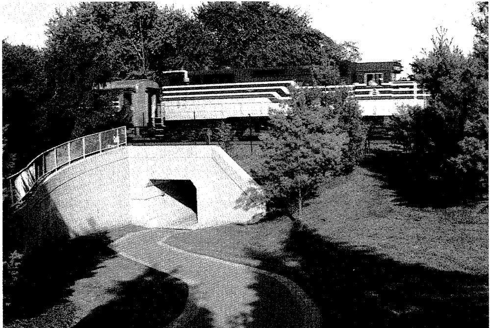
Grade-separated crossings can benefit all users.
