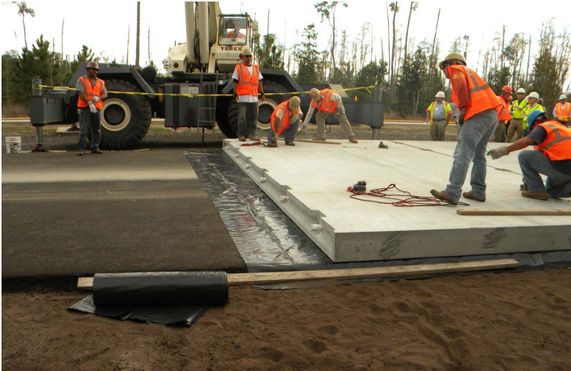
Figure 4. Photo. Panel placement.
