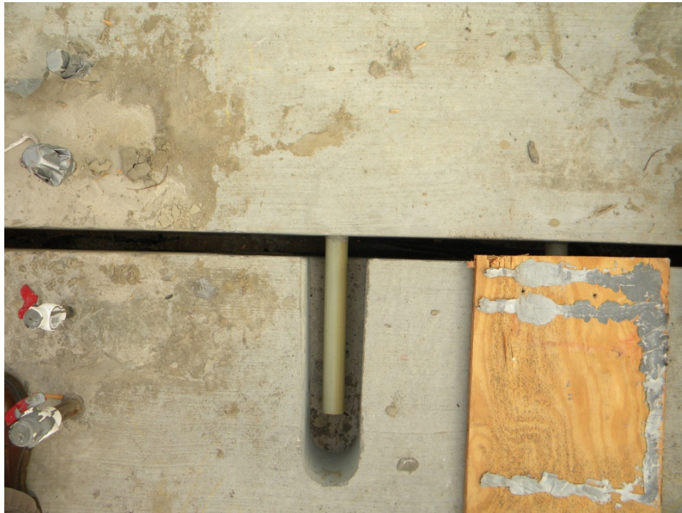
Figure 12. Photo. Dowel pocket.
