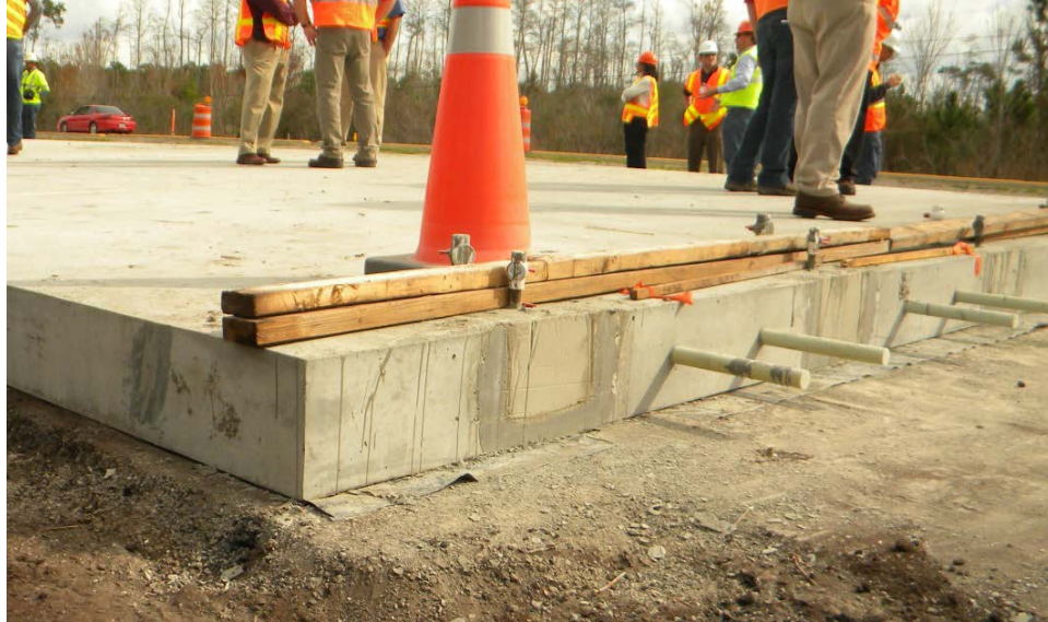
Figure 11. Photo. End panel with exposed dowel bars.
