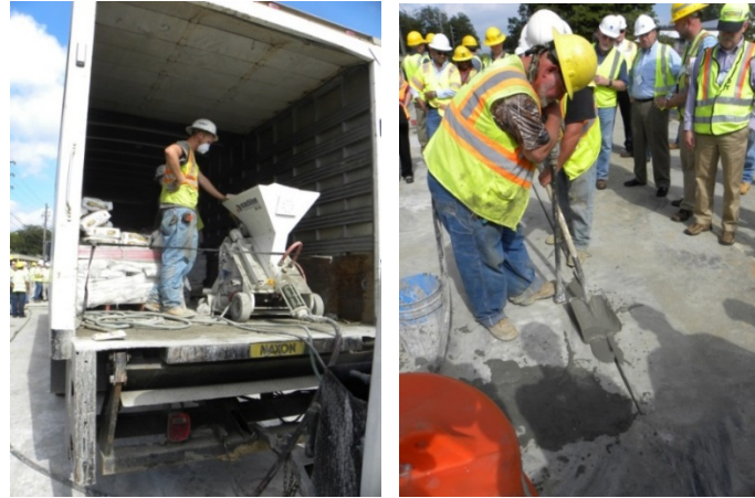
Figure 38. Photo. Dowel slot grouting operation.
