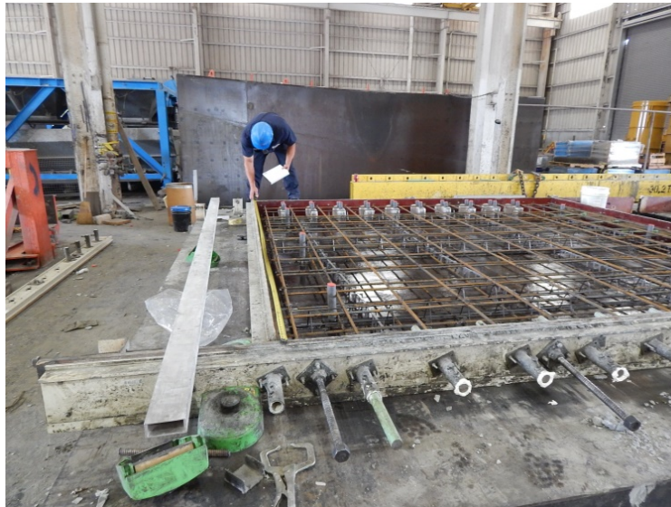
Figure 22. Photo. Formwork being checked for tolerances.
