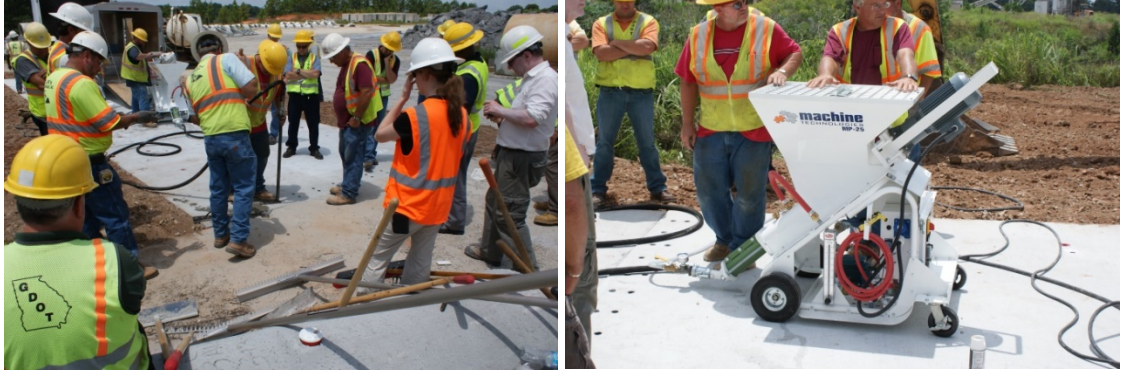
Figure 18. Photos. Slot grouting and grout pump.
