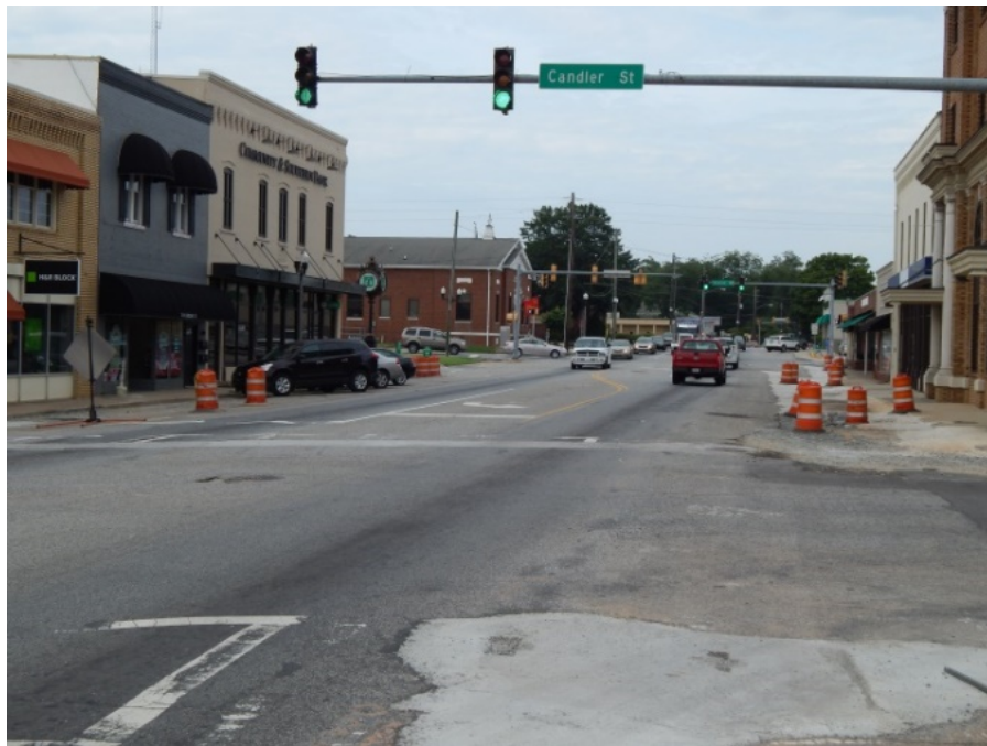
Figure 5. Photo. View of Broad Street and typical rutting (as of August 2013).
