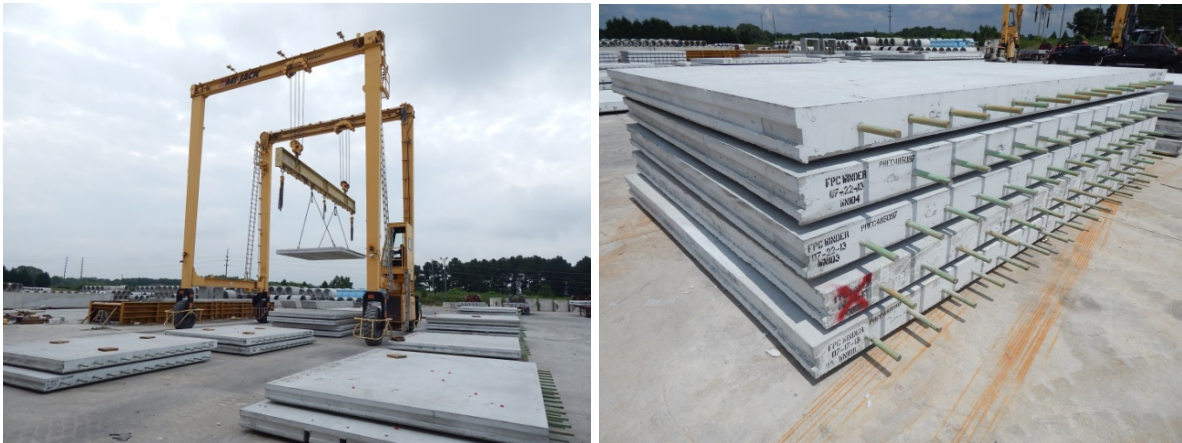
Figure 28. Photos. Panels moved within the precast plant storage area using a gantry crane.
