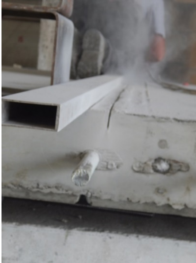
Figure 27. Photo. Longitudinal sawcut in a two-lane wide panel (also showing dowel bar located at the sawed centerline).
