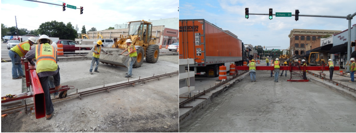
Figure 34. Photos. Bedding material placement and compaction.
