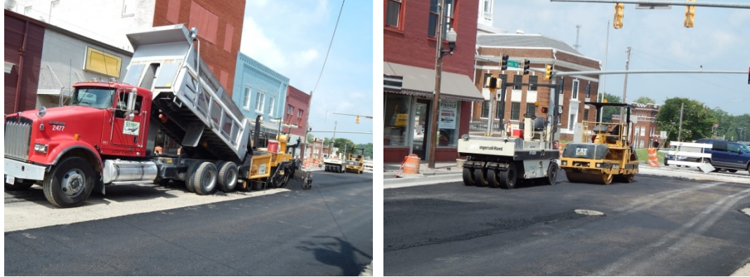
Figure 40. Photos. Resurfacing of an intersecting street.
