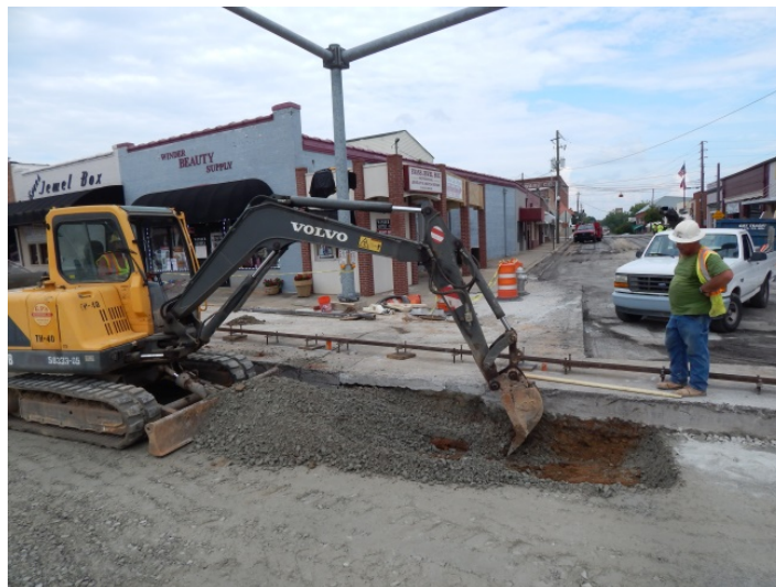
Figure 31. Photo. Removing the softer subgrade material.
