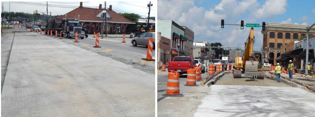
Figure 14. Photos. Lane closure and two-way traffic operation.
