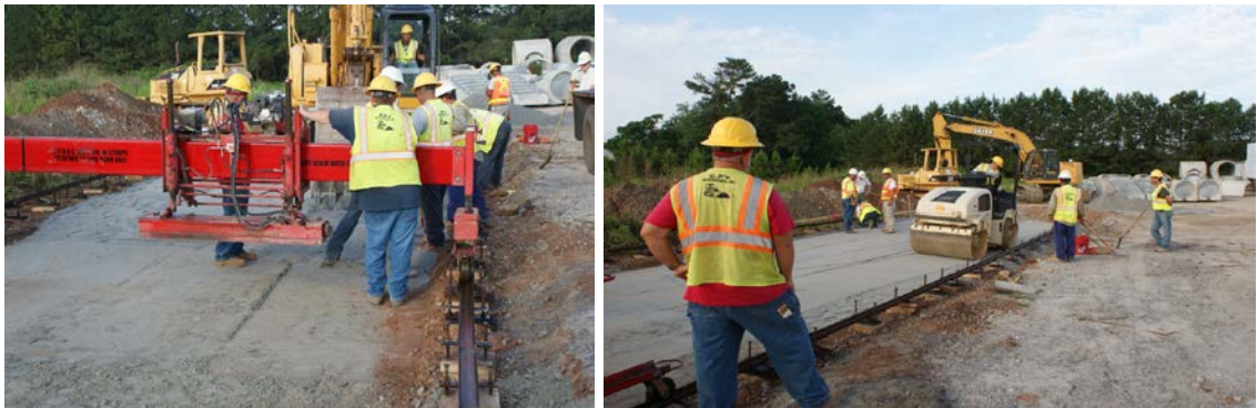
Figure 15. Photos. Base grading and compaction.
