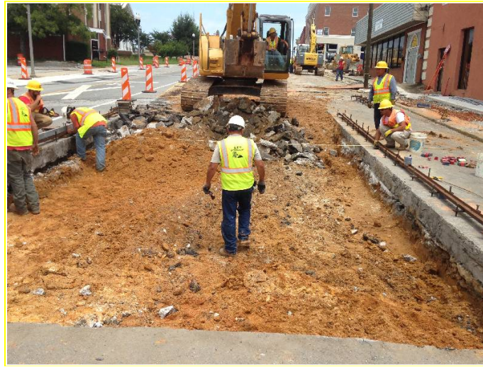
Figure 30. Photo. Existing composite pavement removal.
