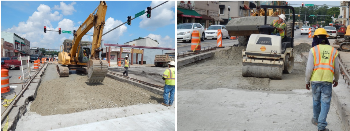
Figure 32. Photos. Base material placement and compaction.
