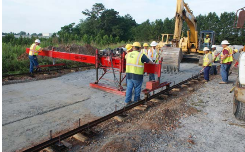
Figure 16. Photo. Bedding layer grading.
