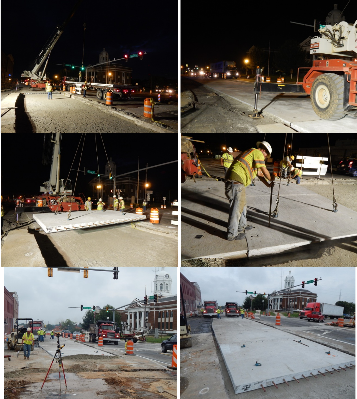
Figure 36. Photos. Typical views of panel installation along Broad Street.
