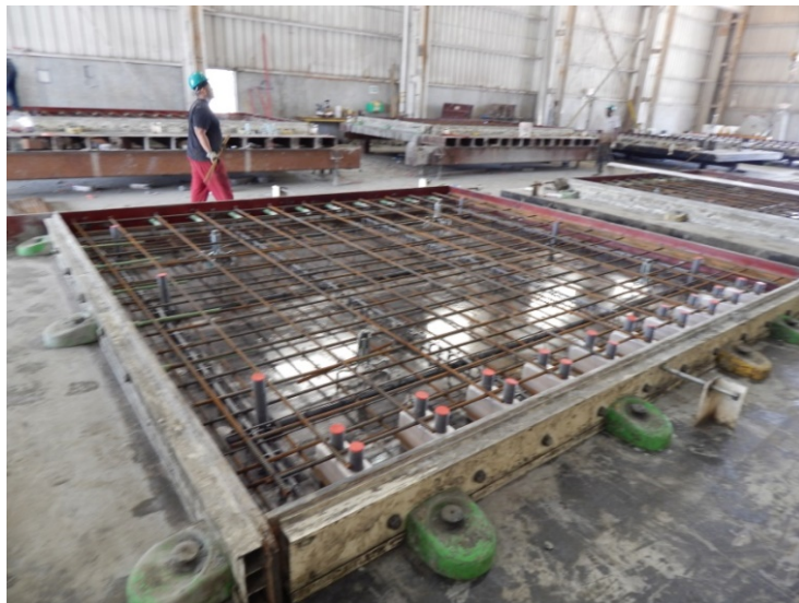
Figure 19. Photo. Panel formwork ready for concrete placement.
