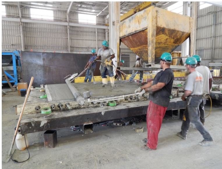
Figure 26. Photo. Concrete surface finishing using a roller screed.
