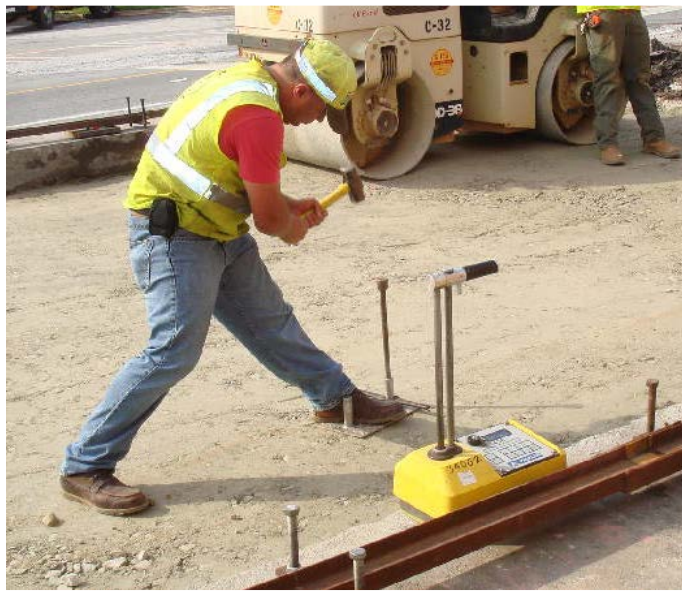
Figure 33. Photo. Granular base compaction testing using a nuclear gage.
