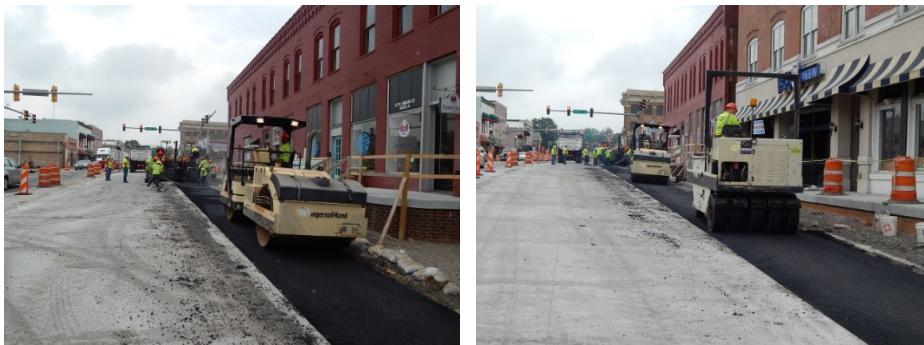
Figure 39. Photos. Parking lane construction using asphalt concrete.
