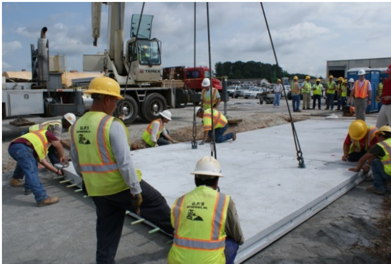
Figure 17. Photo. Panel installation over the prepared base and bedding layer.
