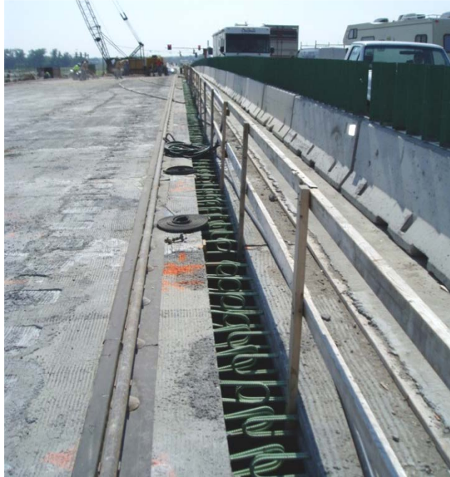
Figure 7. Longitudinal panel connection.
