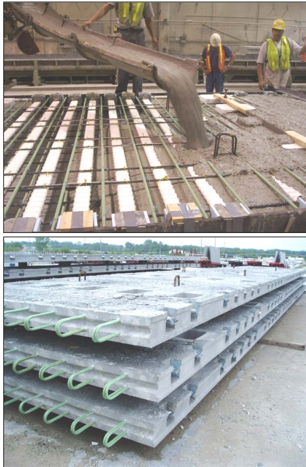
Figure 5. Self-consolidating concrete being placed and three panels ready for delivery.
