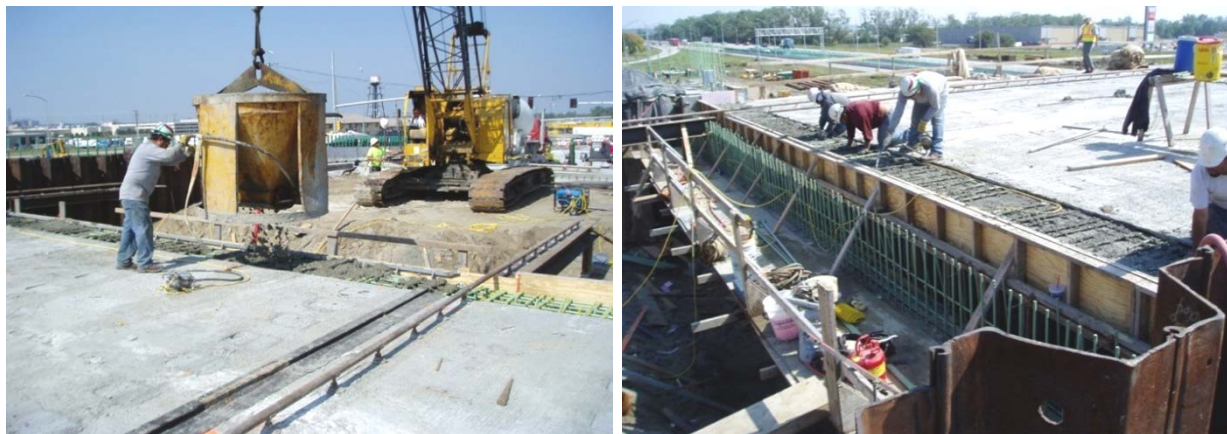
Figure 11. Casting HPC at the bridge abutments.
