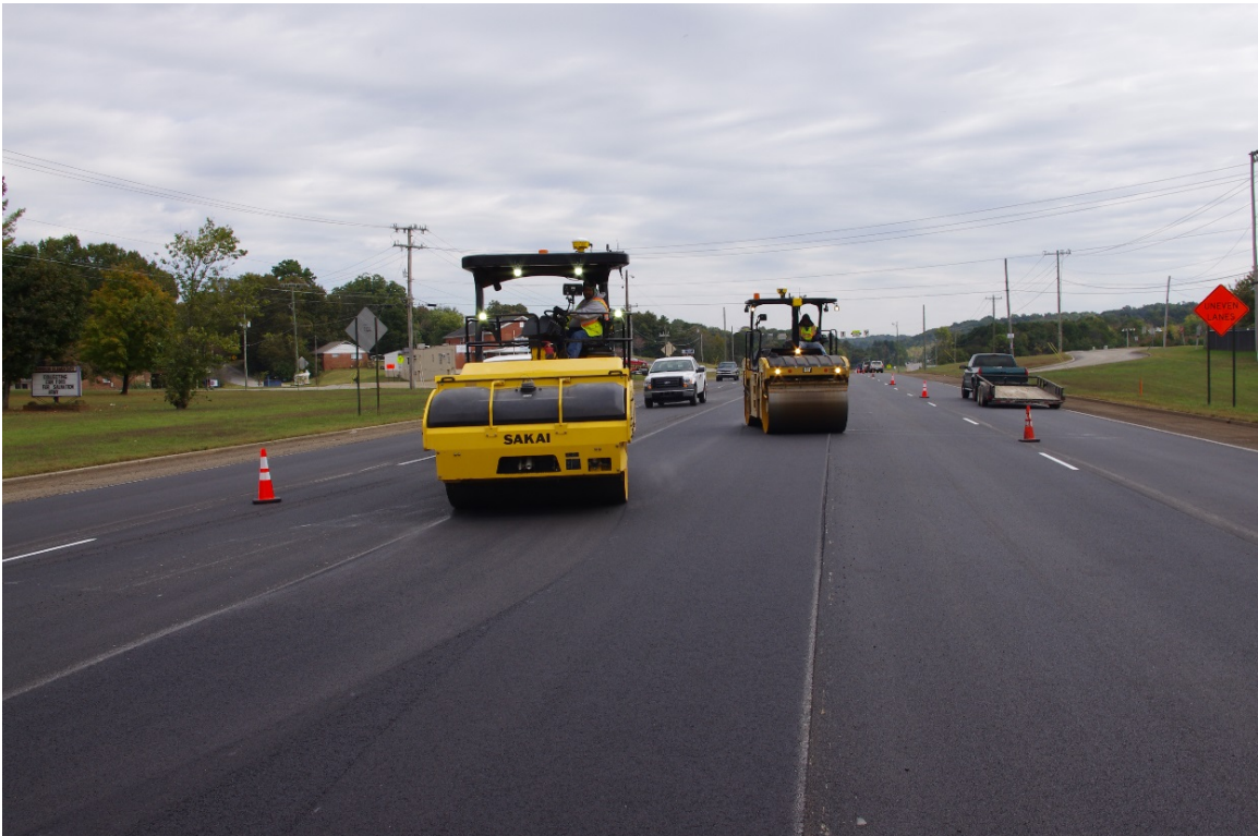
Figure 30. Photo. IC roller in operation. (courtesy: TDOT)
