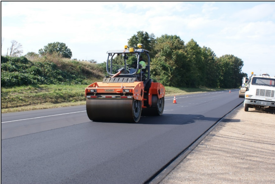
Figure 22. Photo. IC-equipped compaction roller.
