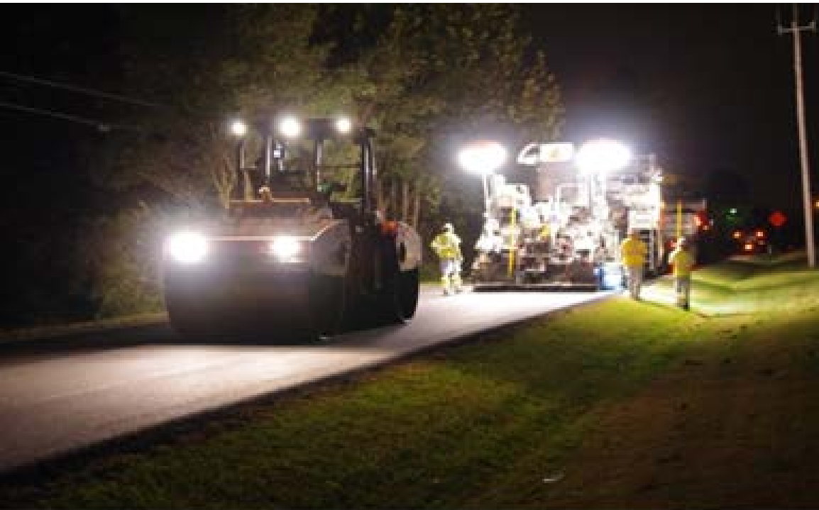
Figure 14. Photo. IC roller in operation. (courtesy: TDOT)
