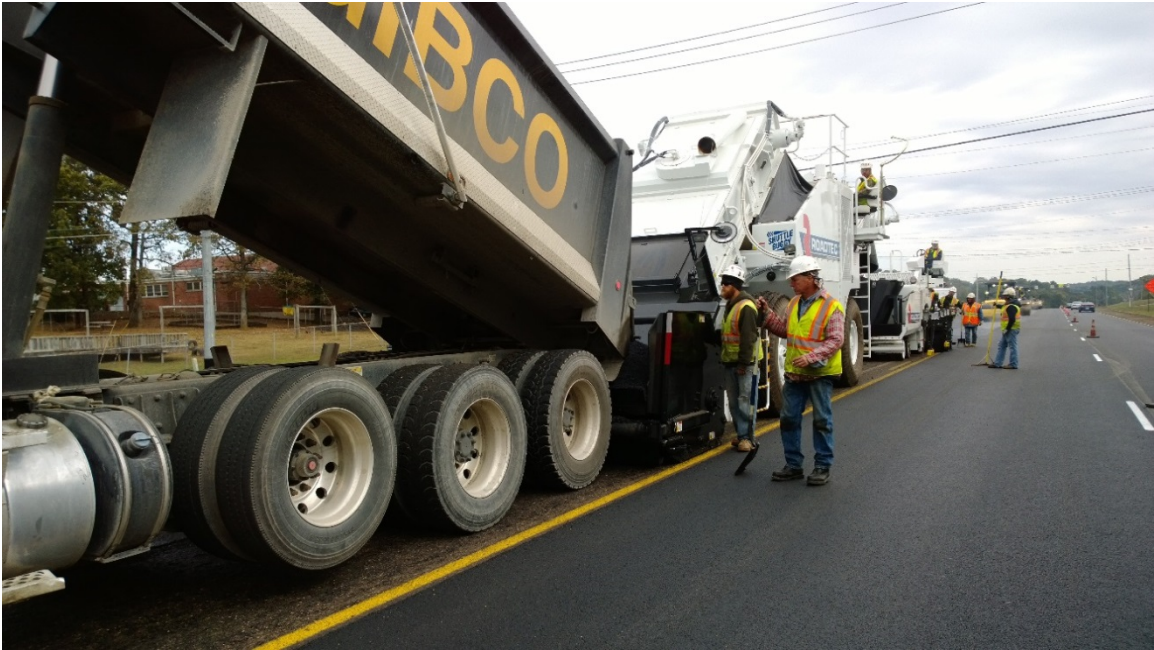
Figure 29. Photo. AC mat placement. (courtesy: TDOT)
