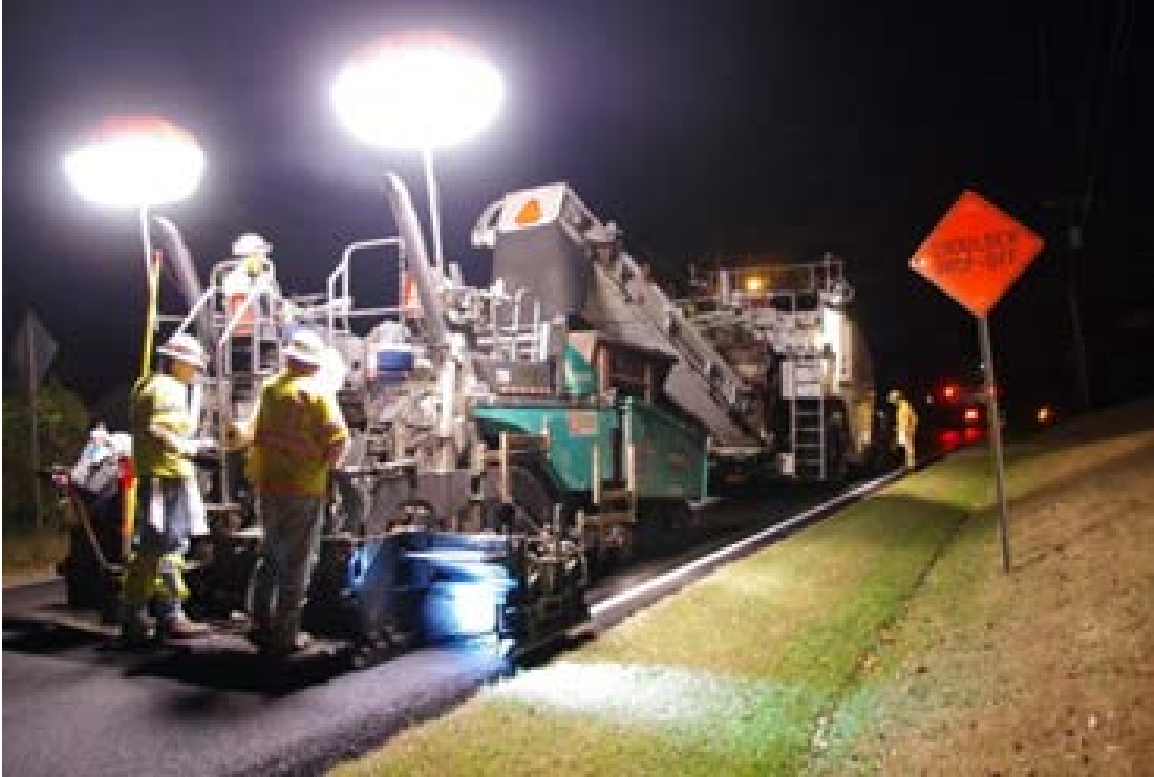
Figure 13. Photo. AC mat placement (courtesy: TDOT)
