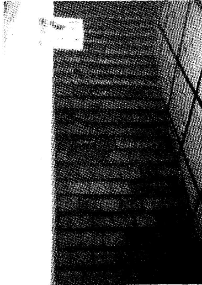
b. The downstream slope after Test ER-2.
