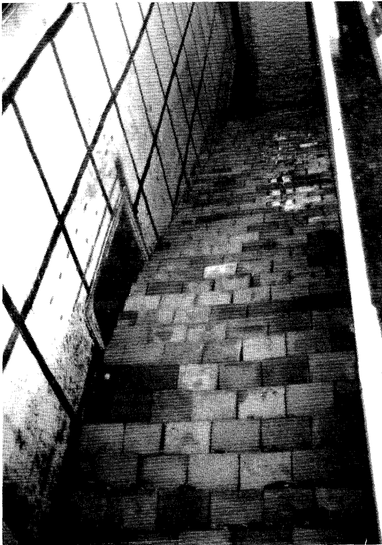
a. Looking downstream after Test ER-2. Note loose gravel remaining in the lee of the blocks
