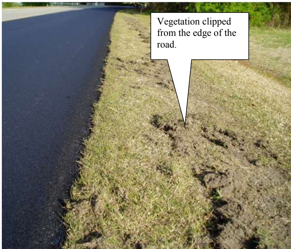
Figure 8. Vegetation removed by clipping the edge of the existing pavement.
