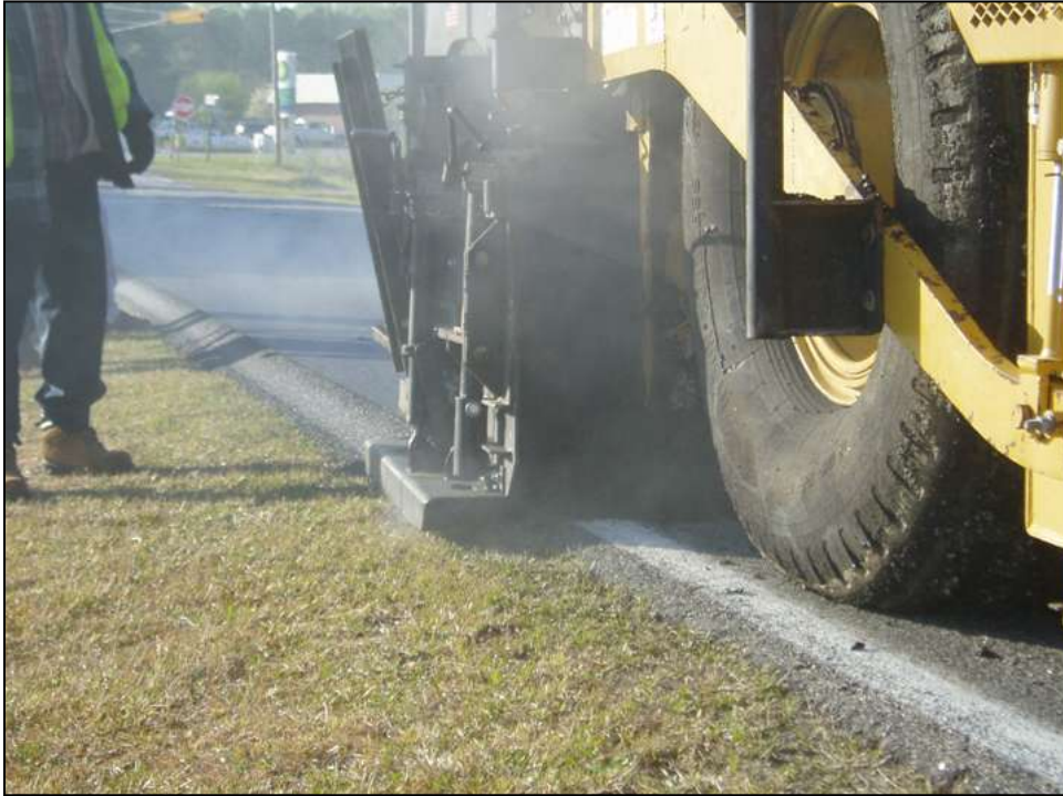
Figure 11. Angled approach of the Carlson device.
