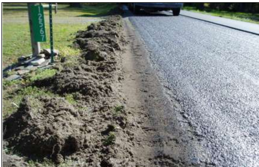
Figure 10. Soil/vegetation piled up from edge preparation work.
