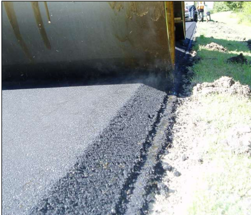
Figure 13. Slope face produced by the Troxler device.
