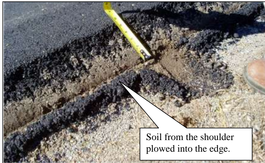
Figure 9. Example of the Safety Edge SM device plowing up soil into the Safety Edge SM .
