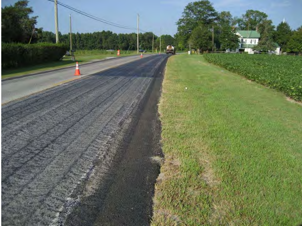
Figure 6. General view of the roadway and right-of-way.
