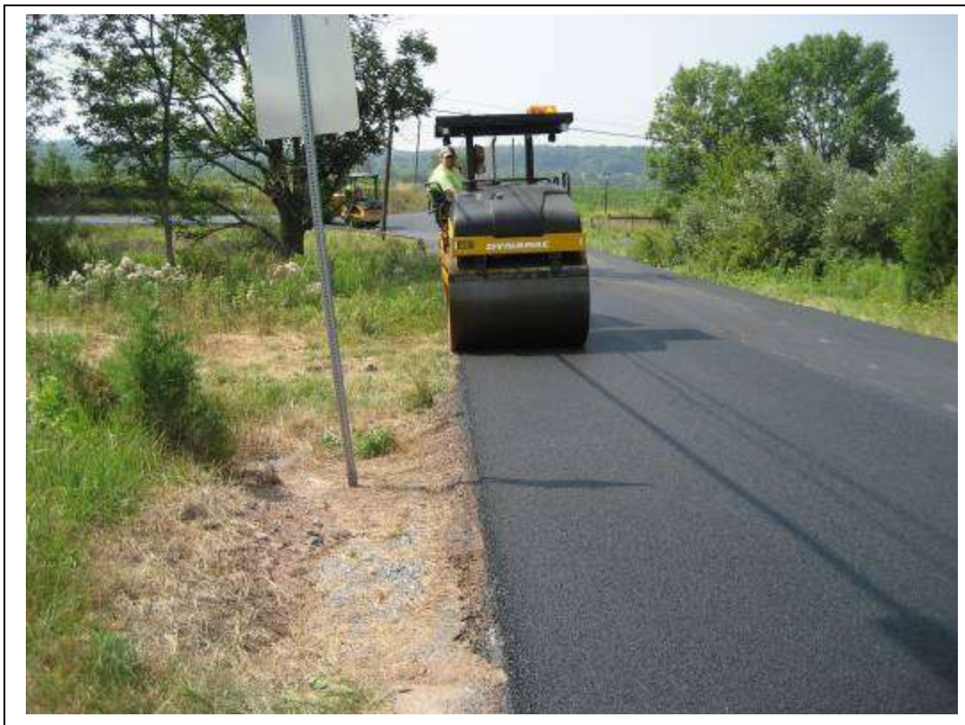
Figure 22. Vibratory steel wheel roller used in the breakdown position shown compacting the Safety Edge SM – first pass overhung the edge about 4 inches.
