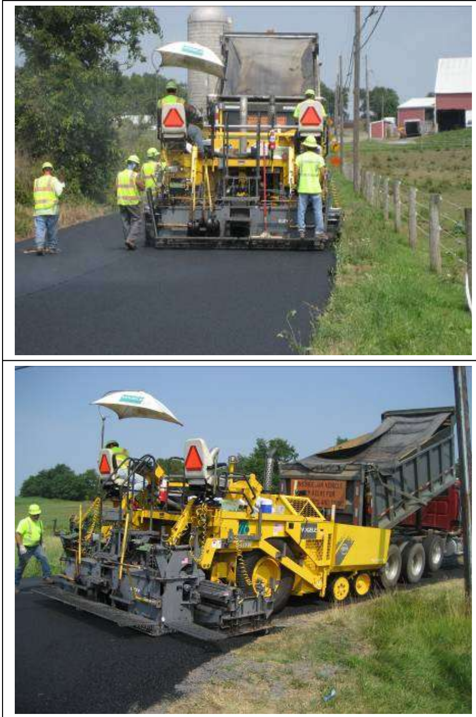
Figure 16. Photo illustrating the edge condition of the pavement.
