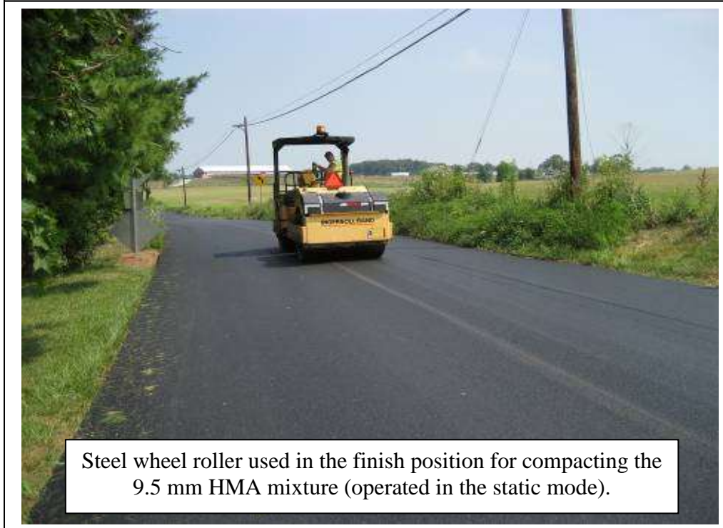
Figure 21. Two steel wheel rollers used to compact the 9.5 mm HMA mix.
