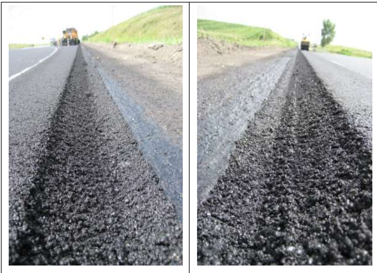
Figure 16. Typical surface texture and slope of the Safety Edge SM sections.
