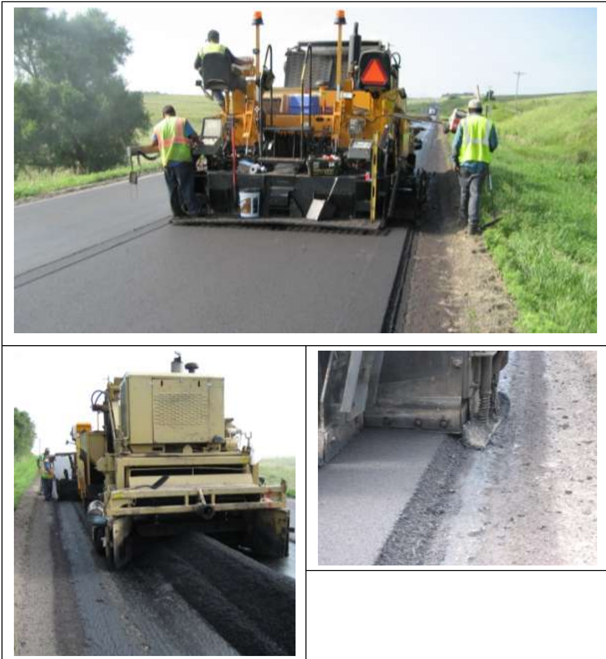
Figure 14. Equipment used to place the HMA overlay.
