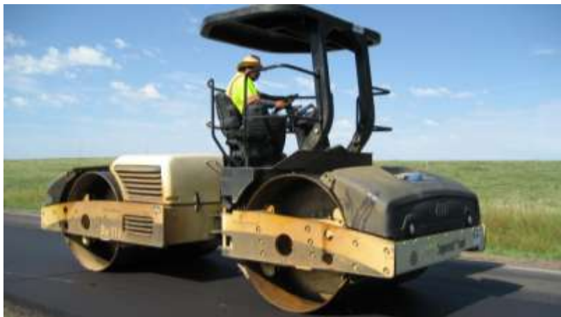
Figure 17. Rollers used for compacting the 12.5 mm HMA overlay mixture.
