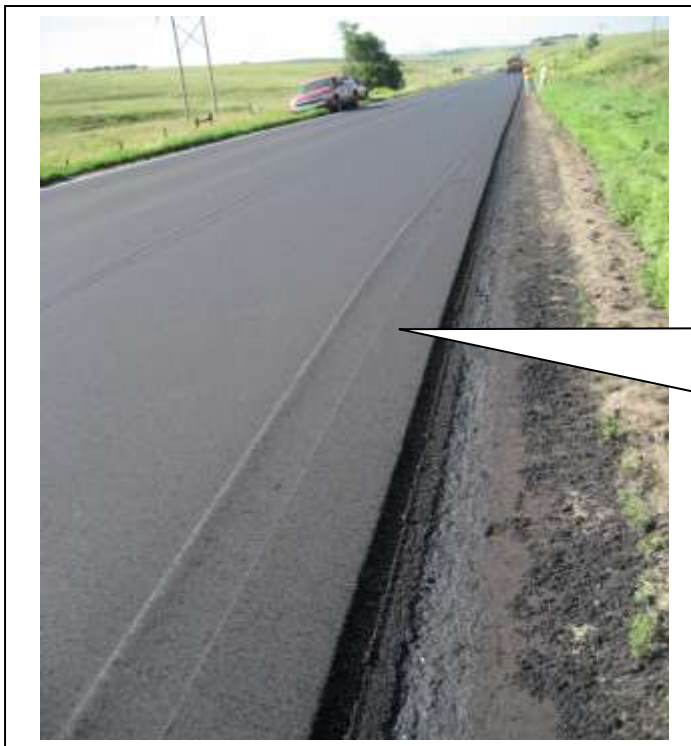
Figure 20. Rolling the unconfined edge with the vibratory steel wheel roller.
