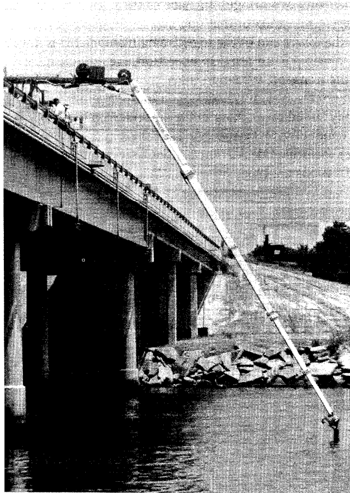
Figure 2. Bridge Inspector in operation.
