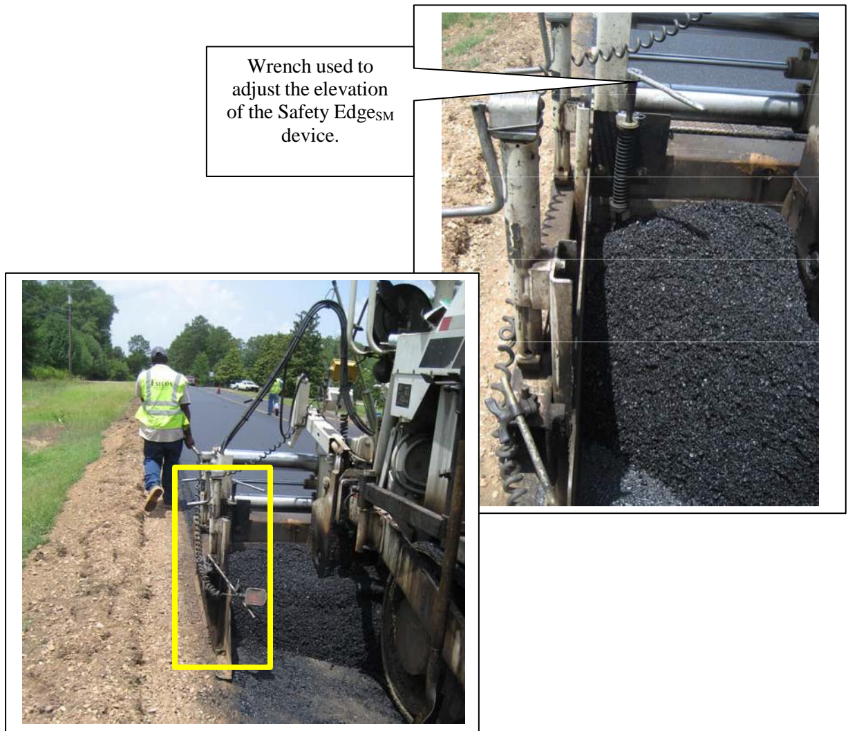
Figure 12. Safety Edges SM adjustment for raising and lowering the device.
