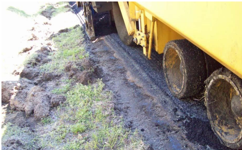
Figure 9. Paver positioned to align the Safety Edge SM break point over the existing pavement.
