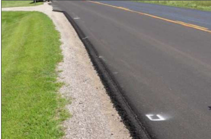
Figure 15. Typical view showing the base and intermediate course with Safety Edge SM and granular shoulder material. Image taken east of Sully.
