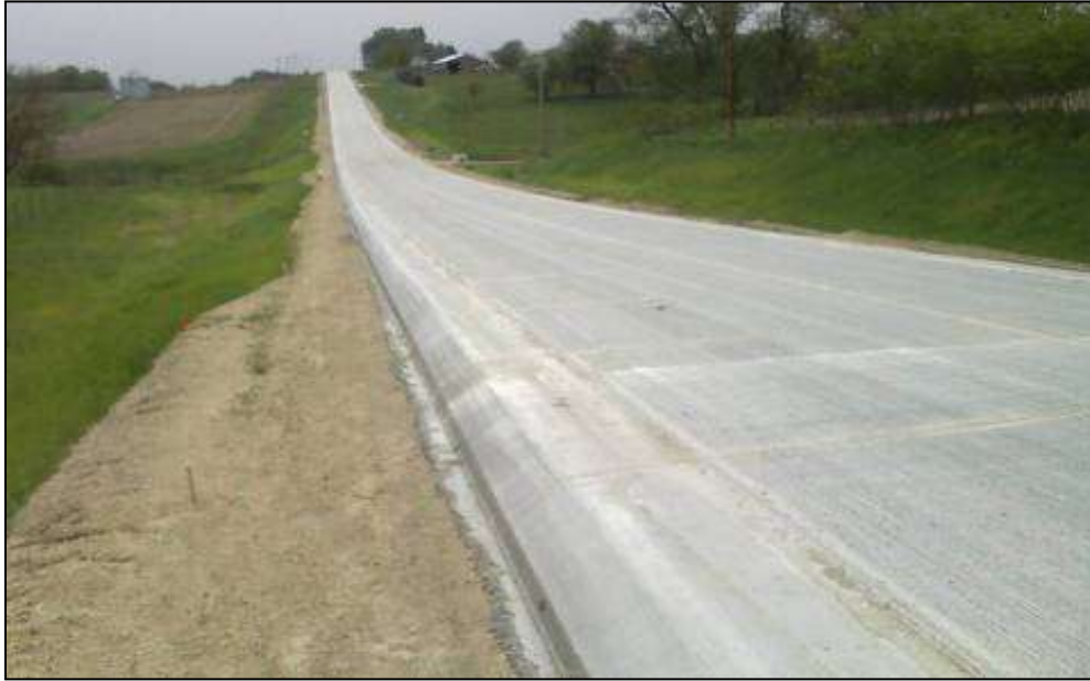
Figure 2. General view of the project showing the Safety Edge SM .
