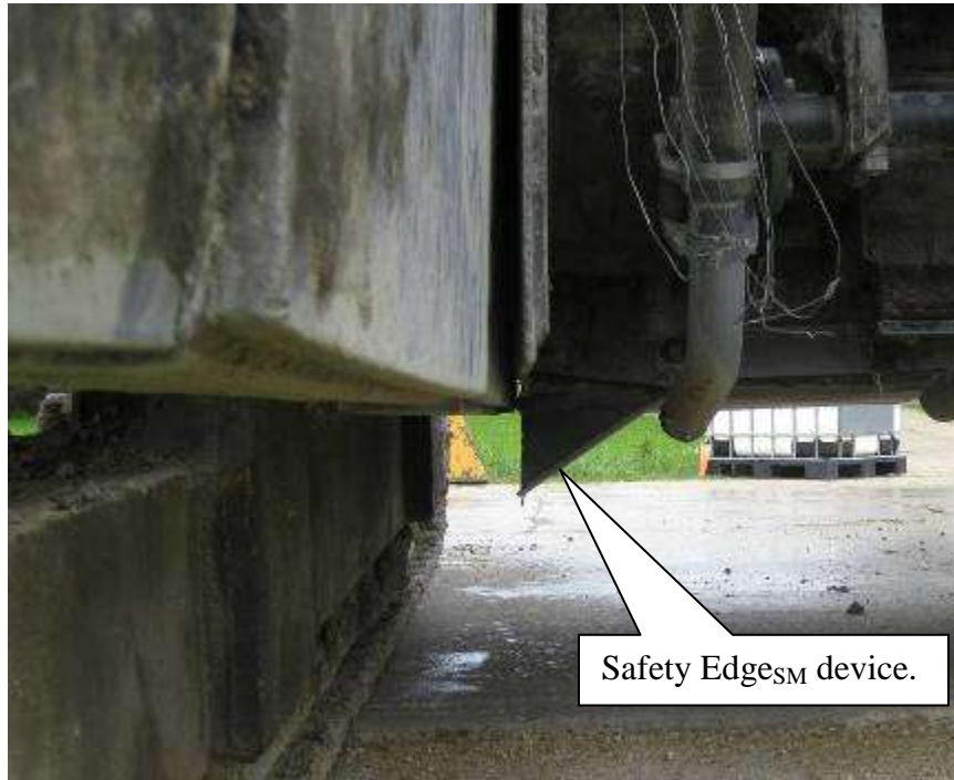
Figure 14. View of the Safety Edge SM device from front of paver.
