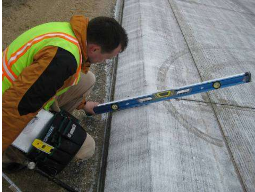
Figure 4. Measuring the slope and flatness of the Safety Edges SM .
