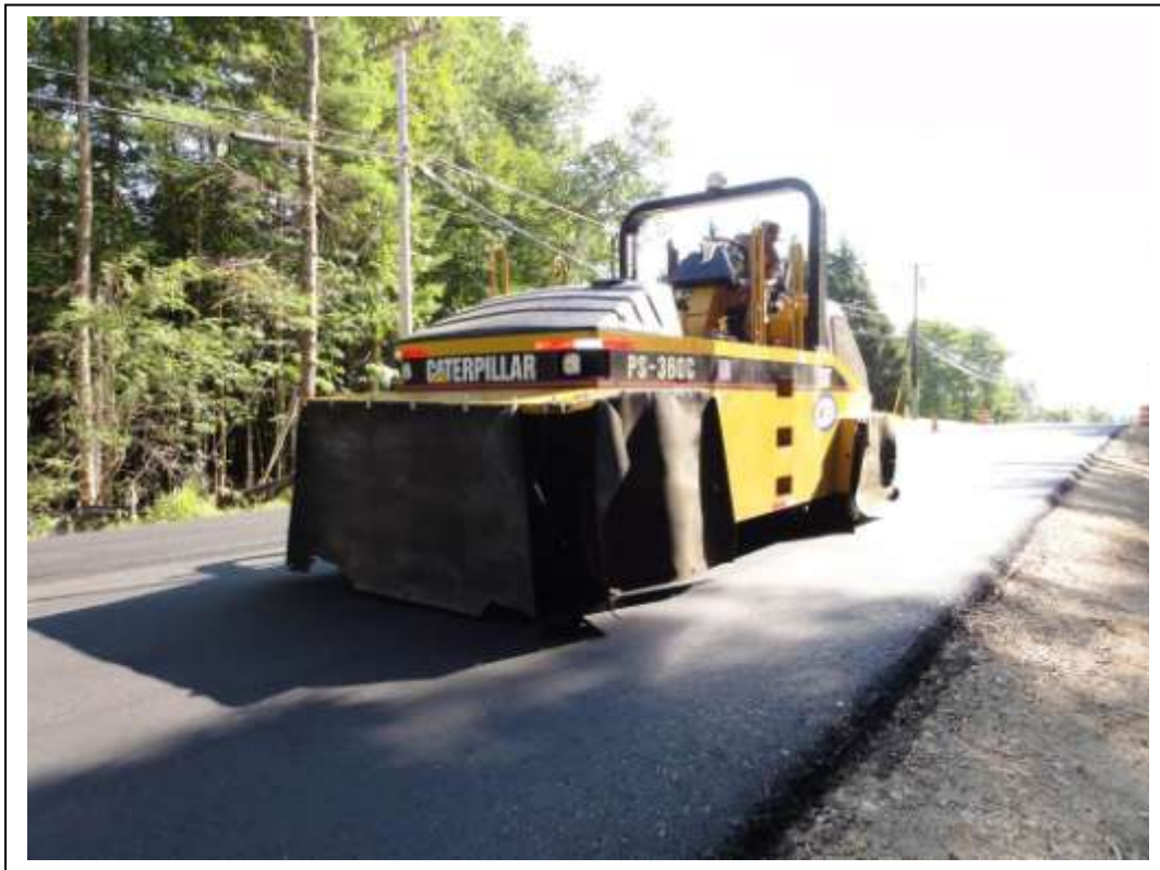
Figure 21. Rubber tire pneumatic roller used in the intermediate position.
