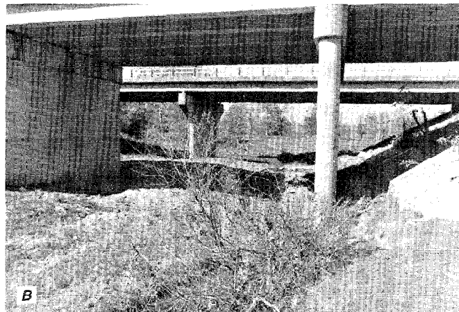
Figure 80. Feather Creek at site 31. A, View upstream in 1978, showing width of bridge waterway in relation to that of natural channel, in left foreground. B, View in 1978, showing location of low-water channel against abutment, at right, and, at left, infilling of wide channel.
