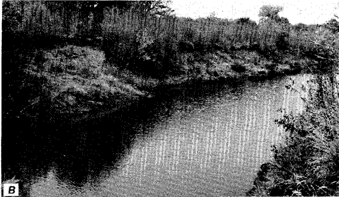
Figure 149. Big Blue River at site 71. A, Downstream junction of relocated channel (foreground) with natural channel, in 1979. B, Bank slumping along relocated channel upstream from bridge, in 1979. C, Natural channel along short segment between relocations, in 1979.
