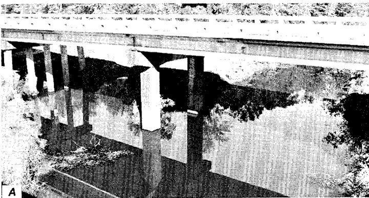
Figure 133. Oakahatta Creek at site 61. A, Channel widening at west-bound interstate bridge, as photographed in 1979. B, Relocated channel downstream from interstate bridges, in 1979.
