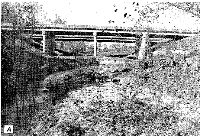
Figure 80. Feather Creek at site 31. A, View upstream in 1978, showing width of bridge waterway in relation to that of natural channel, in left foreground. B, View in 1978, showing location of low-water channel against abutment, at right, and, at left, infilling of wide channel.
