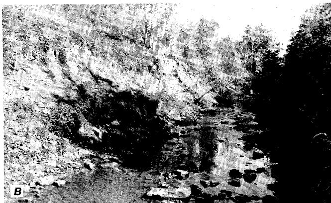
Figure 196. Five Mile Run at site 97. A, View upstream along relocated channel in vicinity of sta. 770. B, Unstable bank along relocated channel in vicinity of sta. 795. C, Natural channel just downstream from sta. 770.
