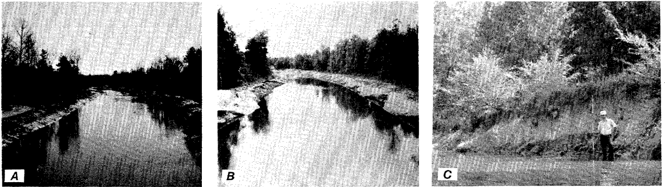
Figure 20. Calebee Creek at site 2. A, Relocated channel as viewed upstream from interstate bridge, on January 19, 1964. B, View from same point as in A, on April 22, 1964. C, Bank erosion at section 2, on August 28, 1978.
