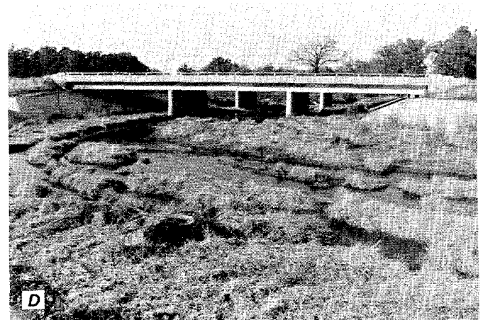
Figure 71. Stevens Creek at site 26. A, Natural channel in 1978, about 125 m downstream from relocated channel. B, Check dam, built after 1974 flood, upstream from I-72 bridge. Natural channel in background. C, View of relocated channel looking downstream from I-72 bridge, in 1978. D, View of relocated channel looking upstream toward I-72 bridge, in 1978.
