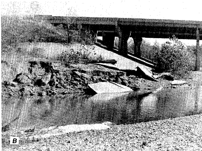
Figure 75. Eagle Creek at site 28. A, Airphoto of channel relocation, in 1972. (From Indiana Dept. of Transportation). B, Eroded concrete slope pavement at left bank upstream from bridge, in 1978. C, Eroded left bank at downstream bend in relocated channel, in 1978.
