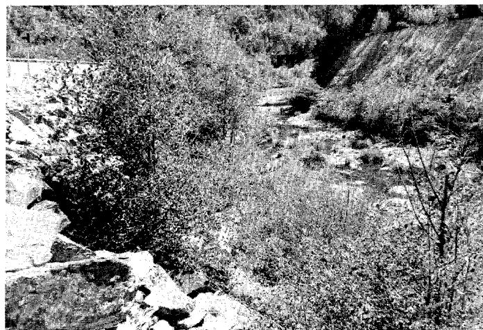
Figure 51. View upstream along relocated channel of Outlet Creek, in 1978.
