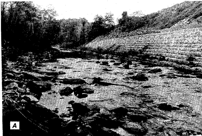
Figure 182. Pocono Creek at site 90. A, View upstream toward gabions on left bank, in 1978. B, View of natural channel downstream from relocation, in 1978.
