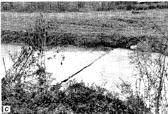
Figure 88. Beargrass Creek at site 36. A, Aerial photograph, taken in 1971, showing channel relocation. Prior channel is shown in dotted line, relocated channel in dashed line. (From U.S. Geological Survey) B, Relocated channel looking downstream from bridge at Grinstead Drive. C, Relocated channel at concrete check dam. D, Relocated channel, looking upstream from bridge at Grinstead Drive.
