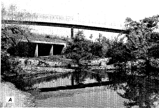
Figure 105. Moores Run at site 46. A, View upstream of stilling basin downstream from culvert. B, Apparent undercutting of gabion at toe of side slope, on stilling pool downstream from twin bridges. Note rock-and-wire mattress in background.
