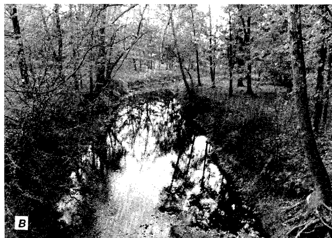
Figure 188. Black Creek at site 93. A, View downstream toward failed left bridge abutment in 1978. B, View from bridge, downstream along relocated channel, in 1978.
