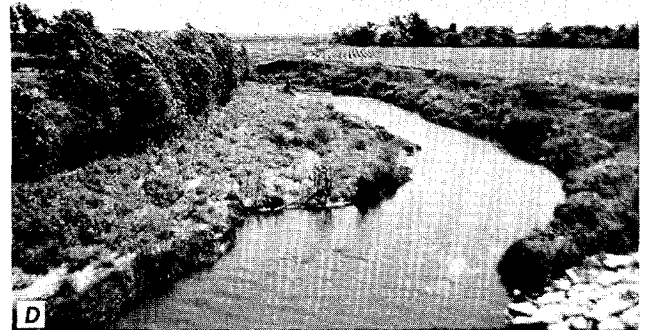
Figure 119. Kanaranzi Creek at site 54. A, Airphoto of site in 1954, before relocation. Solid line indicates position of relocated channel. (From U.S. Dept. of Agriculture) B, Relocated channel upstream from SR-91 bridge, in 1979. C, Relocated channel downstream from check dam, in 1979. D, Downstream intersection of prior channel, foreground, with relocated channel, right background.
