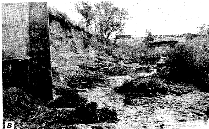
Figure 147. Middle Creek at site 70. A, Airphoto of site in 1955, position of relocated channel shown in dashed line. (From U.S. Dept. of Agriculture) B, View upstream along relocated channel from beneath bridge, in 1979. Top of exposed pier footing is at left. C, Bank erosion at bend upstream from relocated channel, in 1979. Bank height is 7.5 m.
