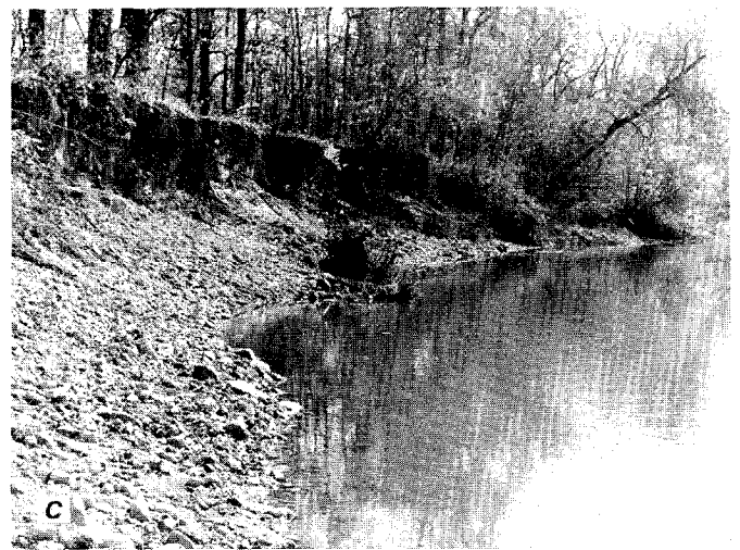
Figure 75. Eagle Creek at site 28. A, Airphoto of channel relocation, in 1972. (From Indiana Dept. of Transportation). B, Eroded concrete slope pavement at left bank upstream from bridge, in 1978. C, Eroded left bank at downstream bend in relocated channel, in 1978.
