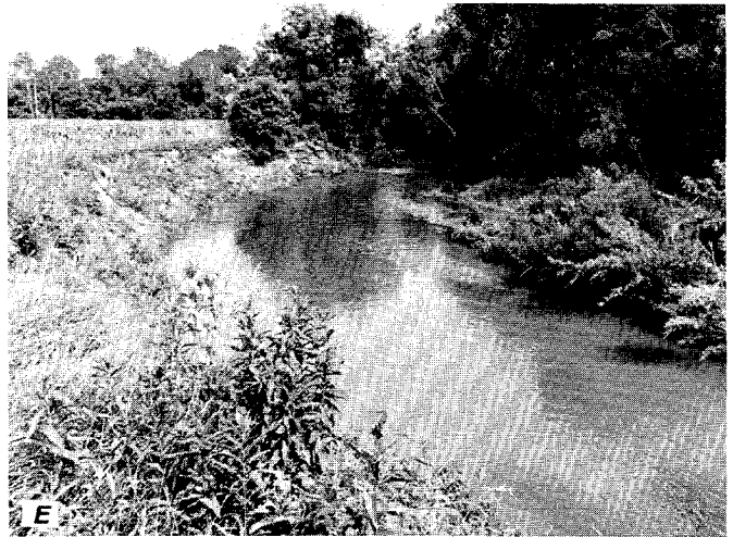
Figure 157. Raccoon Creek at site 75 and near Granville, Ohio. A, Aerial photograph of site in 1964. Approximate position of relocated channel shown in dashed line. B, Riprapped section of relocated channel, in 1979. C, Downstream junction of relocated channel with natural channel, in 1979. D, Relocated channel of Raccoon Creek near Granville, in 1979. E, Bank erosion at bend in relocated channel of Raccoon Creek near Granville, in 1979.
