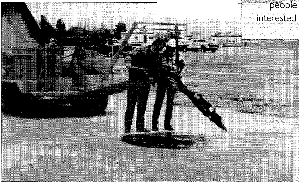
An April field demonstration held by the Lead States team for innovative pavement maintenance in Boise, Idaho, highlighted use of the velocity-fill pothole patcher.
