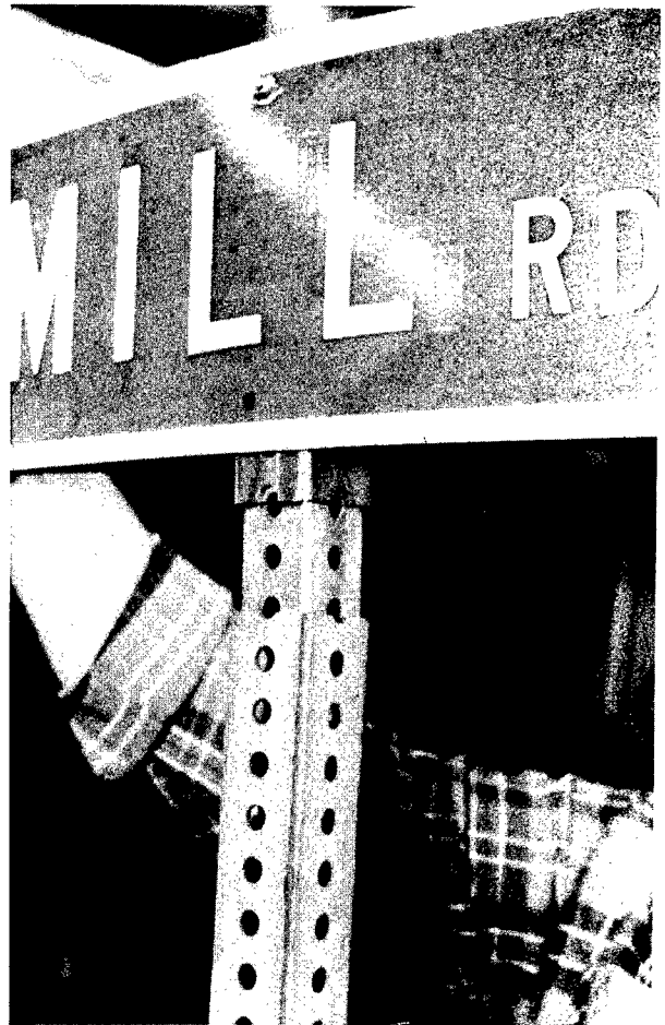
Figure 29. Back-to-back signs are shimmed down the wedge.
