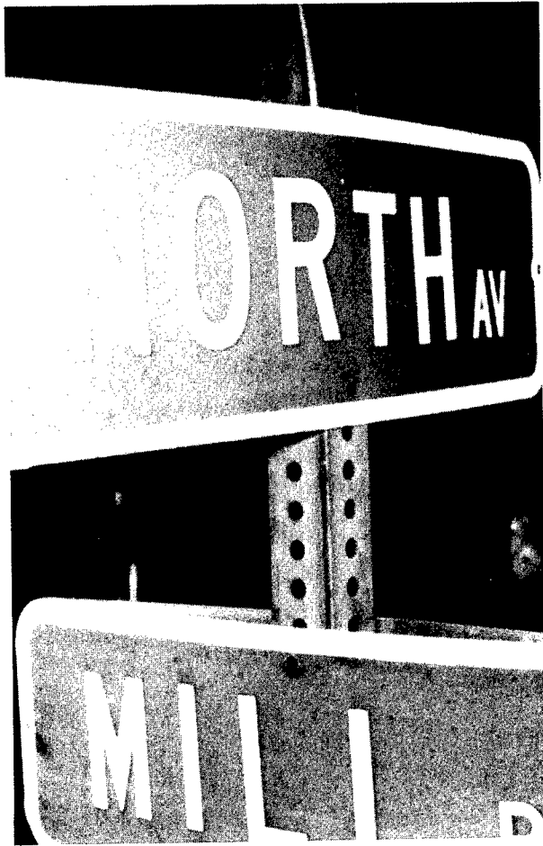
Figure 30. A second set of back-to-back signs is added to the 2-in (50.8-mm) tube.
