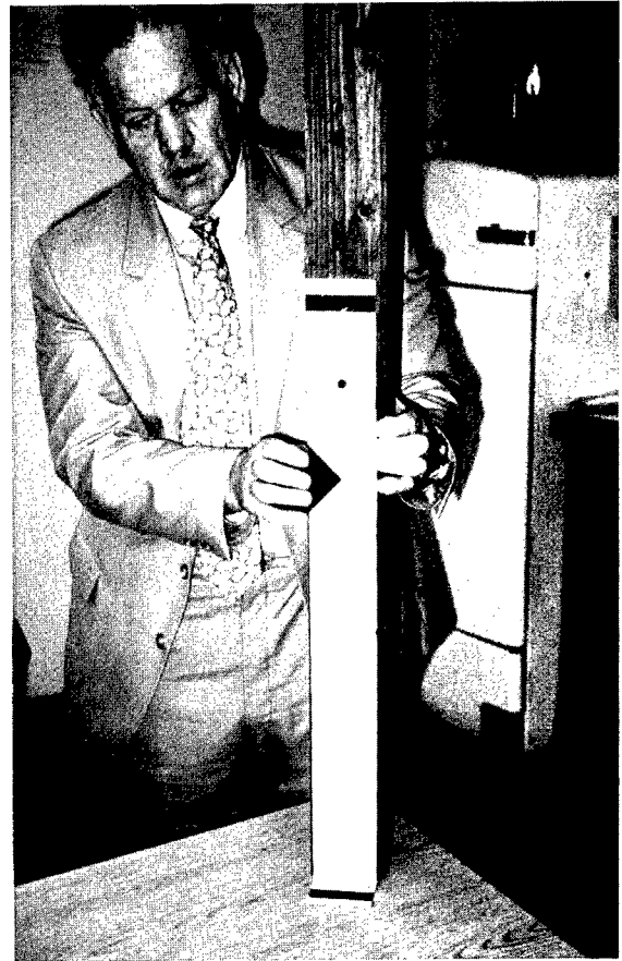
Figure 63. Cleat is attached to the backside at the bottom to the post.
