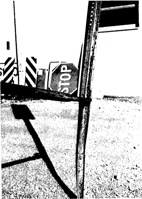
Figure 60. Tool hooks onto front of bent U-channel post.
