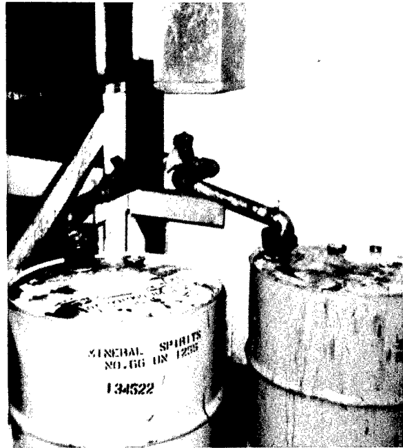
Figure 20. Silk-screen wash bay drainage system showing disposal drums.
