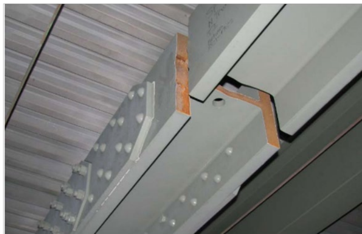
B. Close-up photo of the fractured member.
