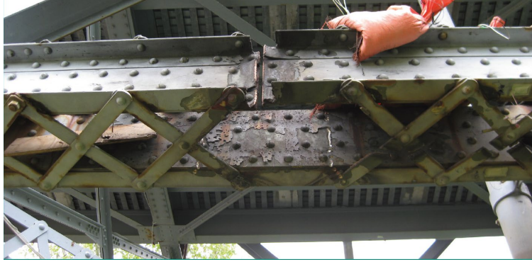
Figure 3. Photo. Blast-induced fracture of the bottom chord member in the Milton–Madison Bridge (FHWA 2013).
