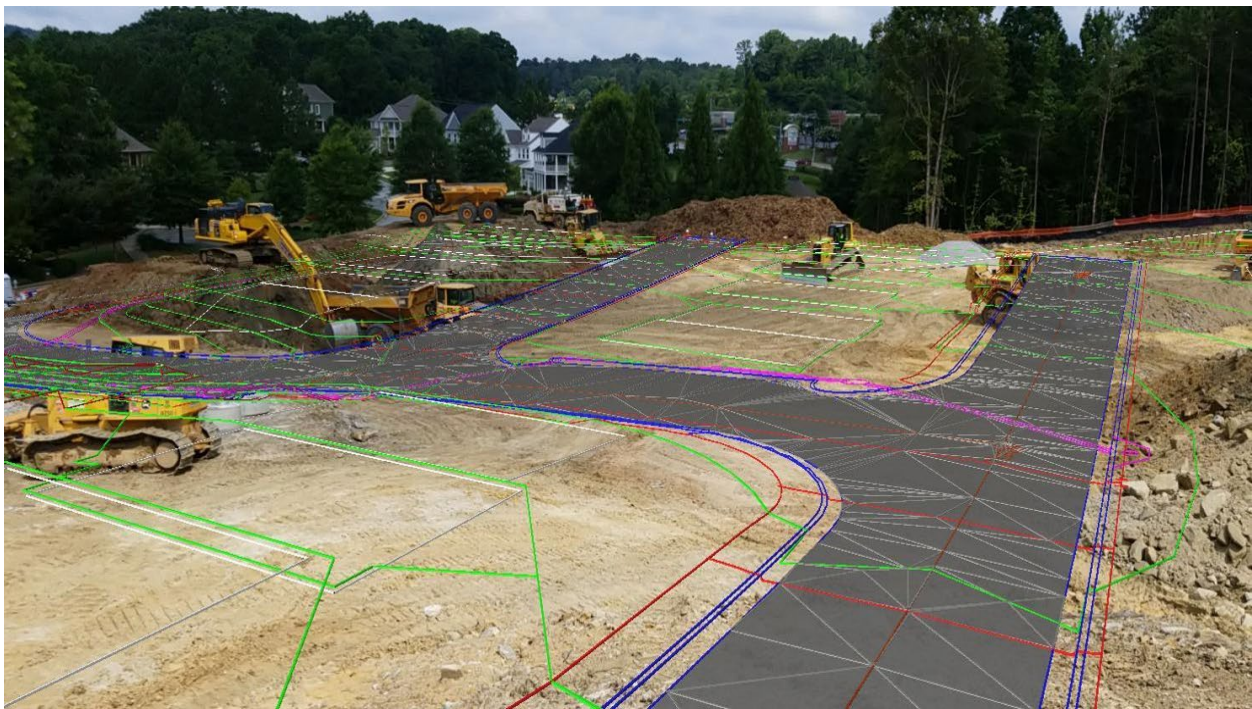
Figure 8. Graphic. Display of design data overlaid on the video display of a tablet device.
