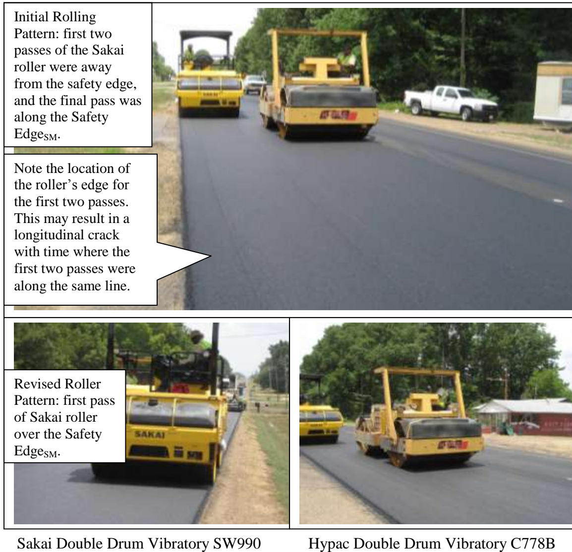
Figure 18. Two double drum vibratory steel wheel rollers were used in parallel in the breakdown position to compact the 9.5 mm HMA mix.
