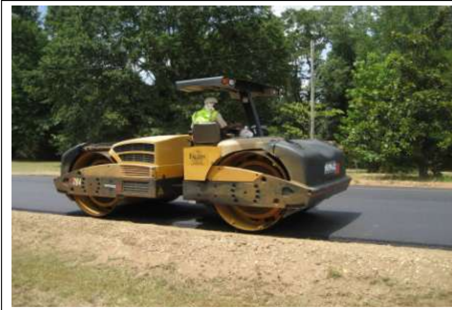
Figure 19. Rollers used in the intermediate and finish positions for compacting the 9.5 mm HMA overlay mixture.
