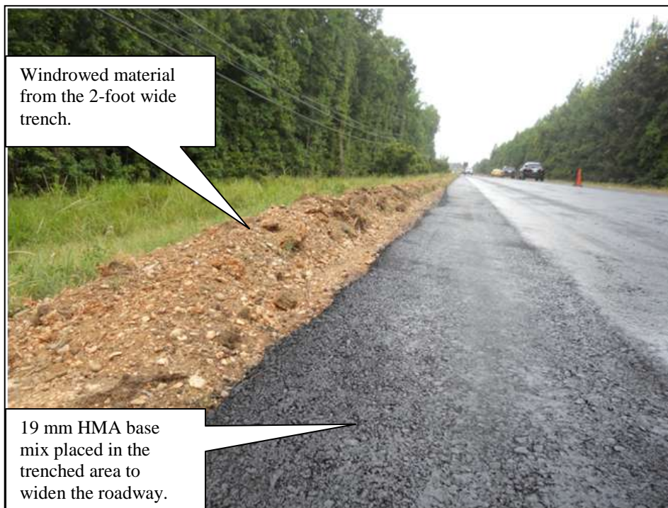
Figure 5. General view of the 19 mm HMA base placed to widen the roadway.
