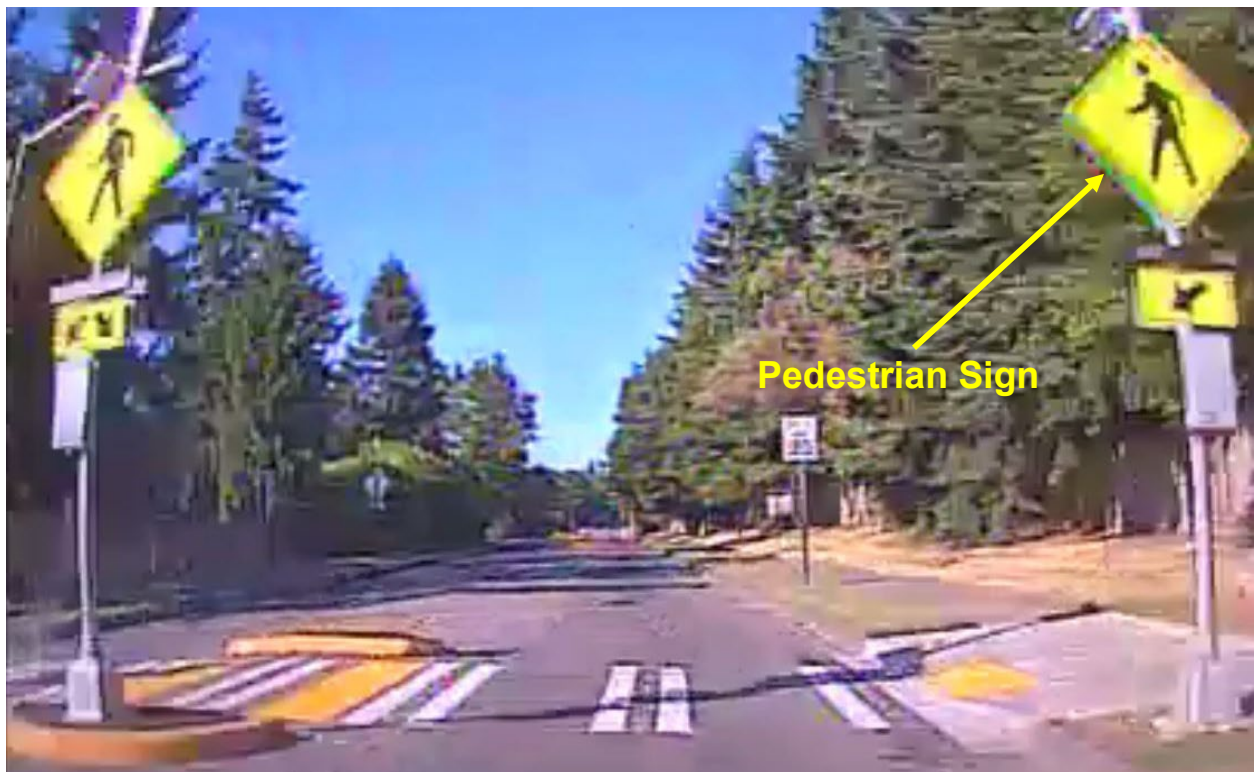
Figure 22. Illustration of HVC fully constructed in HVC site 18.
