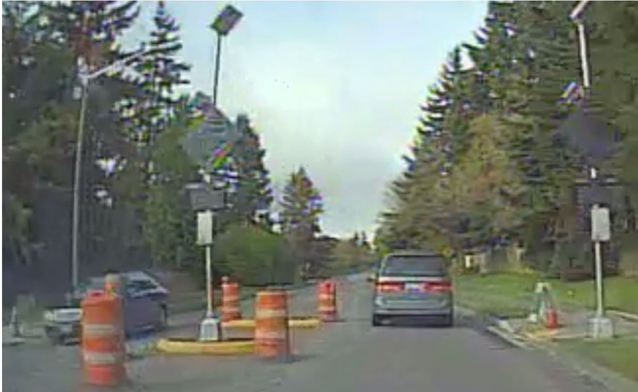
Figure 23. Illustration of HVC under-construction in HVC site 18.
