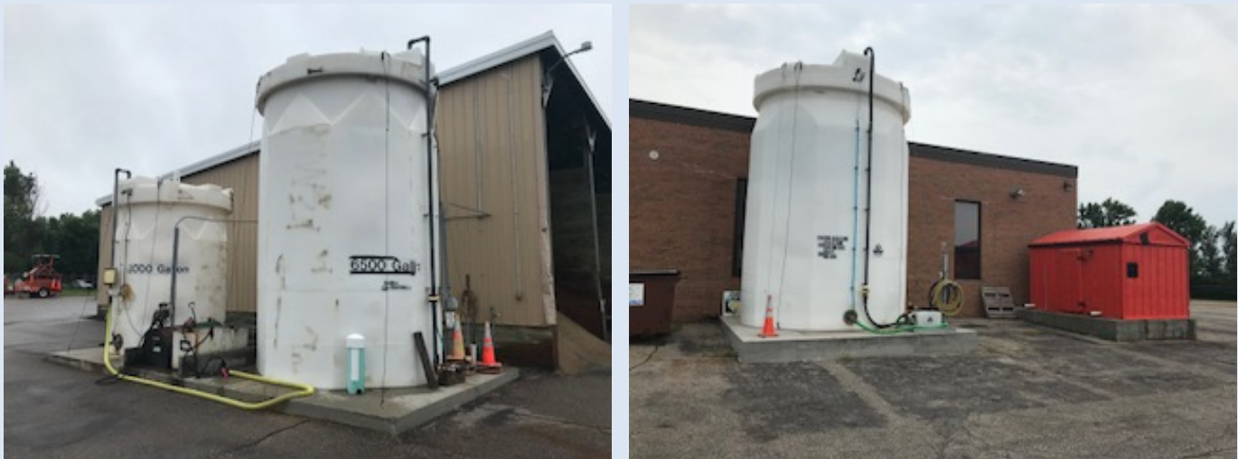
Figure 3. Liquid deicer storage tanks (3000 gal, 6500 gal, and 10,000 gal capacity) used by MnDOT, District 7. Source: C. Fester, MnDOT.
