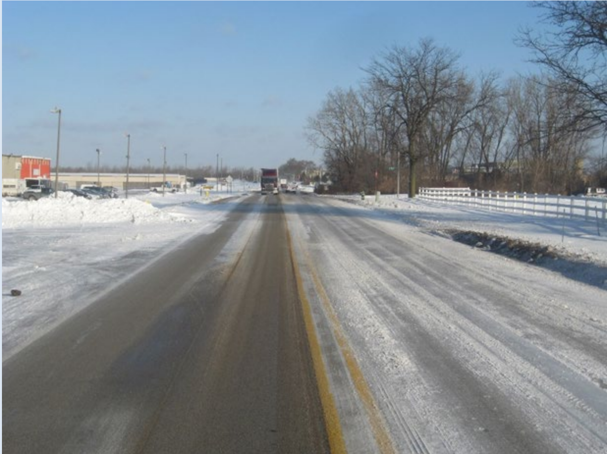
Figure 29. Image of side-by-side comparison of road condition following treatment with liquids (left) versus normal practice without liquids (right) in Dupage County, Il. Conditions were air temperature of -15°F with blowing and drifting snow. Source: Dupage County DOT
