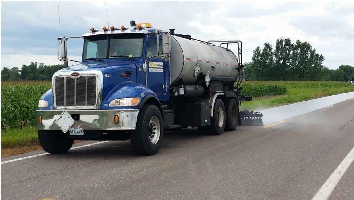
**Figure 1.1** Application of spray applied emulsions.
